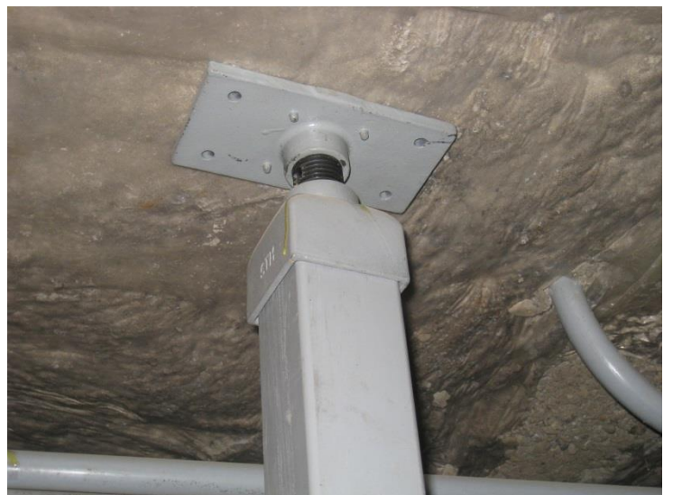
Temporary HSS support in the GSB Crawl Space
