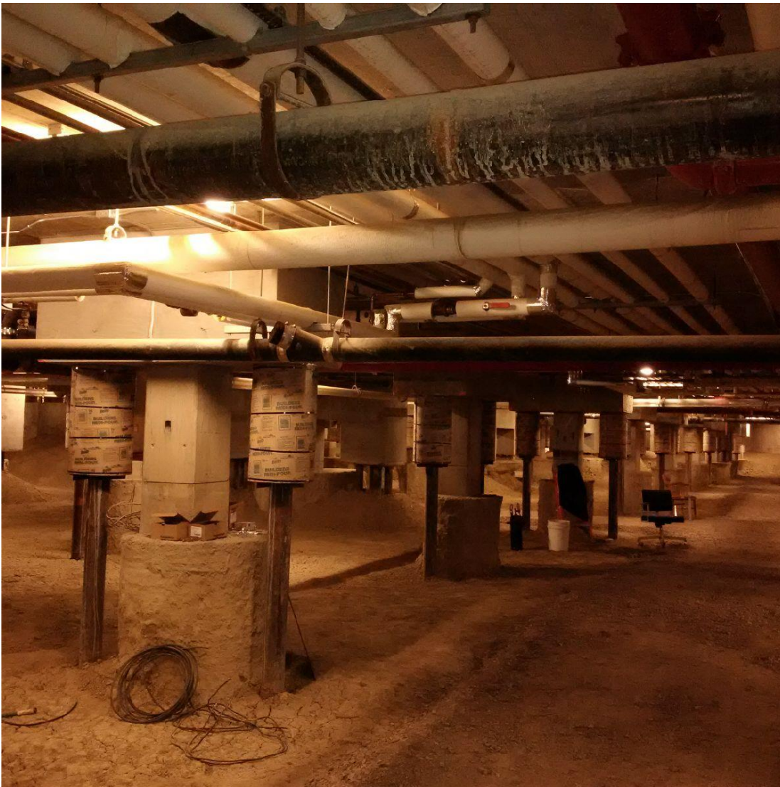
Fig 1: Lethbridge Main Lab (adjacent to the General Services Building) – a lattice system of hydraulically jacked up pipes (each pair of piles was installed next to the original piles) in crawl space underneath ground floor
