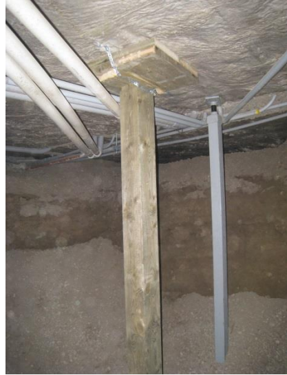
Temporary timber support in crawl space
