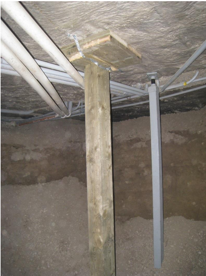
Fig 4: Lethbridge General Services Building (temporary wooded support underneath the office area)
