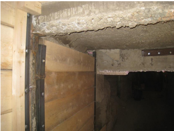
Temporary Shoring in the Crawl Space
