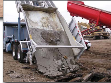
Figure 15. Delivering hardened concrete to a recycler
