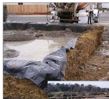
Figure 9. Hay bale and plastic washout pit
