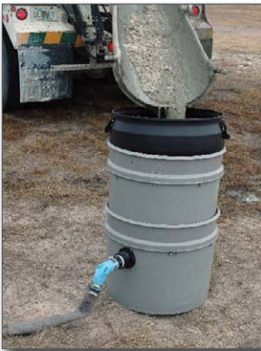
Figure 3. Concrete washout filter
