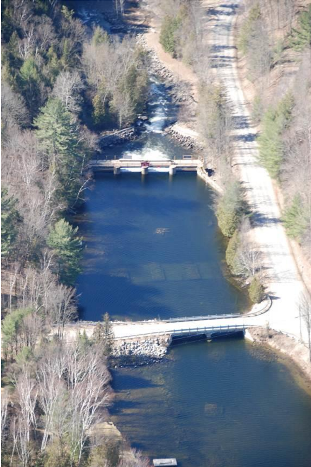
1 Airplane view of the dam looking downstream/south. Remnants of the old timber dam are in the foreground.
