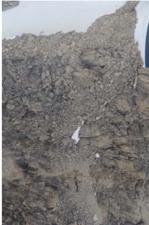
Photo 11: Slide path 3 – fractured and loose surficial material at crest
