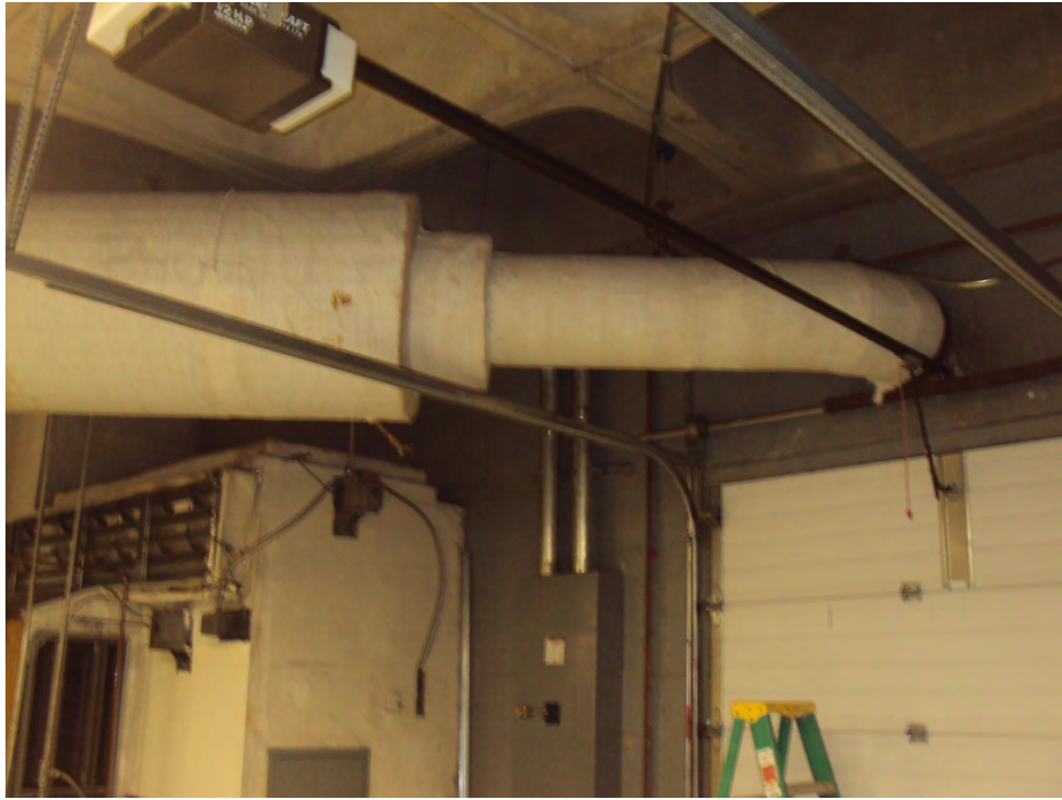
Photo 39: Hot air duct in Building H7 (Substation). Both the weaved, fabric wrap and the underlying paring insulation were sampled in 2012 and found to be asbestos containing. The wrap contains 90% chrysotile asbestos and the insulation contains 3% chrysotile asbestos. (Photo taken during 2012 assessment)
