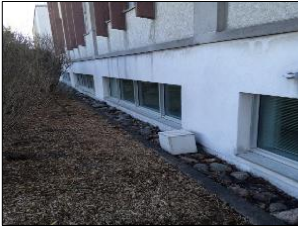
Photo 32 – Non-asbestos white exterior stucco on the north elevation
