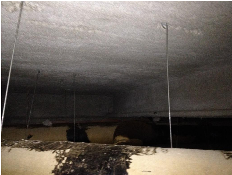
Photo 4: Spray-applied fireproofing was observed on the ceiling deck and structural beams throughout the ground floor south wing. Overspray and debris were also observed throughout.
