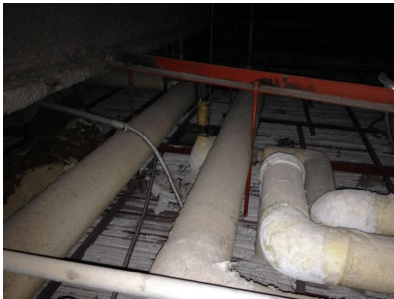
Photo 1: Pipe runs insulated with asbestos-containing Sweatwrap and parged fittings were observed in a pipe chase, accessible via a wall hatch in office G-002.
