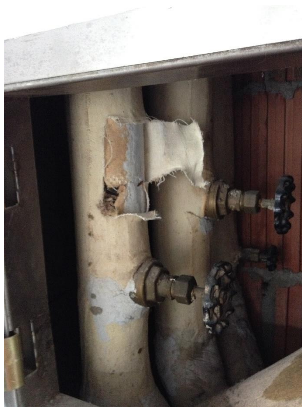
Photo 1: Pipe runs insulated with asbestos-containing Sweatwrap and parged fittings were observed in a pipe chase, accessible via a wall hatch in office G-002.
