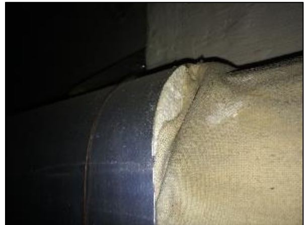
Photo 11 – Non-asbestos styrofoam insulation on pipe straight.
