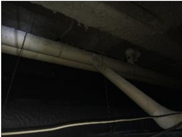
Photo 8 – Friable asbestos containing aircell and sweat wrap insulation on pipe straights
