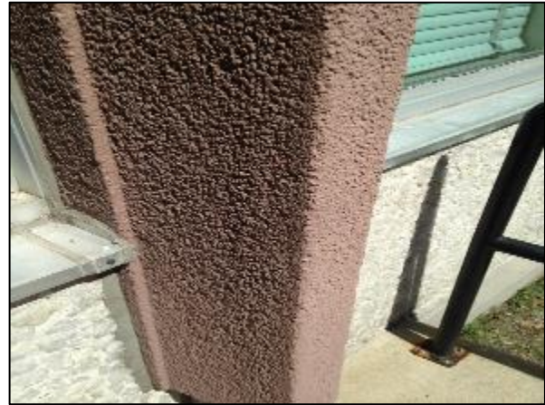
Photo 33 – Non-asbestos red exterior arch detail on the south elevation
