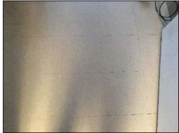
Photo 23 – Non-asbestos 12"x12" vinyl floor tile, beige with beige streaks
