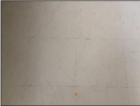
Photo 22 – Non-asbestos 12"x12" vinyl floor tile, beige with dark streaks
