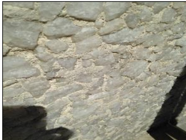
Photo 34 – Non-asbestos exterior plaster with stone inclusions
