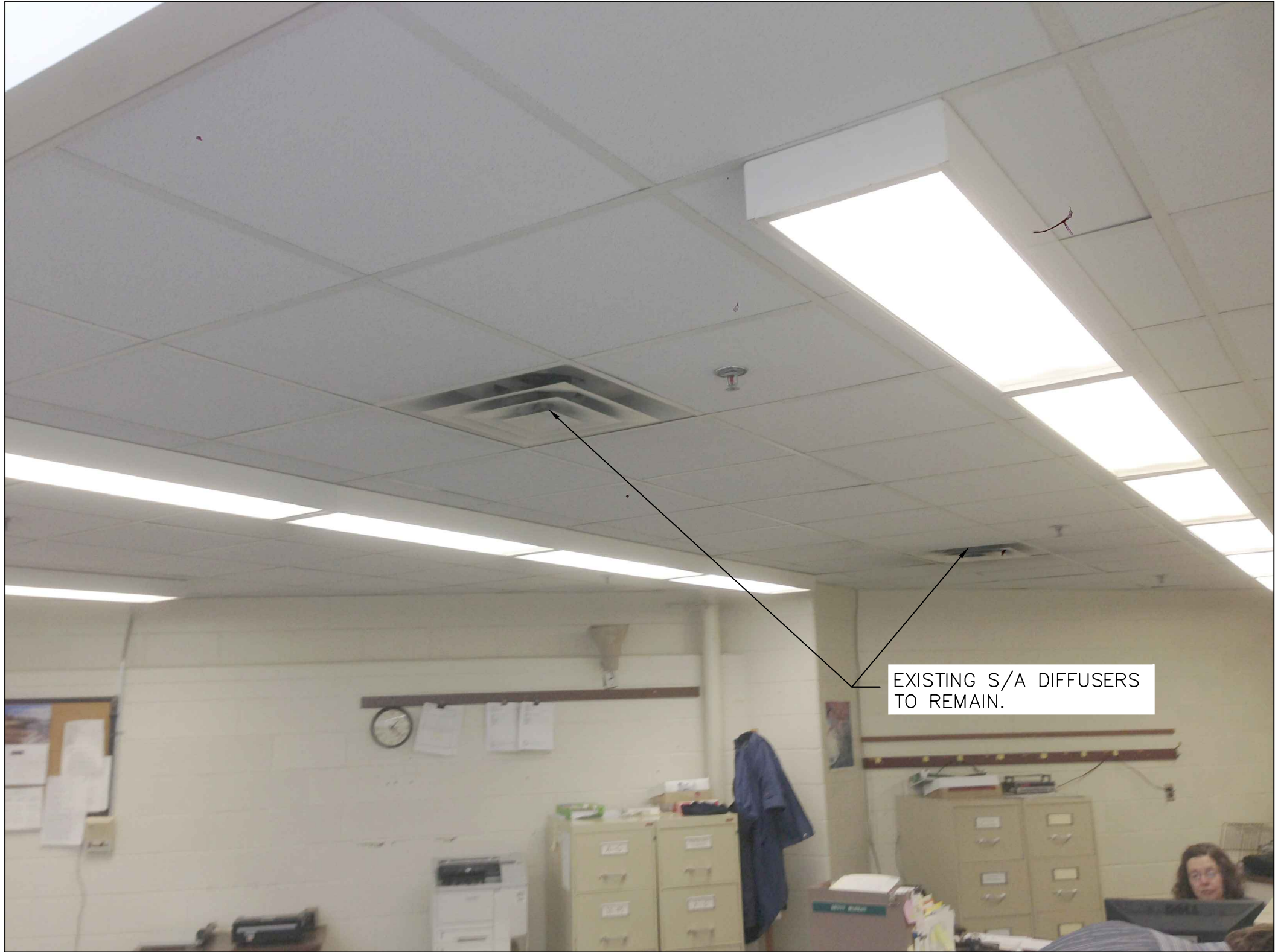
3 EXISTING S/A GRILLES SHALL BE REMOVED M-801/ NTS
