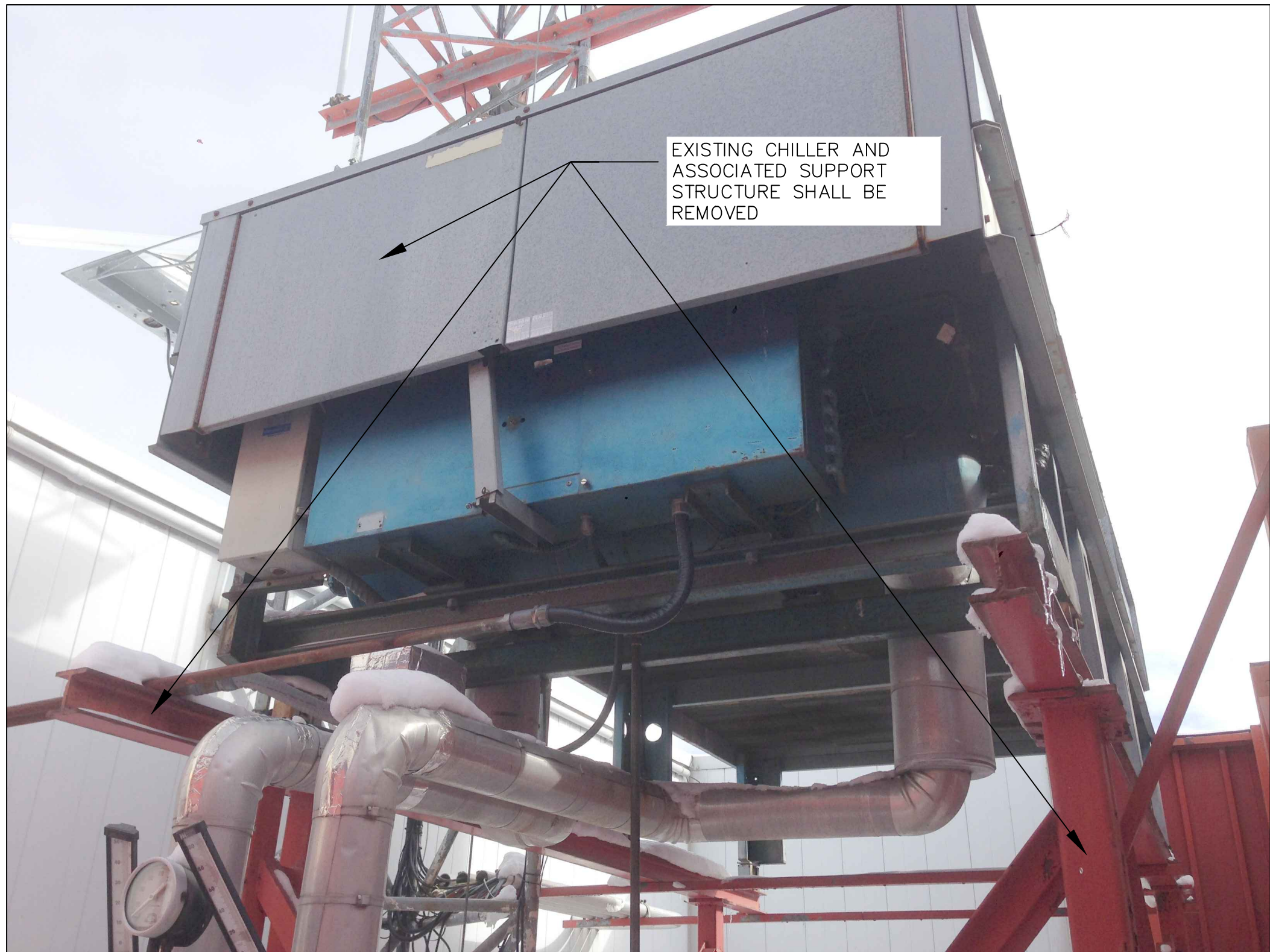
1 EXISTING CHILLER AND STRUCTURAL SUPPORT SHALL BE REMOVED M-802 NTS
