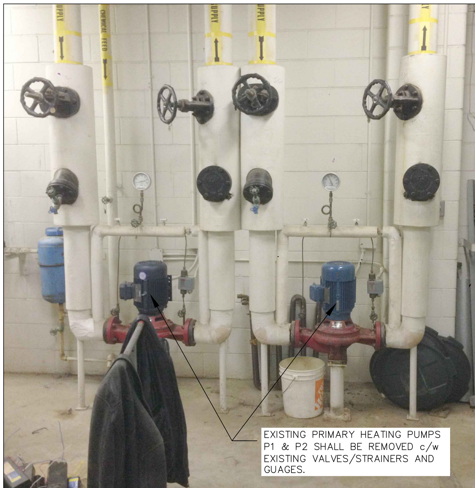
7 EXISTING HEATING PUMPS SHALL BE REMOVED M-801/ NTS
