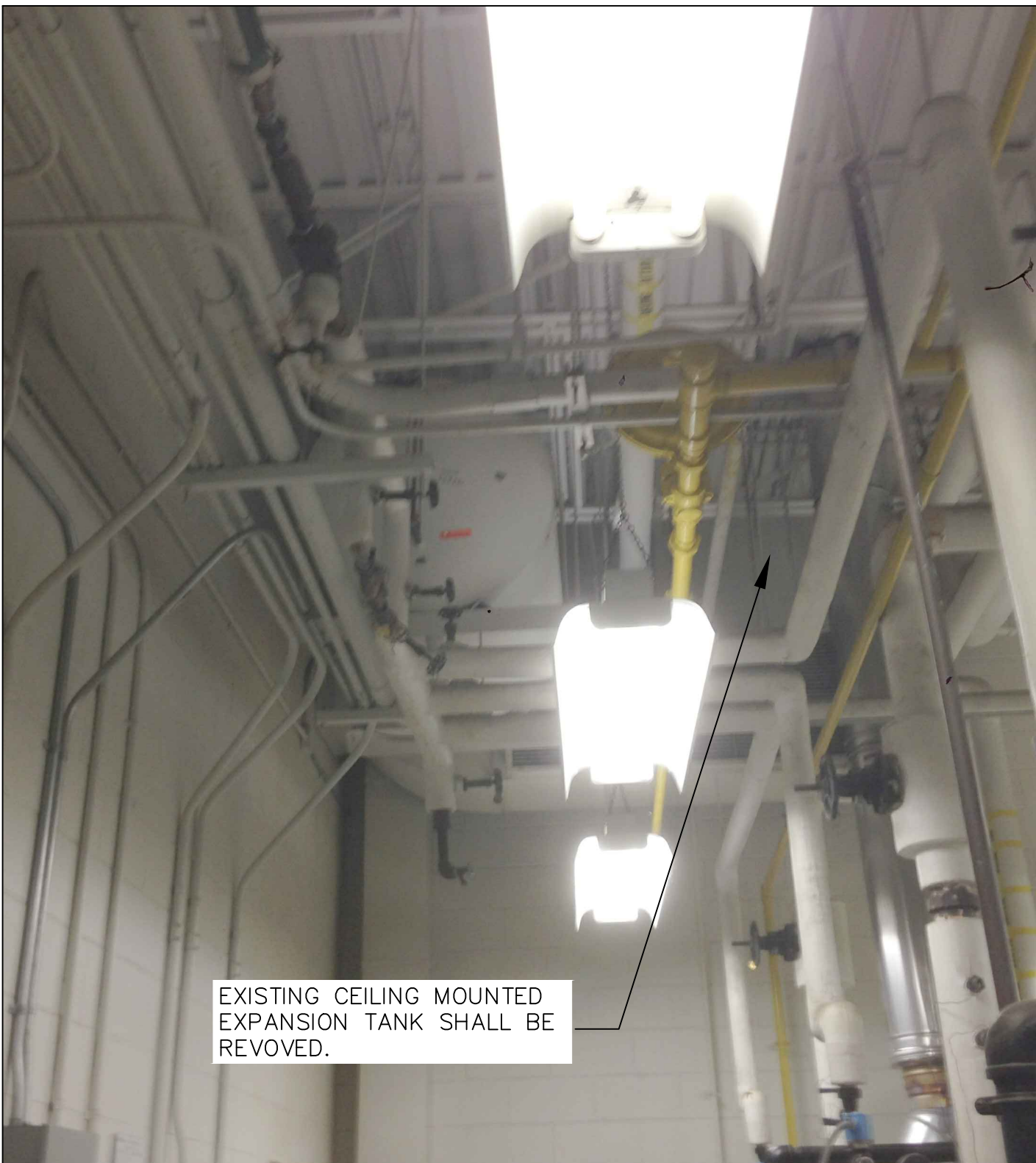
5 EXISTING CEILING MOUNTED EXPANSION TANK SHALL BE REMOVED M-801/ NTS
