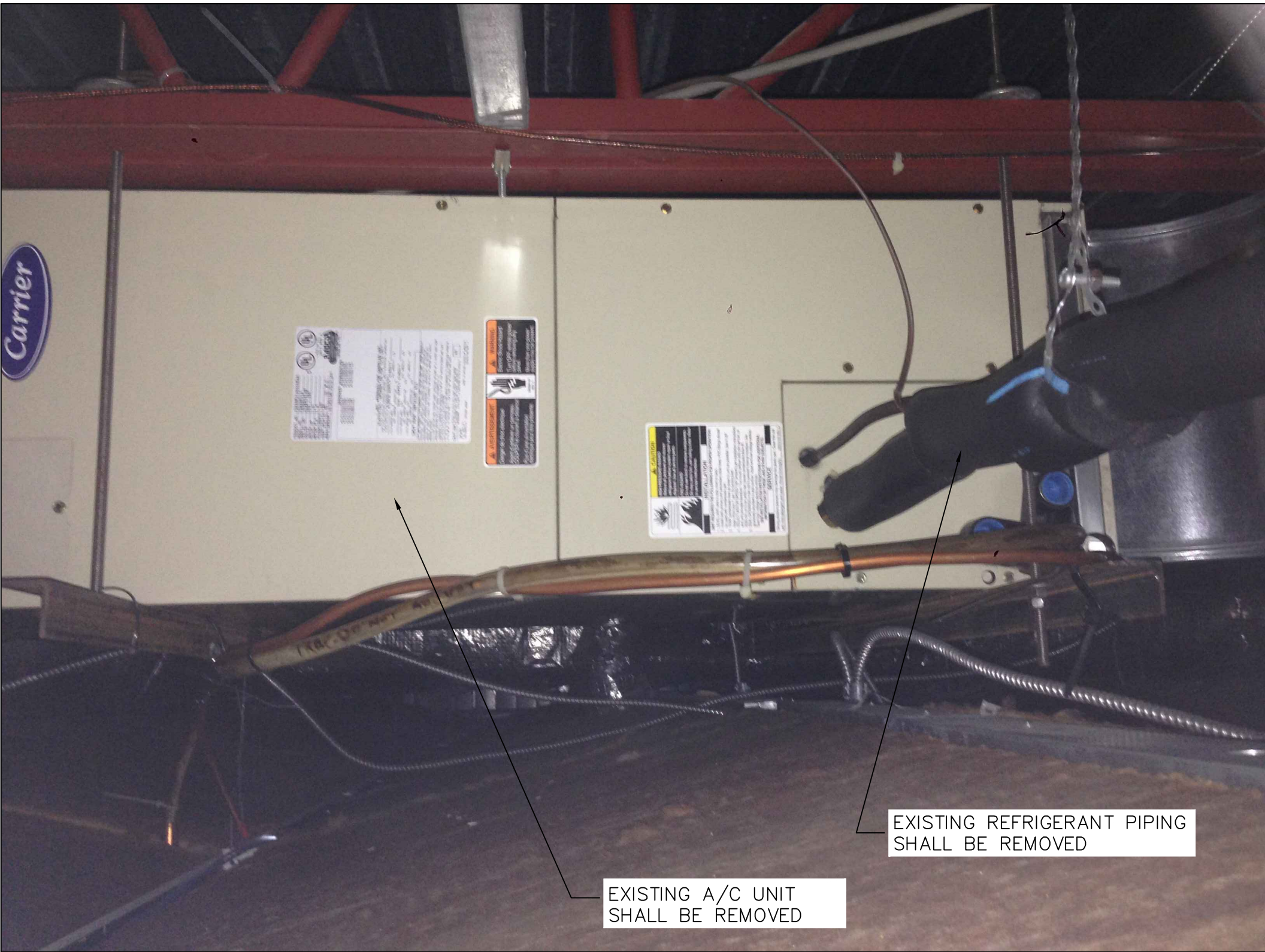
9 EXISTING A/C UNIT SHALL BE REMOVED M-801/ NTS
