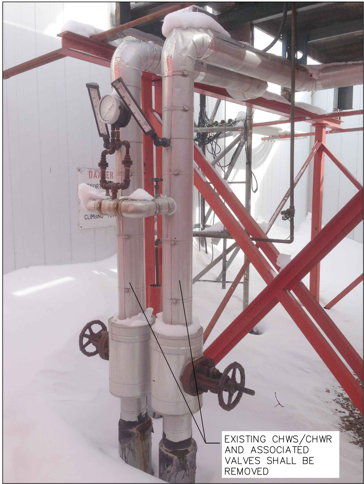
10 EXISTING CHWS/CHWR SHALL BE REMOVED M-801/ NTS
