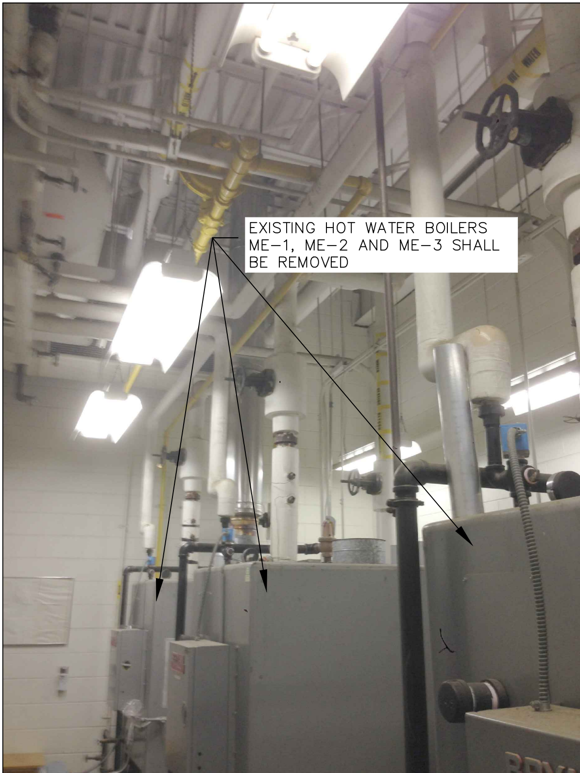
8 EXISTING HOT WATER BOILERS SHALL BE REMOVED M-801/ NTS
