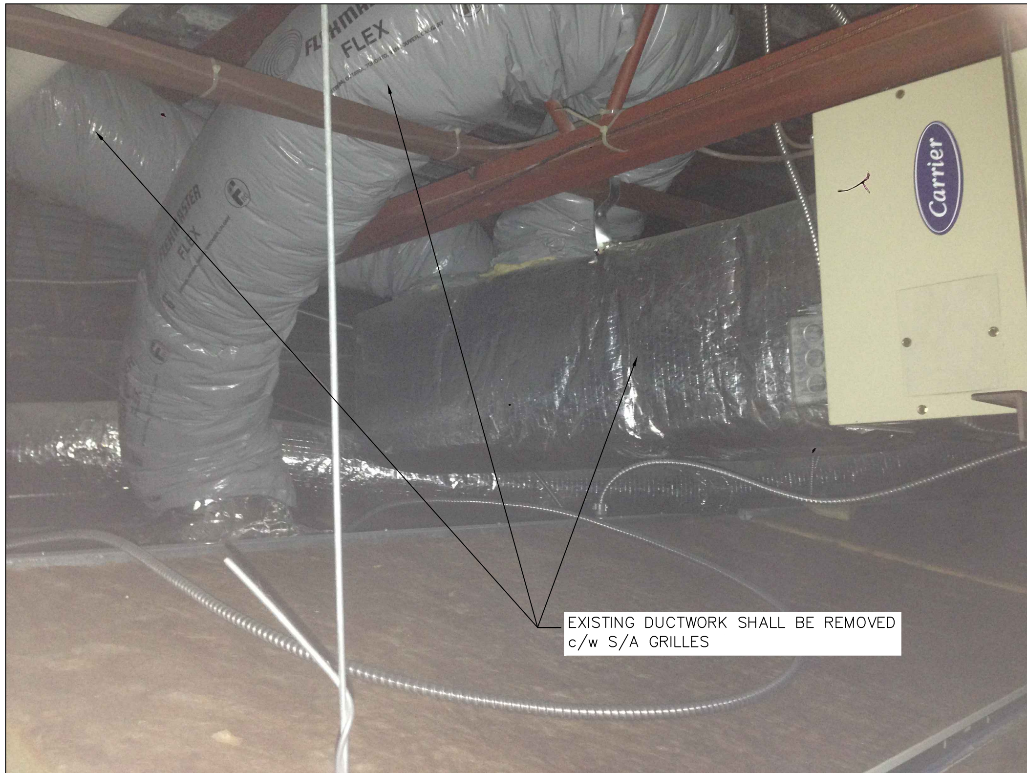
4 EXISTING DUCTWORK SHALL BE REMOVED M-801/ NTS
