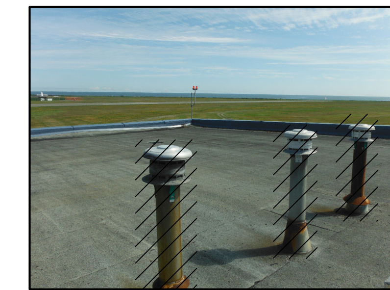
FIGURE 12: EXISTING BOILER VENTS TO BE DEMOLISHED -ROOF.
