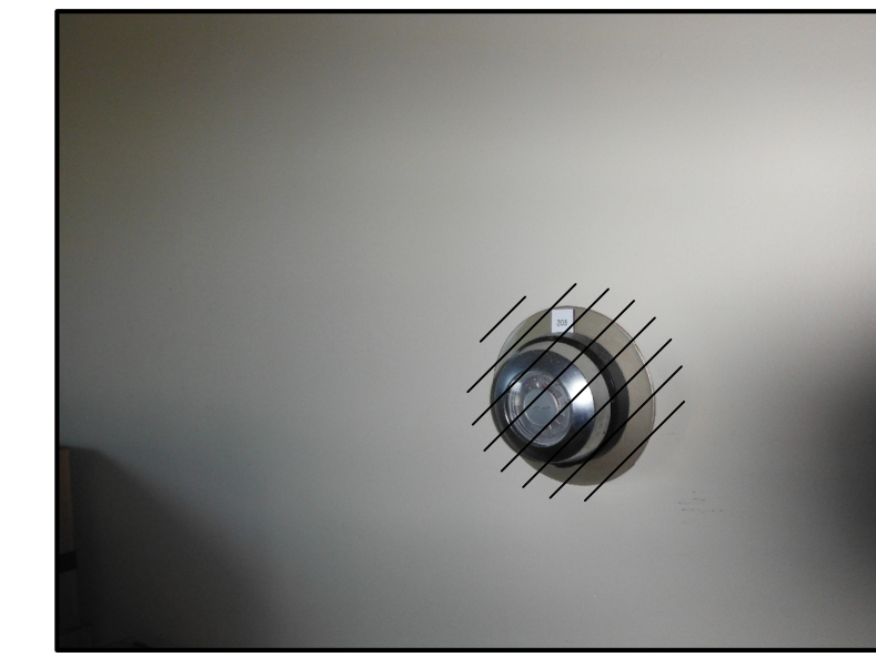
FIGURE 1: EXISTING THERMOSTAT UNIT DEMOLITION - OFFICE 123. TYPICAL OF 9.
