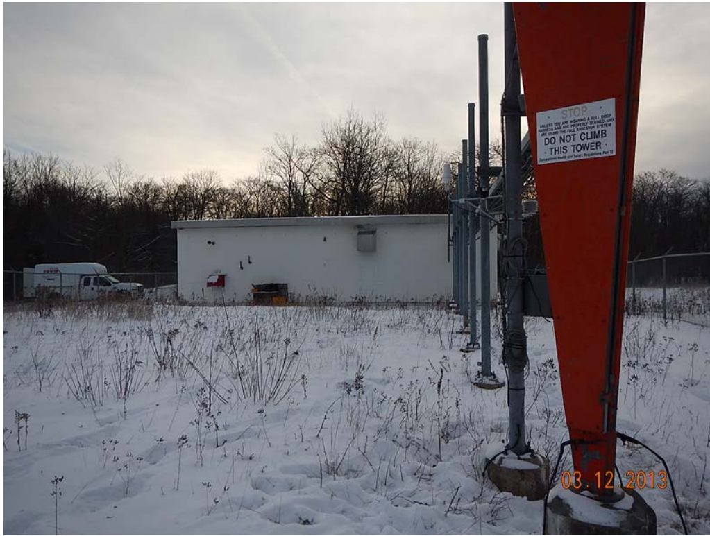
Figure 3: Existing Waveguide Bridge
