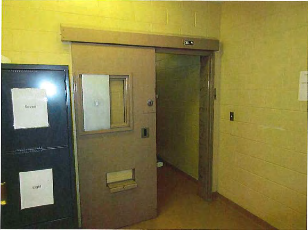
Photo 5 - Typical Cell Door
