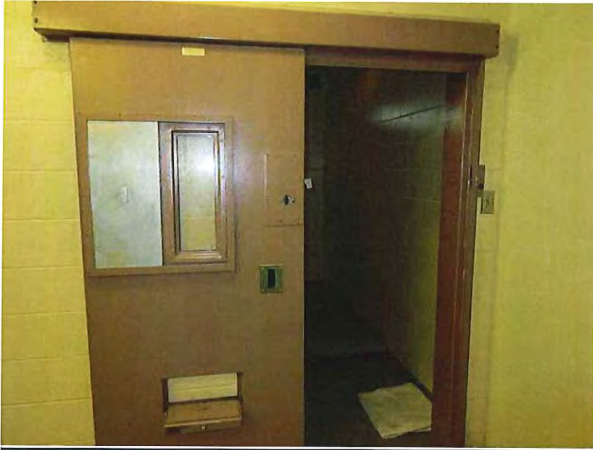
Photo 9 - Typical Cell Door
