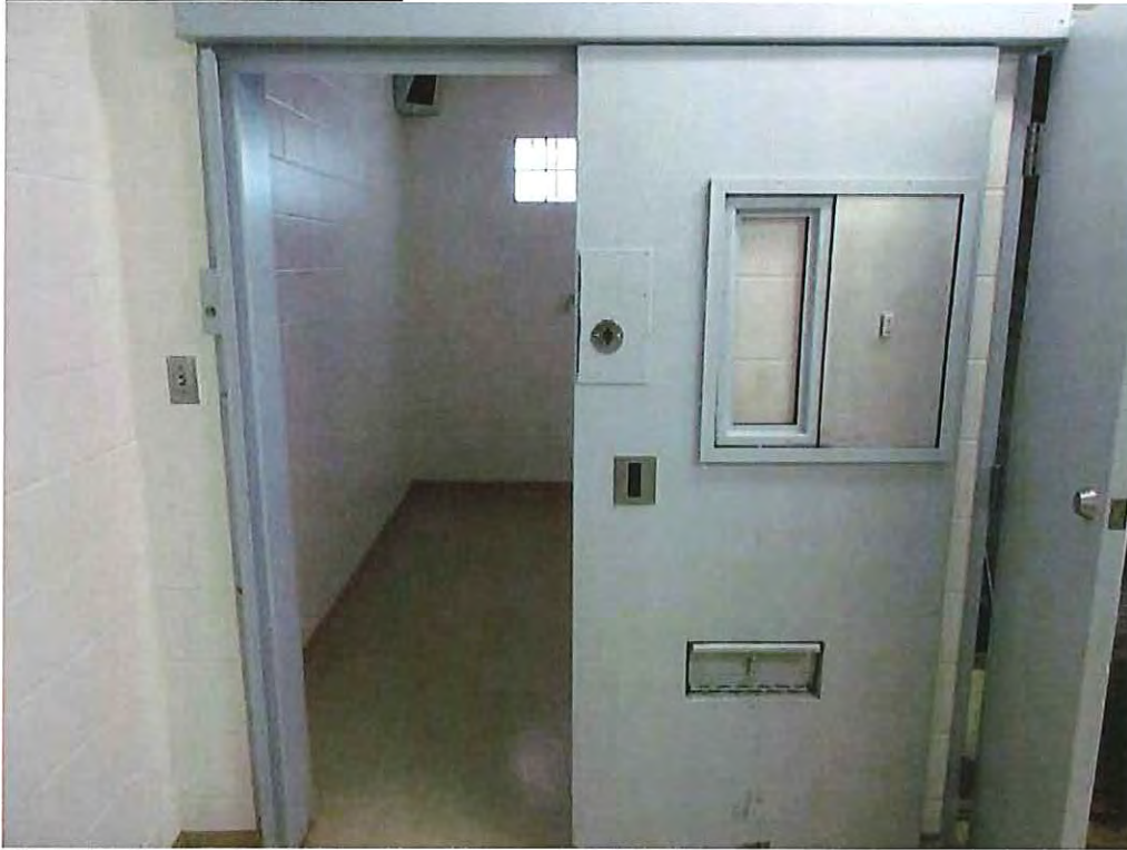
Photo 1 - Typical Cell Door
