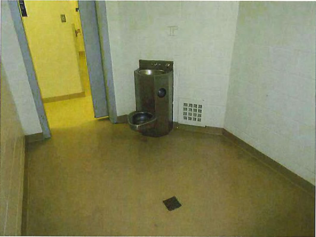
Photo 3 - Typical Detention Toilet and Floor Drain
