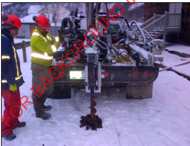
Photo 2: Drilling at BH14-01
