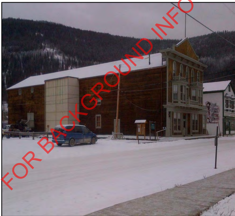
Photo 1: Front/west side of Theatre, viewing northeast
