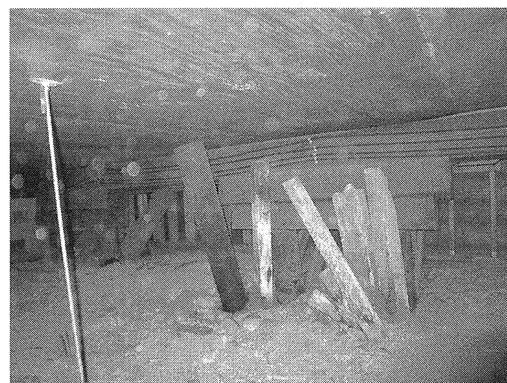
9 VIEW OF EXISTING PILE SUPPORT AT WEST SIDE OF MAIN BUILDING
