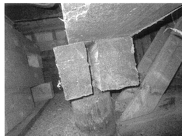
17 VIEW OF SPLIT PILE CAP AT NORTHWEST CORNER
