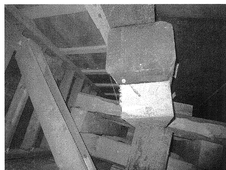
15 GENERAL VIEW OF EXISTING PILE CAP AND GROUND FLOOR BEAM THAT ARE ROTATED
