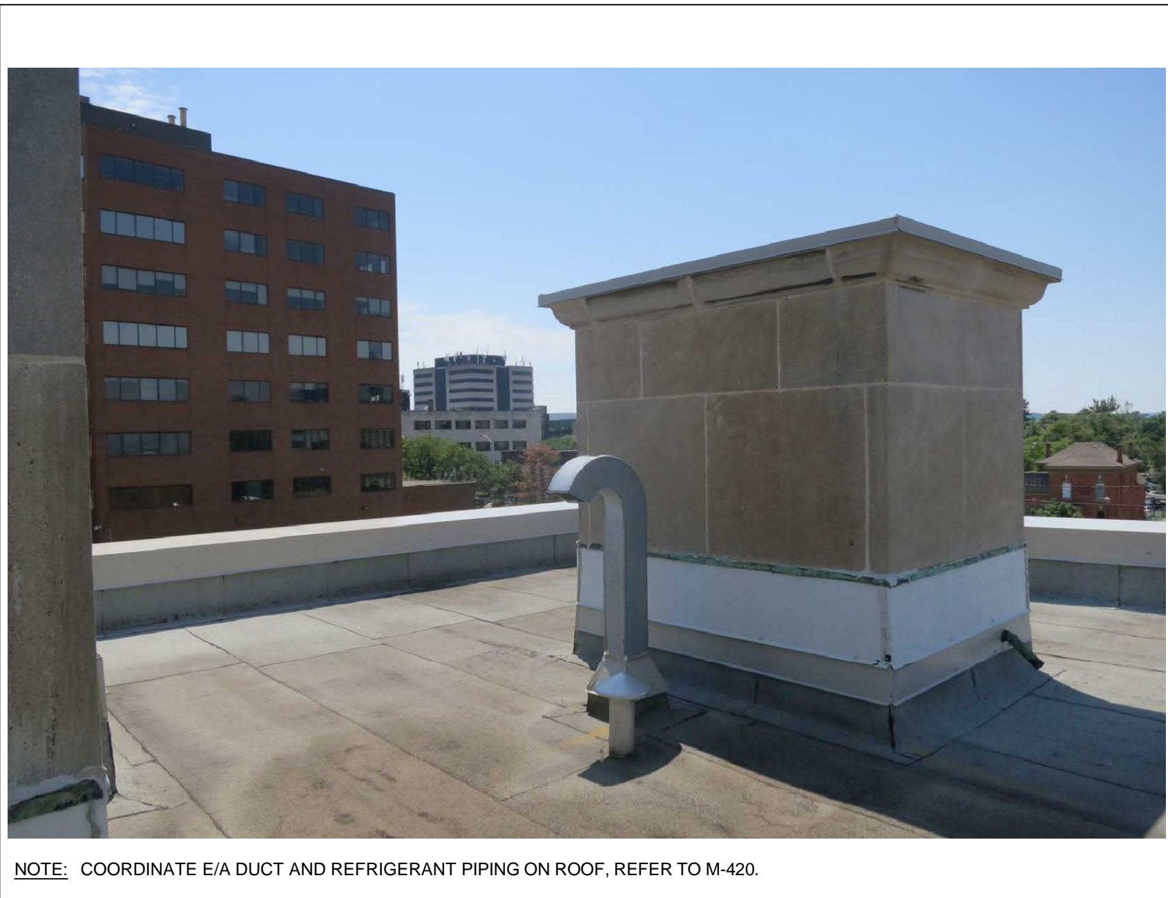
3 EXISTING ROOF ENCLOSURE AND GOOSENECK M-600 N.T.S.
