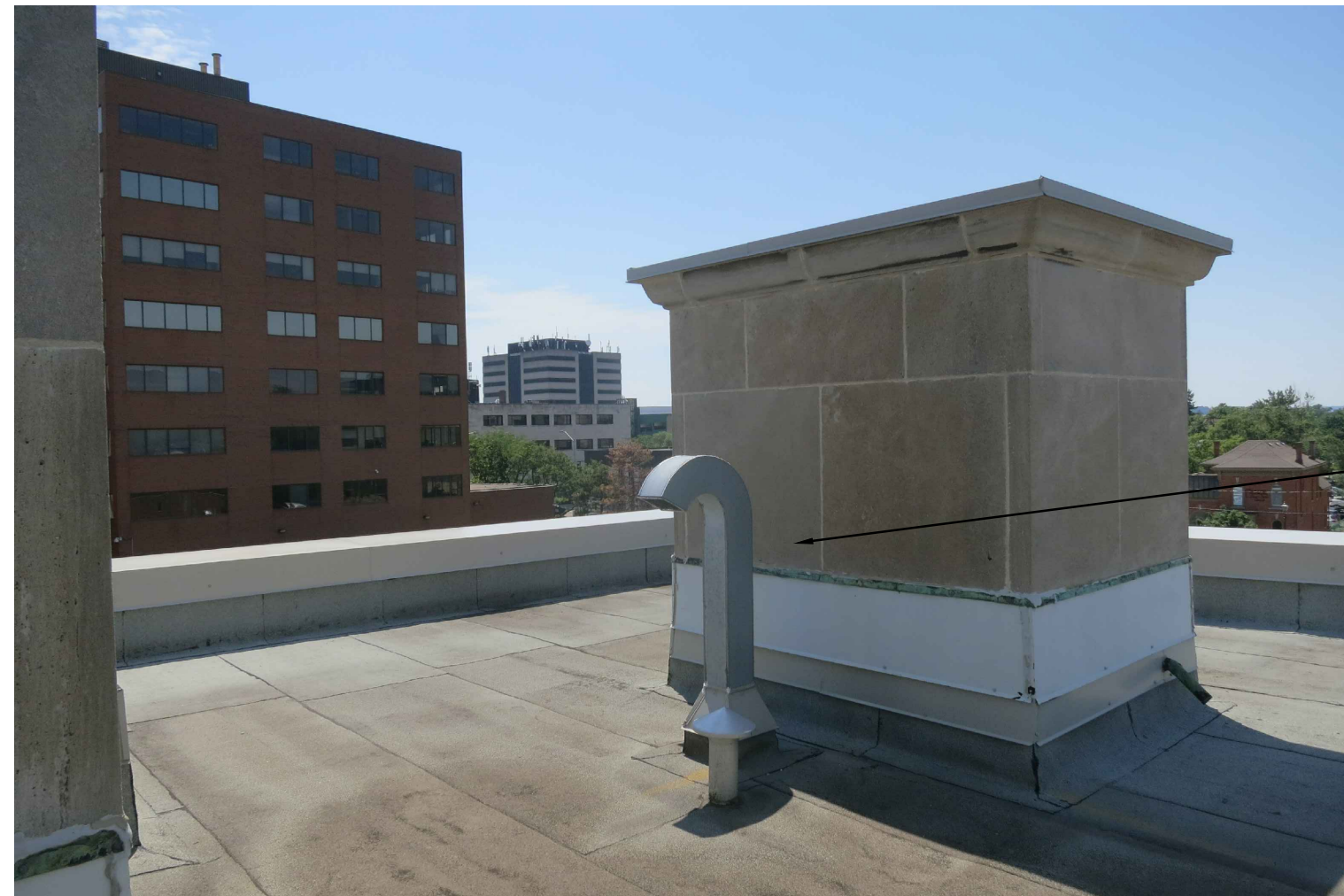
5 PHOTO OF ROOFTOP ENCLOSURE WHERE NEW MECH SERVICES TO PENETRATE 1:50
