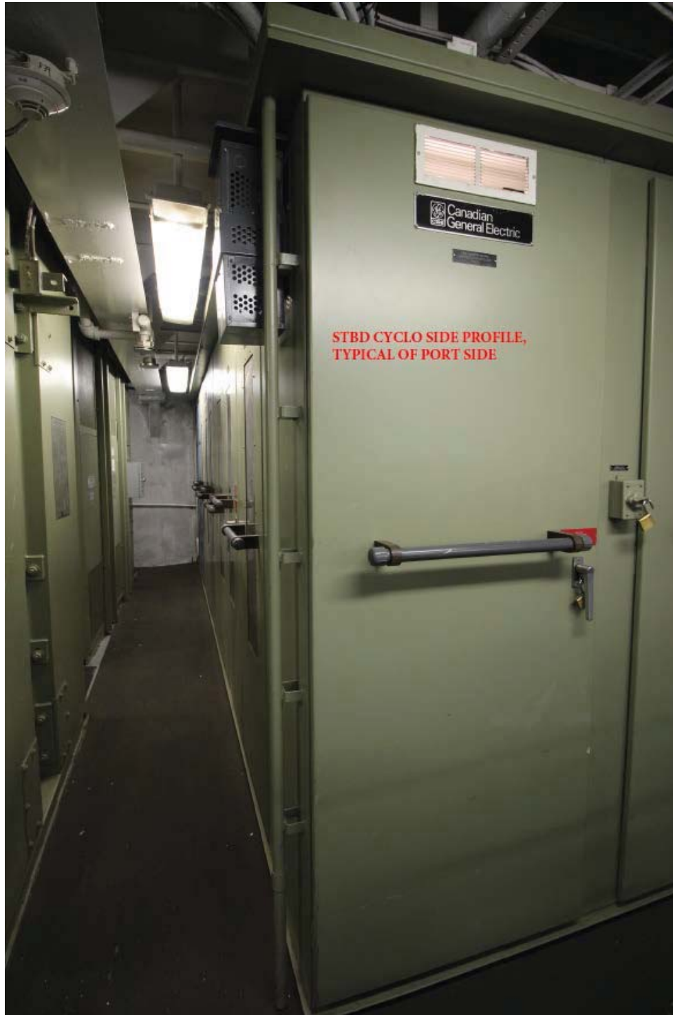
10.5 Figure 5 Cycloconverter side profile
