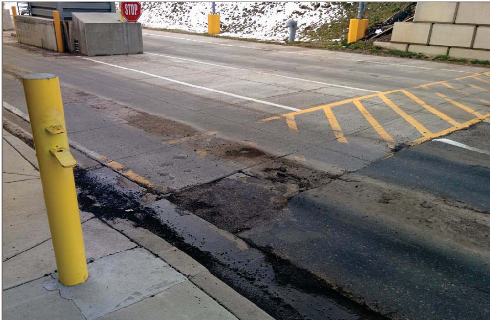
Photo 1: View of the ACP on the Canadian side, and PCCP on the American side. Note rutting in the ACP, and cracking of the PCCP at the transition. The PCCP is otherwise in good condition.
