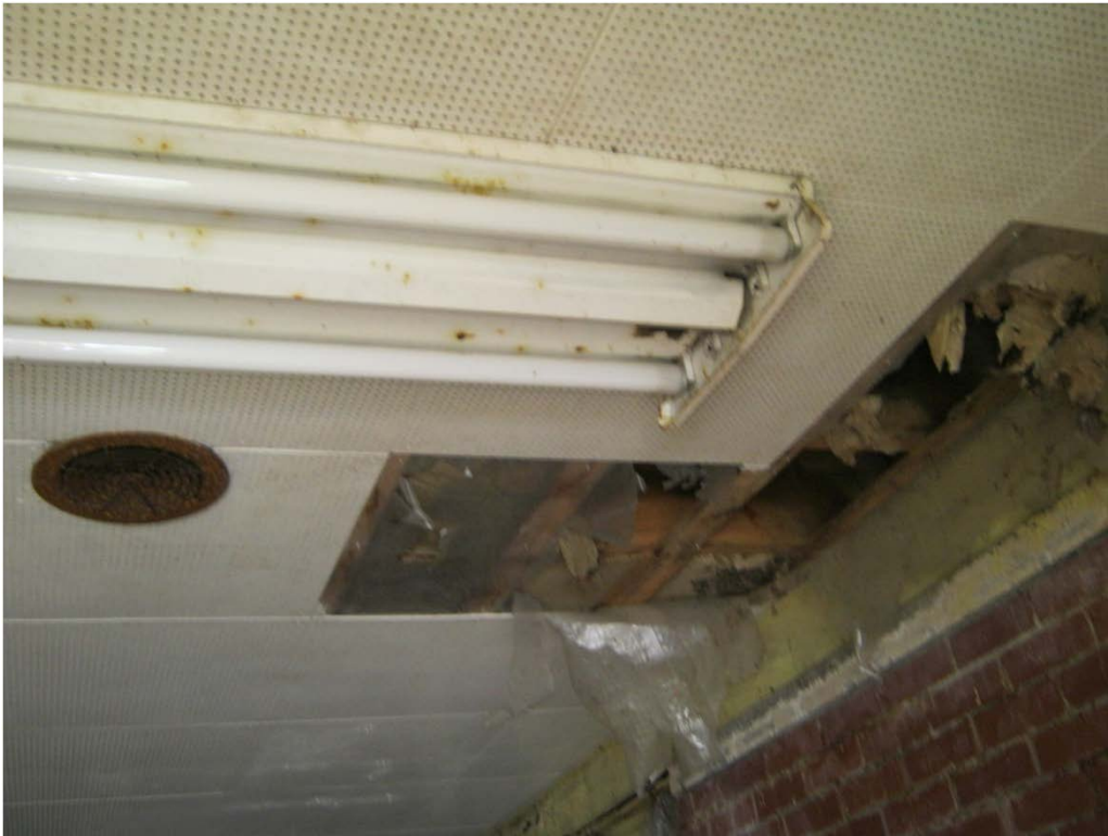
PHOTO 9: View of asbestos-containing 2' x 2' perforated "Transite" cement board ceiling panels (off-white colour) observed in building L9 located at the Point Wolfe Campground.
