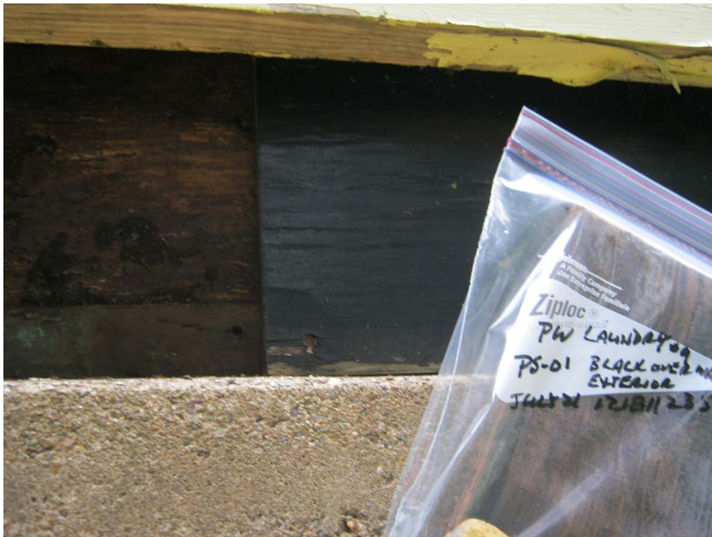
PHOTO 14: View of location of paint sample PW-PS-01 (black over white paint on wood substrate) found to be lead-containing. This sample was obtained from the exterior plywood on building L9 located at the Point Wolfe Campground.
