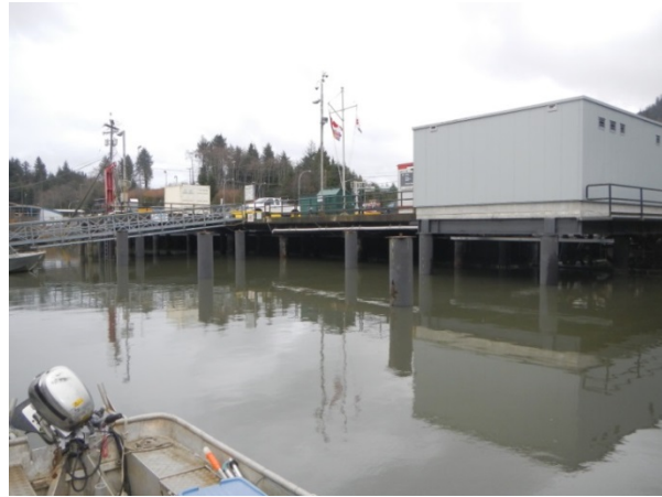
Photo 1-4 Project Site looking Northeast showing Concrete Wharf and Existing Steel Pilings
