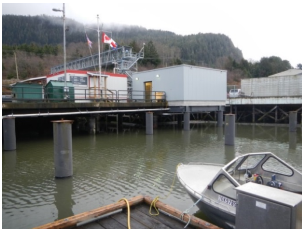
Photo 1-1 Project Site looking Southeast showing Current SAR Station and Existing Steel Pilings
