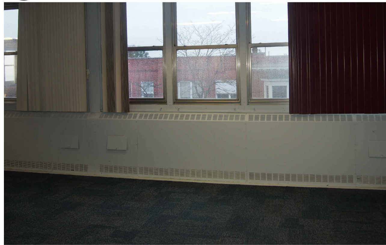
PH #02 OVERVIEW OF EXISTING WINDOWS NTS
