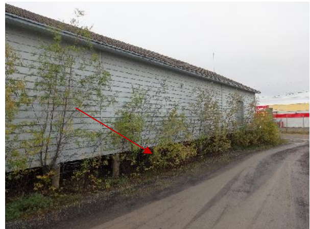
Photo 38: View of access to crawlspace underneath Warehouse #3 building.
