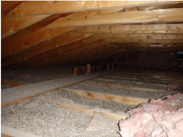
Photo 21: View of structural members within attic space of 15 Nanuk Place.
