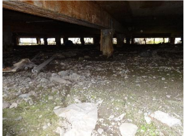
Photo 50: View of structural members within crawlspace of Trade Shop.
