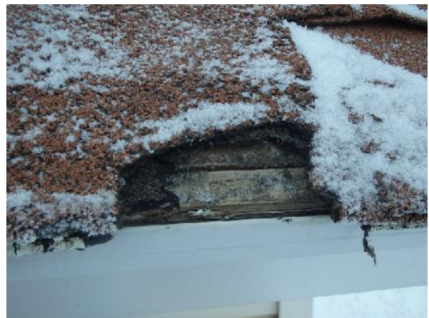
Photo 36: View of wood lath underneath asphalt shingles at 221 Mackenzie Road.
