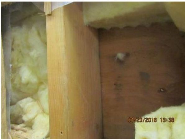
Photo 59: View of wall stud sheeting and insulation at Trade Shop.
