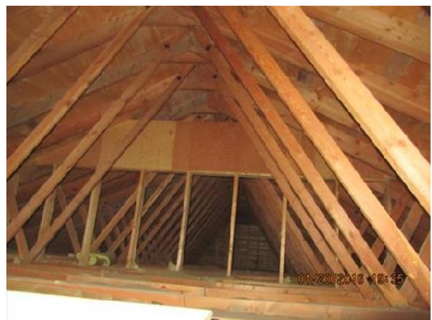
Photo 42: View of roof trusses at Warehouse #3.
