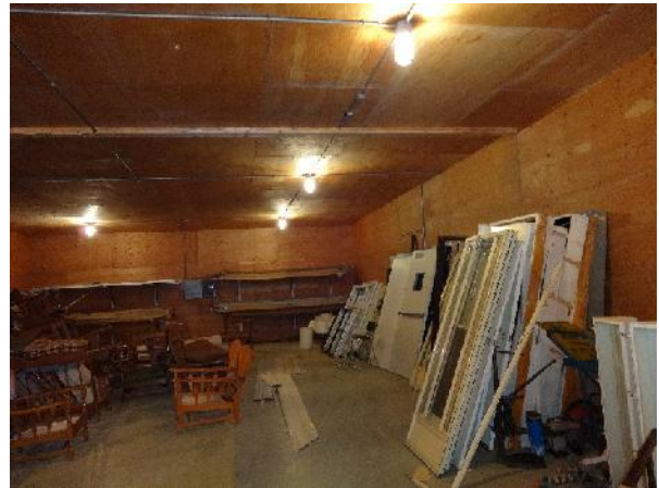
Photo 40: View of interior finishing within Warehouse #3 building.
