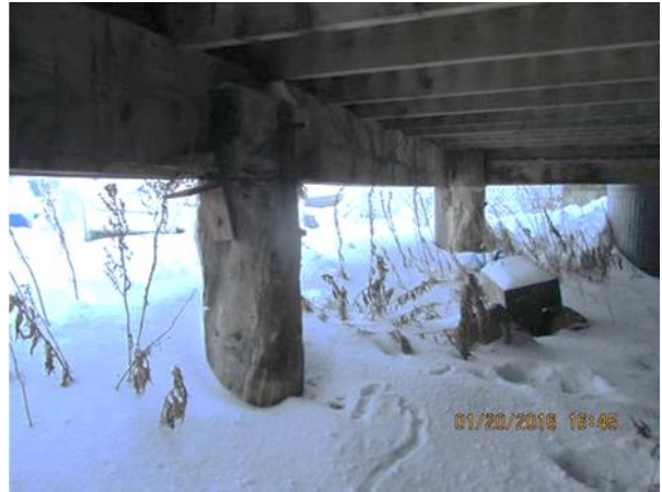
Photo 56: View of pile along edge at Trade Shop.
