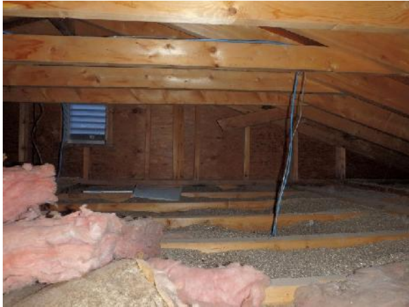
Photo 19: View of structural members within attic space of 15 Nanuk Place.
