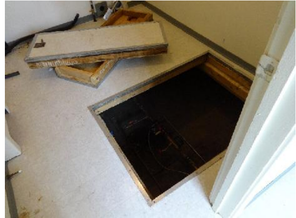
Photo 32: Additional crawlspace access in back entrance at 221 Mackenzie Road.
