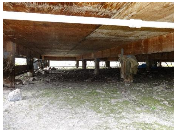
Photo 48: View of structural members within crawlspace of Trade Shop.
