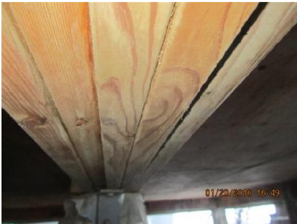
Photo 57: Main floor beam (typical) at Trade Shop.
