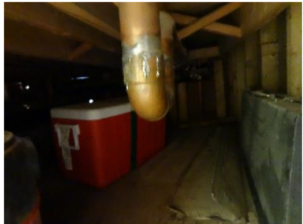
Photo 52: View of crawlspace underneath bathroom of Trade Shop.
