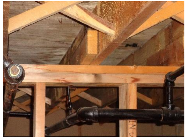
Photo 28: View of structural members within crawlspace of 18 Camsell Place.
