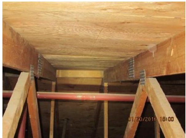
Photo 60: View of roof truss members and truss/sheeting connection at Trade Shop.
