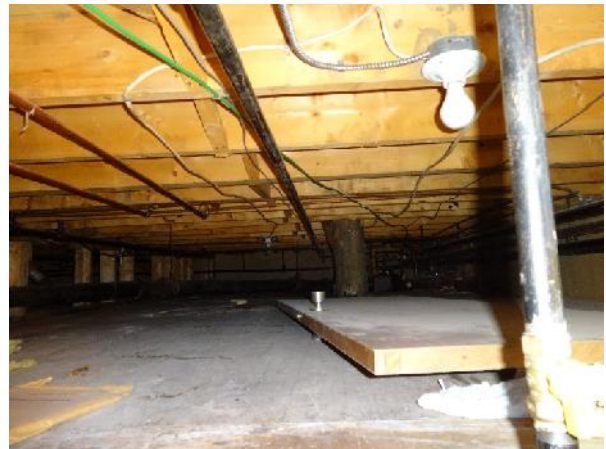
Photo 16: View of structural members within crawlspace of 15 Nanuk Place.
