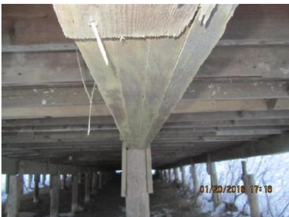
Photo 41: View of 4-ply beam under Warehouse #3.
