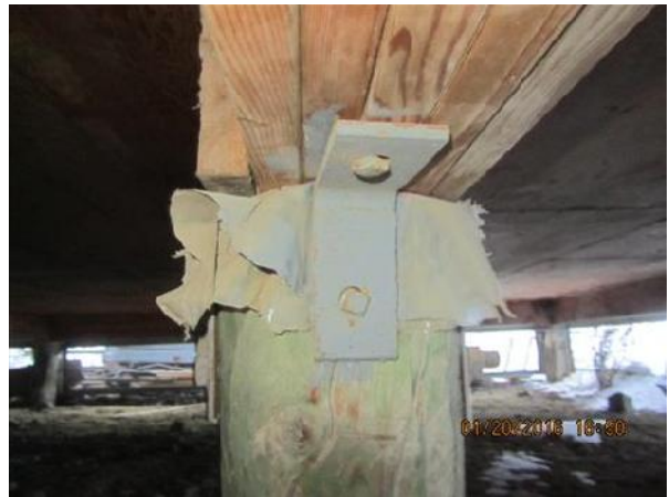
Photo 58: Pile/beam connection at Trade Shop.
