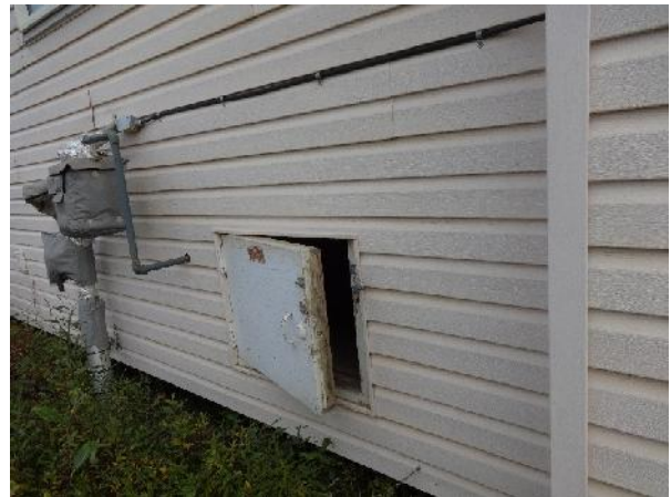
Photo 34: View of exterior crawlspace entry at 221 Mackenzie Road.
