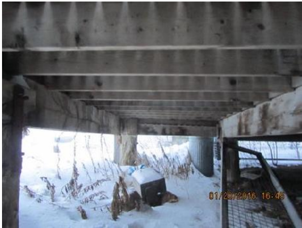
Photo 55: View of structural components under front porch of Trade Shop.
