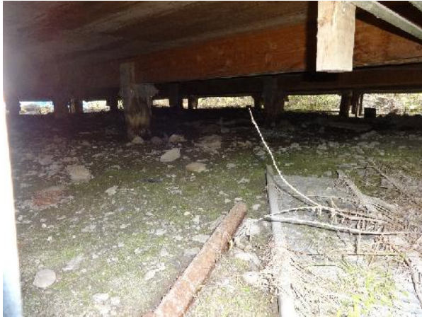
Photo 49: View of structural members within crawlspace of Trade Shop.
