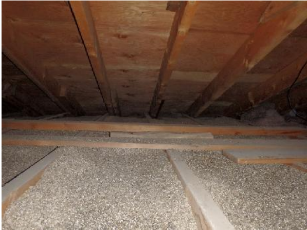
Photo 20: View of structural members within attic space of 15 Nanuk Place.
