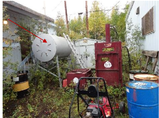
Photo 44: View of above ground storage tank (AST) located directly south of Trade Shop building. AST has an approximate volume of three 3 \text{ m}^3 .
