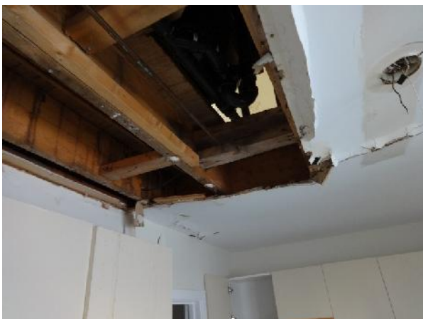
Photo 29: View of structural members located in ceiling cavity of 18 Camsell Place.
