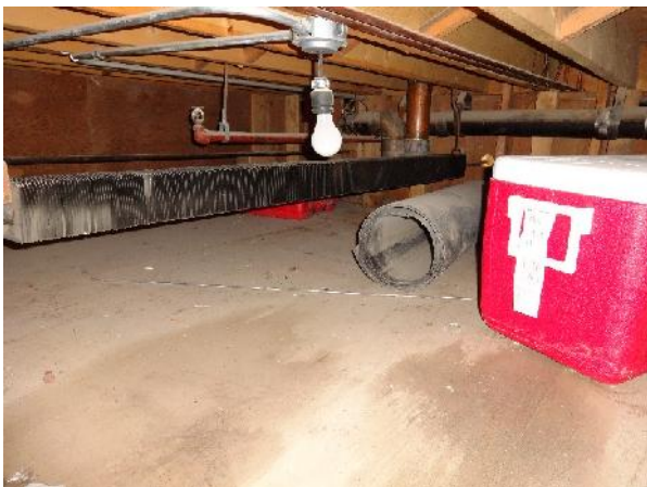
Photo 53: View of structural members within crawlspace under bathroom of Trade Shop.
