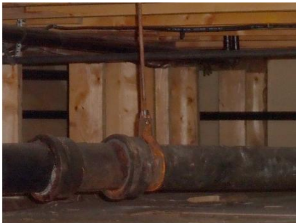
Photo 17: View of cast iron pipe within crawlspace of 15 Nanuk Place.
