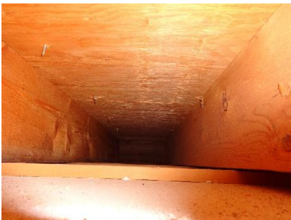
Photo 11: View of initial ceiling cavity directly underneath gypsum board ceiling followed by plywood at 66 and 68 Alder Drive.
