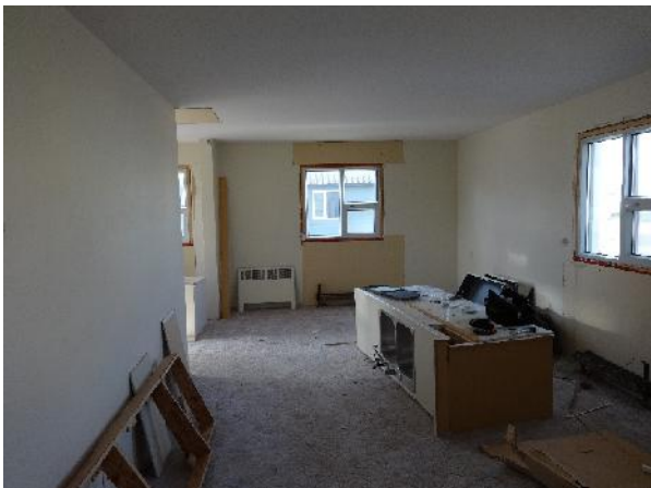
Photo 24: View of interior living room with ceiling height of approximately 2.4 m.
