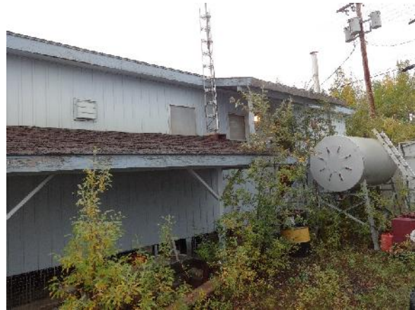
Photo 46: View of overhead power lines located directly east of Trade Shop on right of way, rail line.
