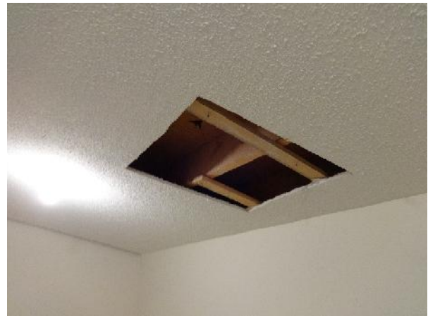
Photo 10: View of ceiling cavity with wood trusses at 66 and 68 Alder Drive.
