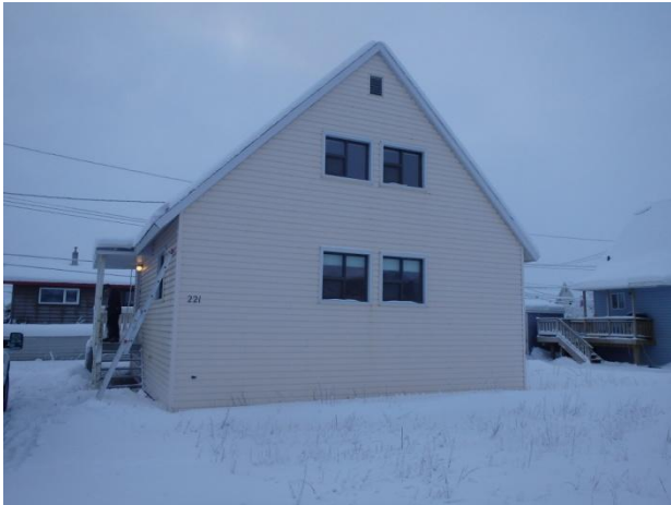
Photo 1: View of front of 221 Mackenzie Road in Inuvik, NT (the "Site").
