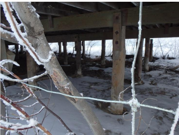
Photo 5: Warehouse crawl space.
