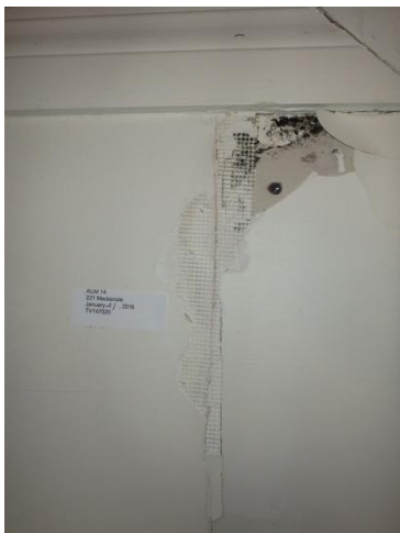
Photo 27: ACM-14, GBJC in bedroom 1 below window. No asbestos fibres detected.
