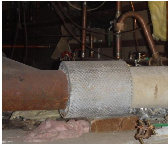
Photo 15: Sample PB04, joint seal between cement coupler and cast iron pipe was determined to contain 125,000 mg/kg lead
