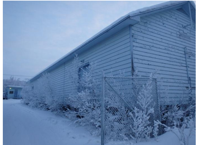
Photo 2: View of rear of warehouse, northwest corner.
