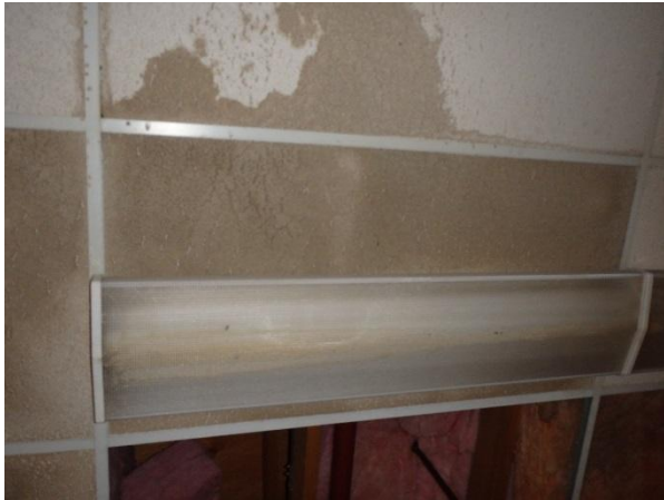
Photo 13: Sample ACM-19; Back Office, suspended ceiling tile; no asbestos fibres detected.
