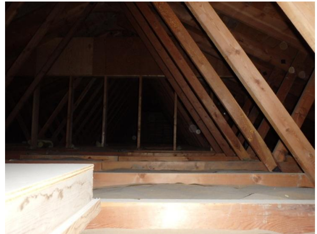
Photo 4: Warehouse attic, looking West.
