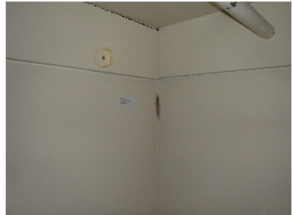
Photo 10: Sample ACM-14, GBJC, master bedroom closet was determined to contain 5% Chrysotile asbestos fibres.
