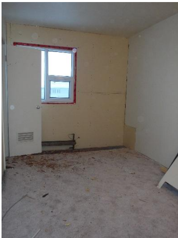
Photo 21: Gypsum board replaced in several areas, including areas around windows.
