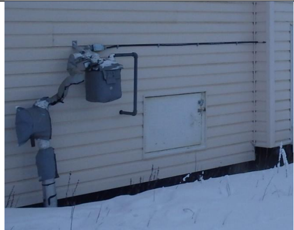
Photo 14: Sample PB03, beige, orange, red, white paint on exterior door to crawl space, was determined to contain 34,400 mg/kg lead.
