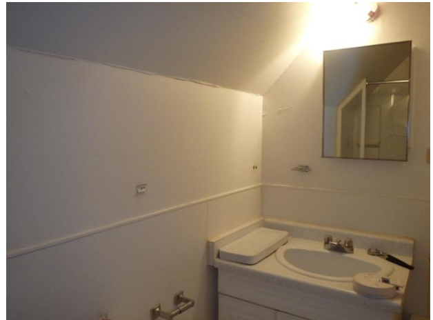
Photo 20: Sample PB09, white paint on sloped ceiling of bathroom was determined to contain 370 mg/kg lead .
