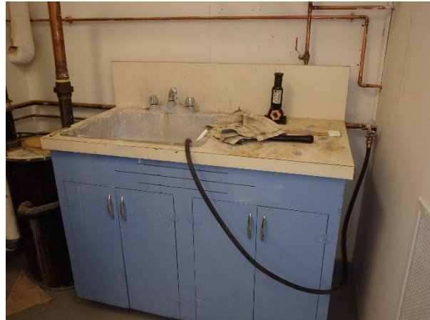
Photo 14: Sample ACM-24; Mechanical room, counter top; no asbestos fibres detected.
