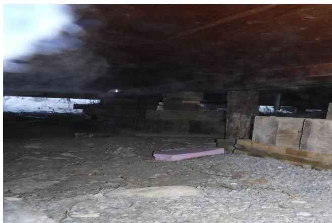
Photo 24: View of the crawlspace and foundation beneath the building.
