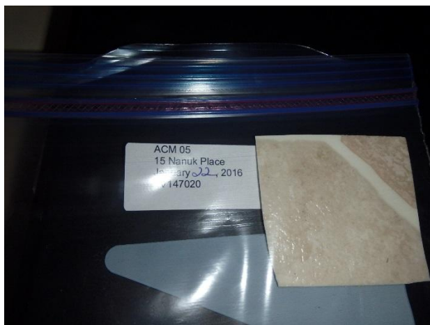
Photo 23: ACM-05, VRF, laundry room. No asbestos fibres detected.
