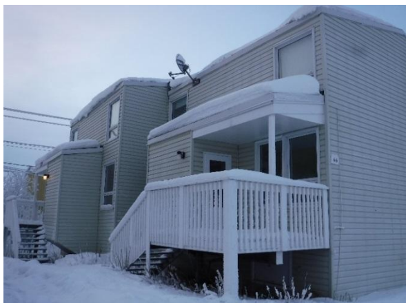
Photo 1: View of 66 & 68 Alder Drive located in Inuvik, NT.
