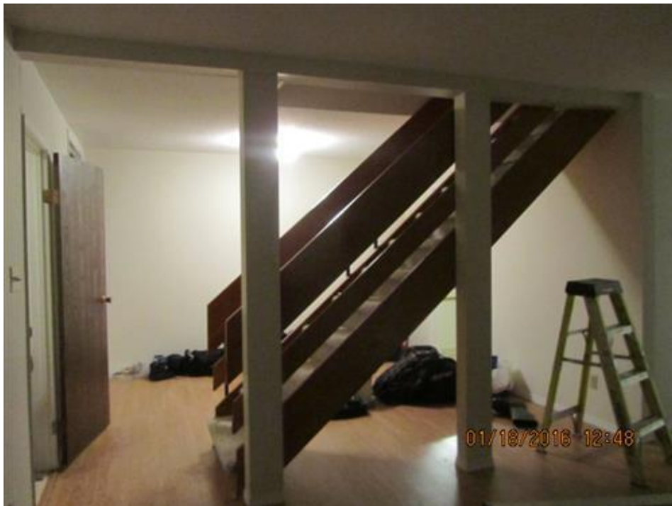
Photograph 12 -Built-up beam and columns along the staircase in House #66
