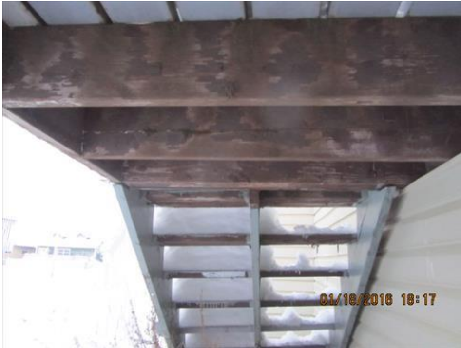
Photograph 45- Condition of beams and joist under the rear porch
