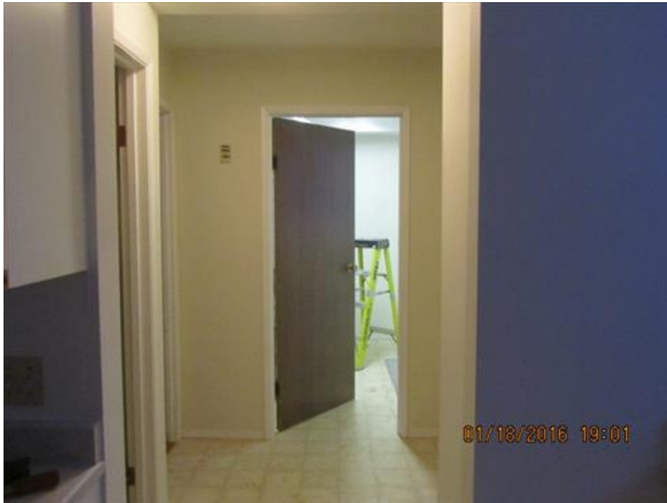
Photograph 60- Back foyer and furnace room-House #68
