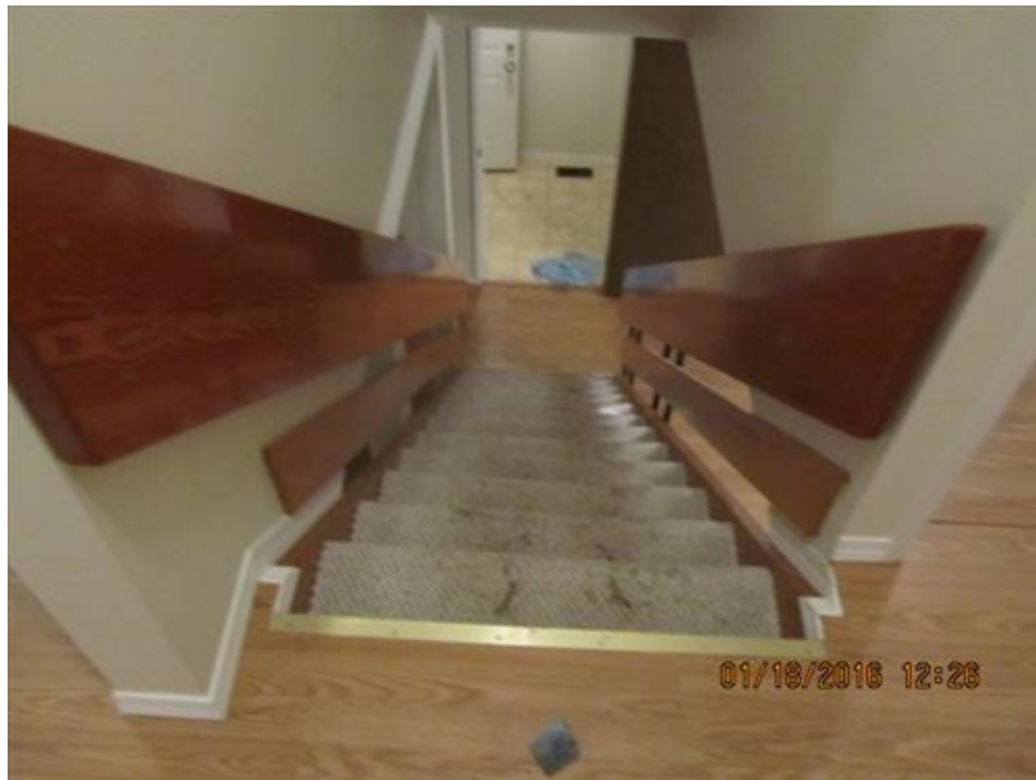
Photograph 54- Stairs from ground floor
