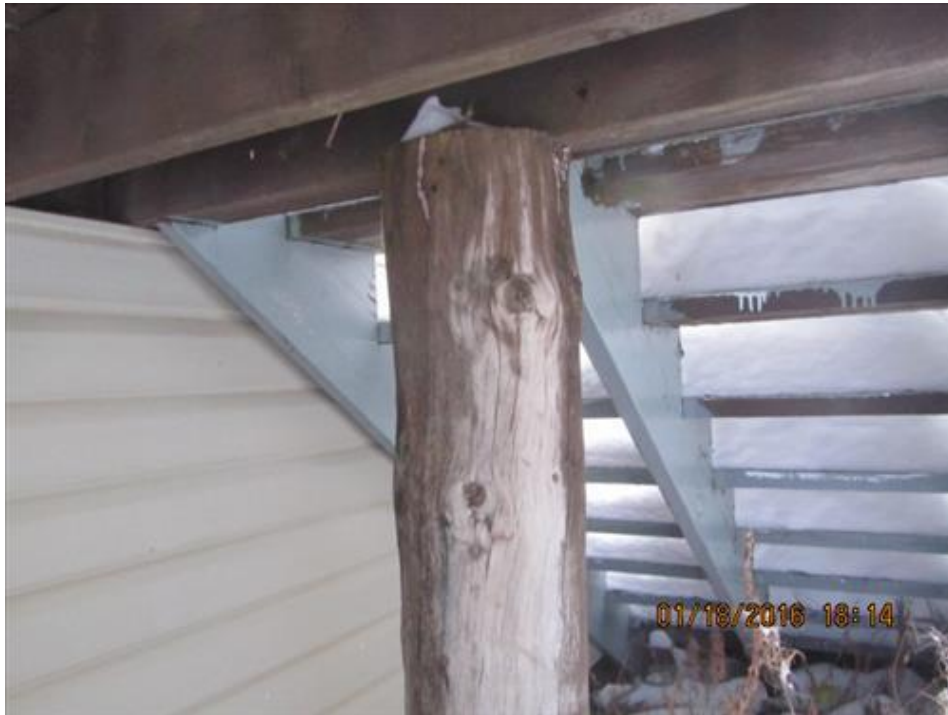
Photograph 15- Wood pile/column supporting the rear stair case and porch of House #66
