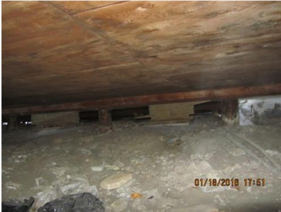
Photograph 21- Temporary supports provided at the north end of building
