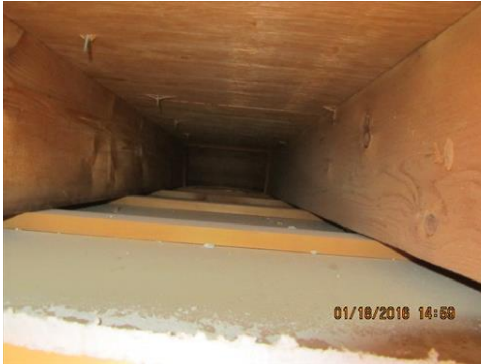
Photograph 13- Joists within the second floor ceiling of House #66
