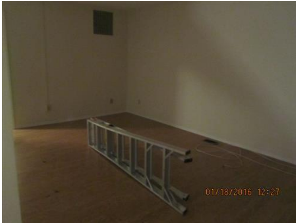
Photograph 51- Ground floor sitting/living room-House # 66
