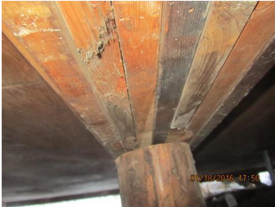
Photograph 5 -Typical main built-up beam placed on the top of driven pile
