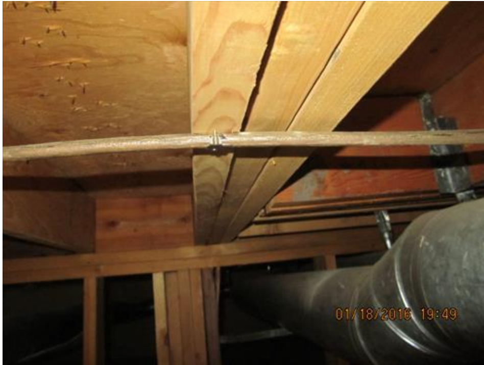
Photograph 9- Built-up beam noted within crawl space supporting the ground floor
