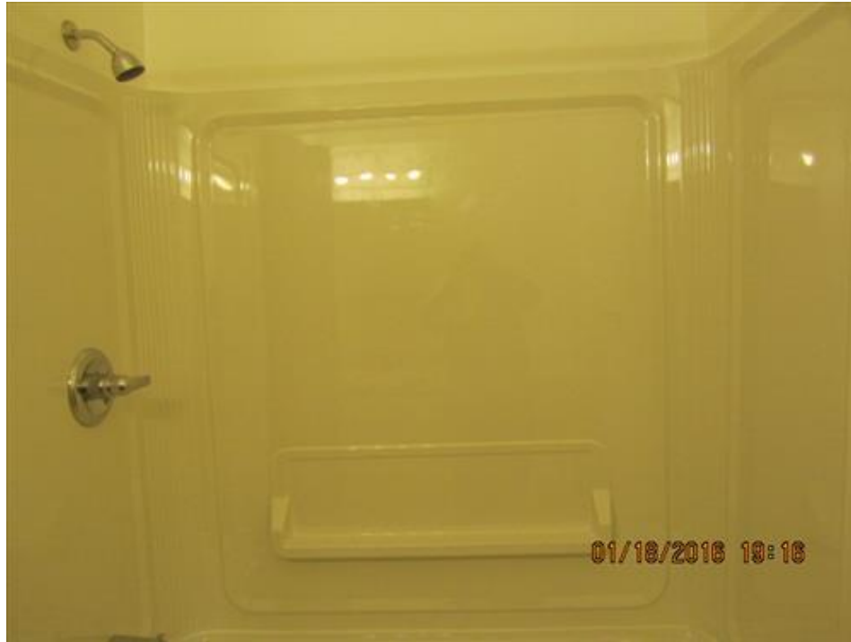
Photograph 63- Bathroom shower – House #68
