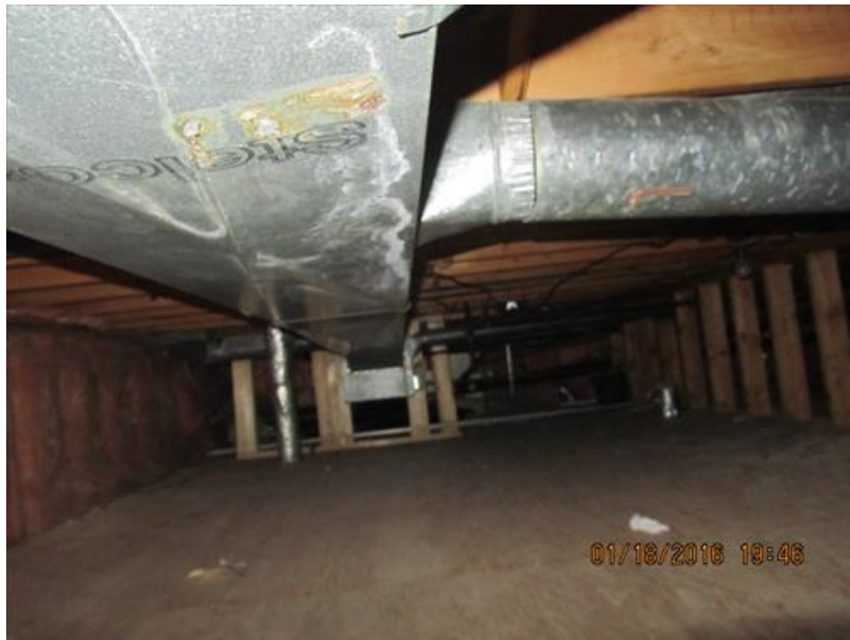
Photograph 6 -General view of raised, enclosed crawl space under the building
