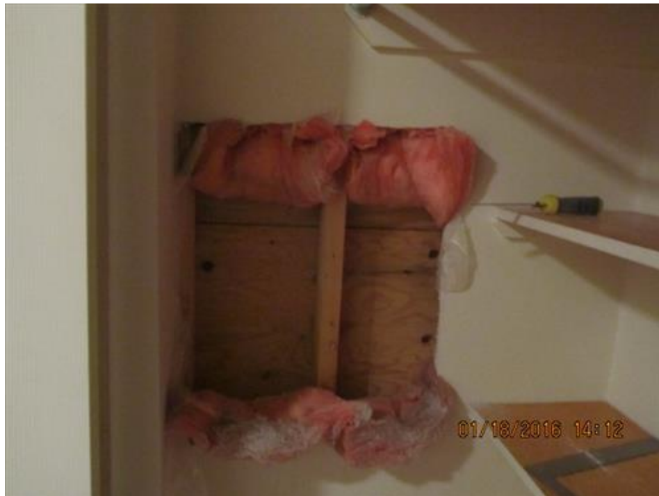
Photograph 48- Exterior wall components noted within the cut-out in second floor bedroom
