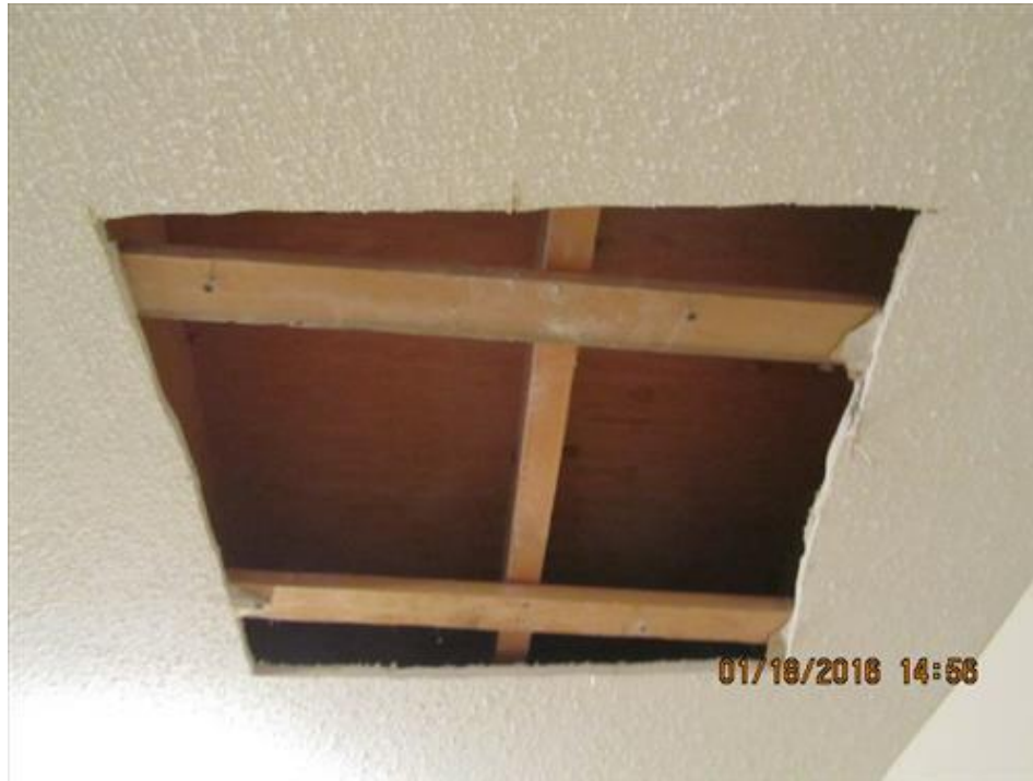
Photograph 103- Roof Joist and lower layer deck sheathing observed through cut-out – House #66
