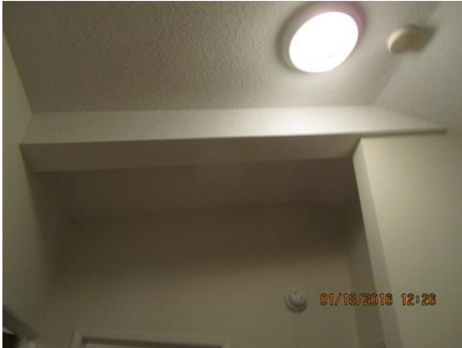
Photograph 11 -Beam within the ceiling of the second floor in House #66
