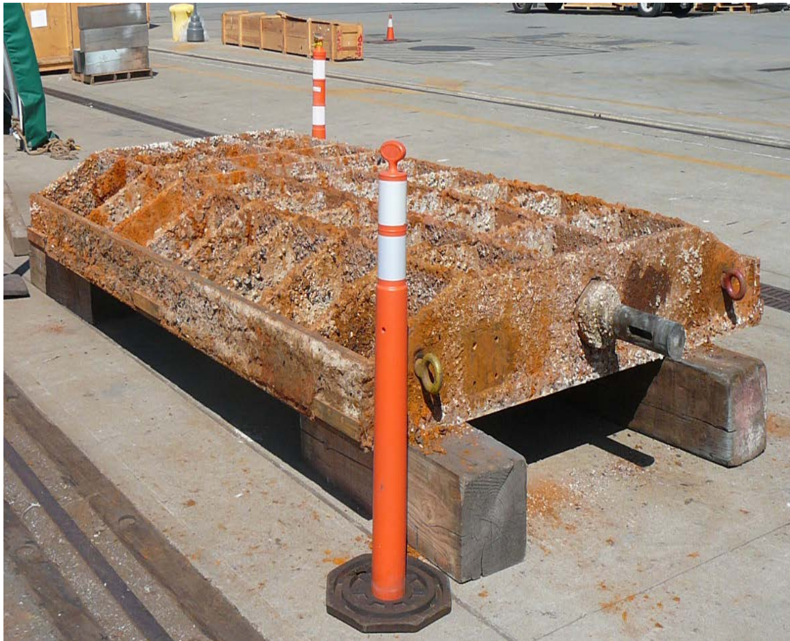
Figure 1. Existing Main Penstock Gate with attachment pin shown below and is provided for reference purposes only.
