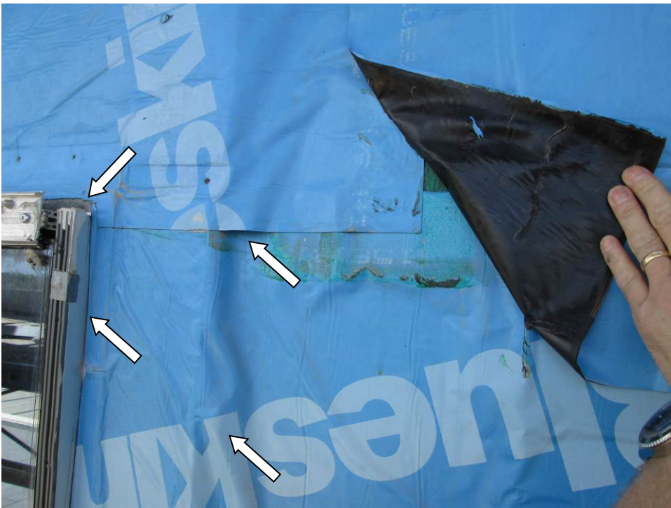
Photograph 12 – Typical Membrane Installation
