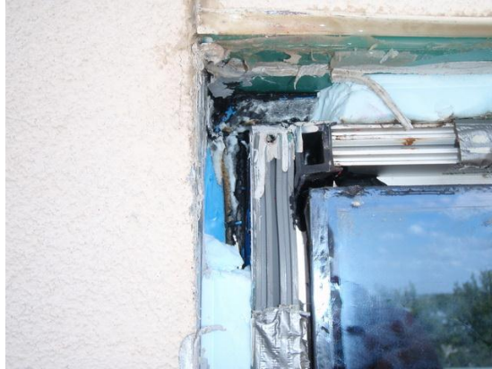
Photo 23: Window head/jamb showing no mechanical fastening of the SBS membrane to the tube face of the curtain wall with an anti-rotation channel.
