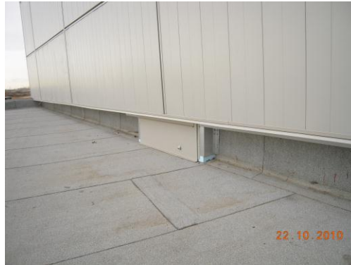
Photo 14: Example from Regional Roof Inspections The insulation and cladding would continue across the upstand SBS membrane that is sealed to the SBS membrane air seal of the wall above.
