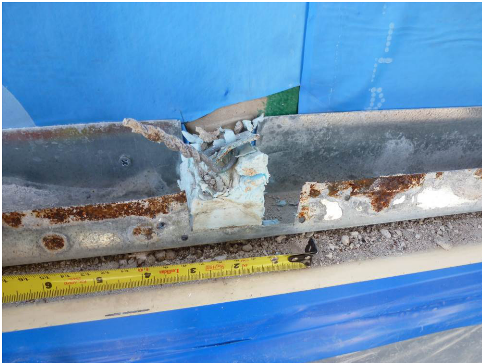
Photograph 20 – Scaffold Tie-Back Note: Membrane not sealed at tie-back location, and corrosion of the subgirt framing.
