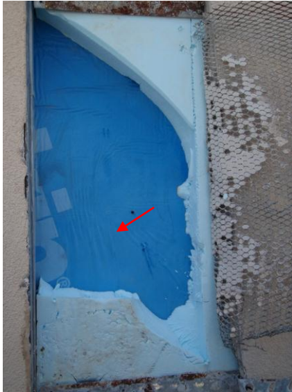
Photo 5, 6: Wrinkles in the membrane means that there is a lack of bond between the gypsum sheathing and the membrane. These voids make increase in time or become collection areas for water to accumulate on the interior of the SBS membrane.
