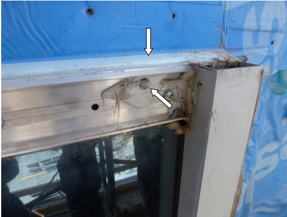
Photograph 23 – Typical Window Head Detail (Flashing Removed) Note: Glazing packet filled with rigid insulation, and weep holes plugged with sealant.
