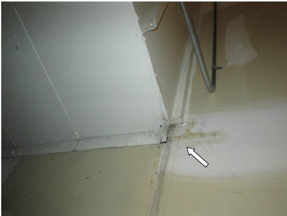
Photograph 18 – East Elevation Louvre Sill Corner Interior Note: Indications of previous water leakage.
