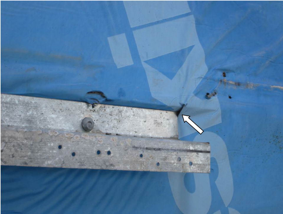
Photograph 15 – Typical Subgirt Note: Membrane tear at end of subgirt where not adequately supported
