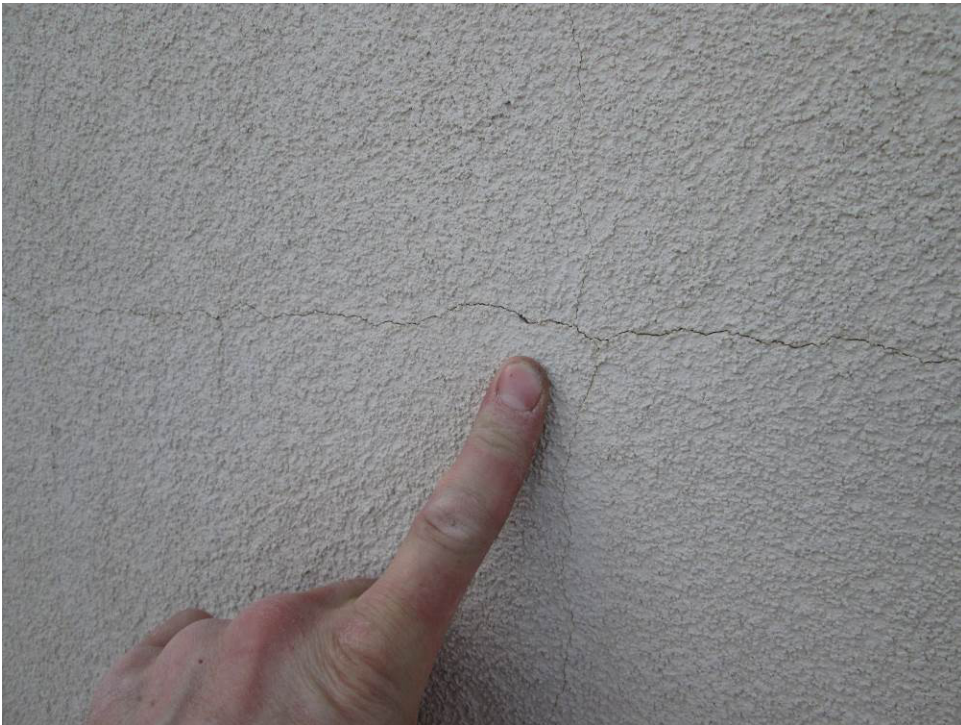
Photograph 4 – Typical Stucco Cracking
