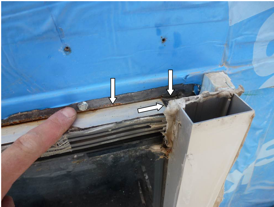
Photograph 24 - Typical Window Head Detail (Pressure Plate and Insulation Blocking Removed) Note: Previous moisture stains, membrane not sealed to framing, unsealed fasteners and corner block, etc.
