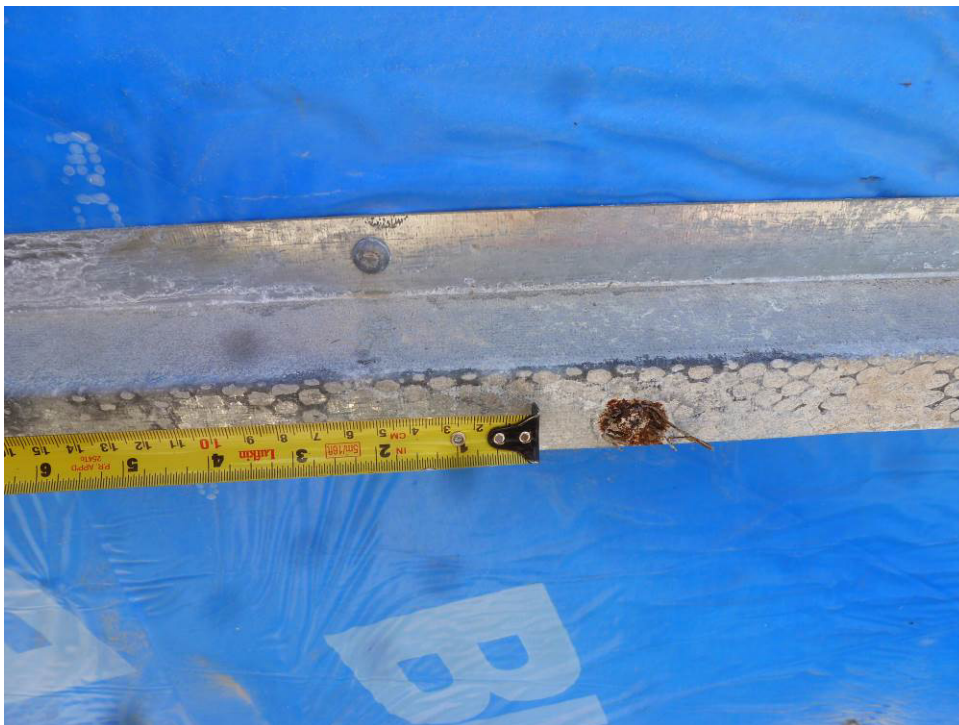
Photograph 8 – Typical Fastener Used to Secure the Metal Lath to the Subgirt Framing
