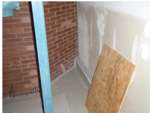
Photo 15, 16: These details provide no indication that the continuity of the air seal or water protection of the original building construction and the newer Annex were joined.
