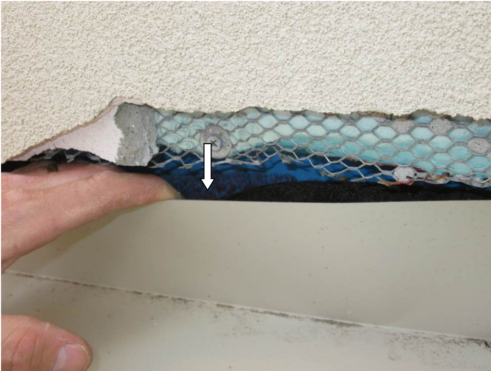
Photograph 27 – Roof Curb Detail, SW Building Corner Note: Roofing membrane not sealed to the wall air/vapour barrier.
