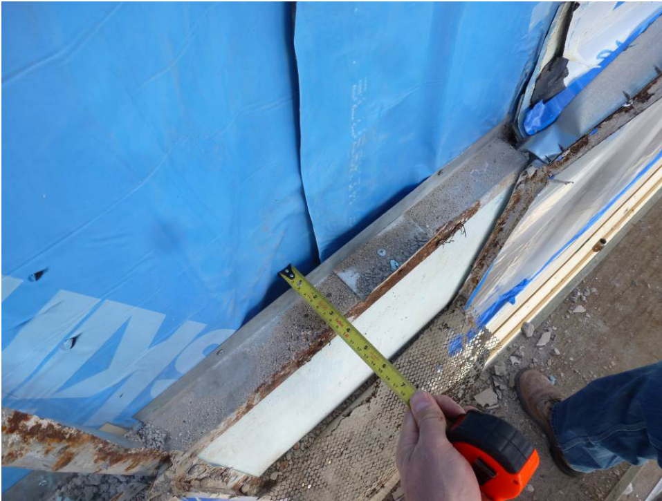
Photograph 21 – Typical Column Detail Note: Large gaps between the insulation and air/vapour barrier membrane.
