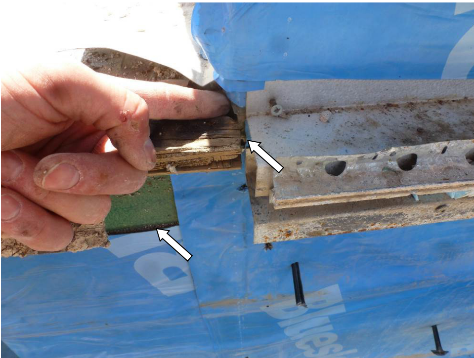
Photograph 16 – Roof Parapet Saddle Detail Note: Membrane not continuous
