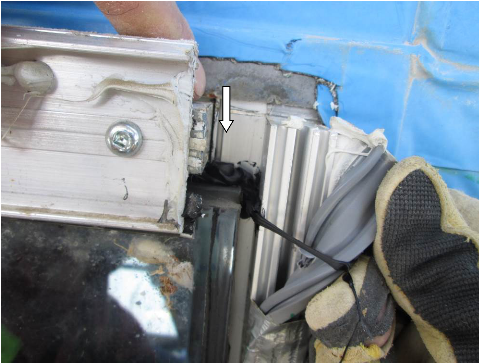
Photograph 25 - Typical Window Head Detail (Corner Block Removed) Note: Corner block not sealed, allowing moisture leakage onto the sealed unit head below.
