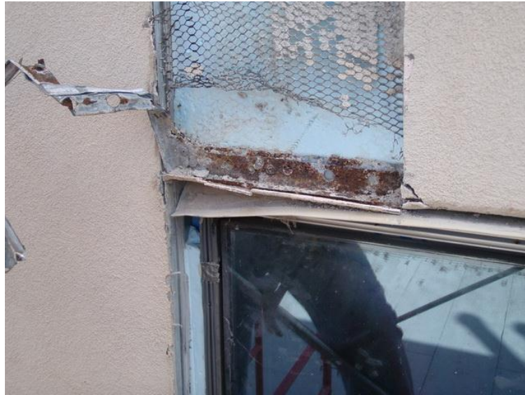
Photo 3: Corrosion of the horizontal metal edge profile. Not significant corrosion on the vertical profile or the lath.
