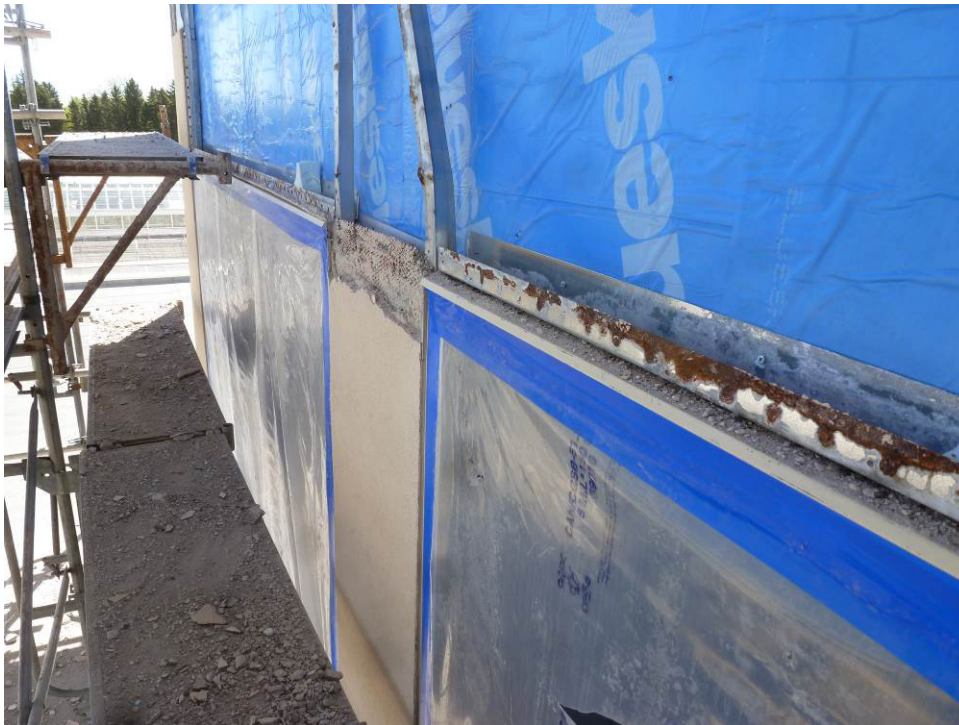
Photograph 7 – Level 3 Window Head Detail
