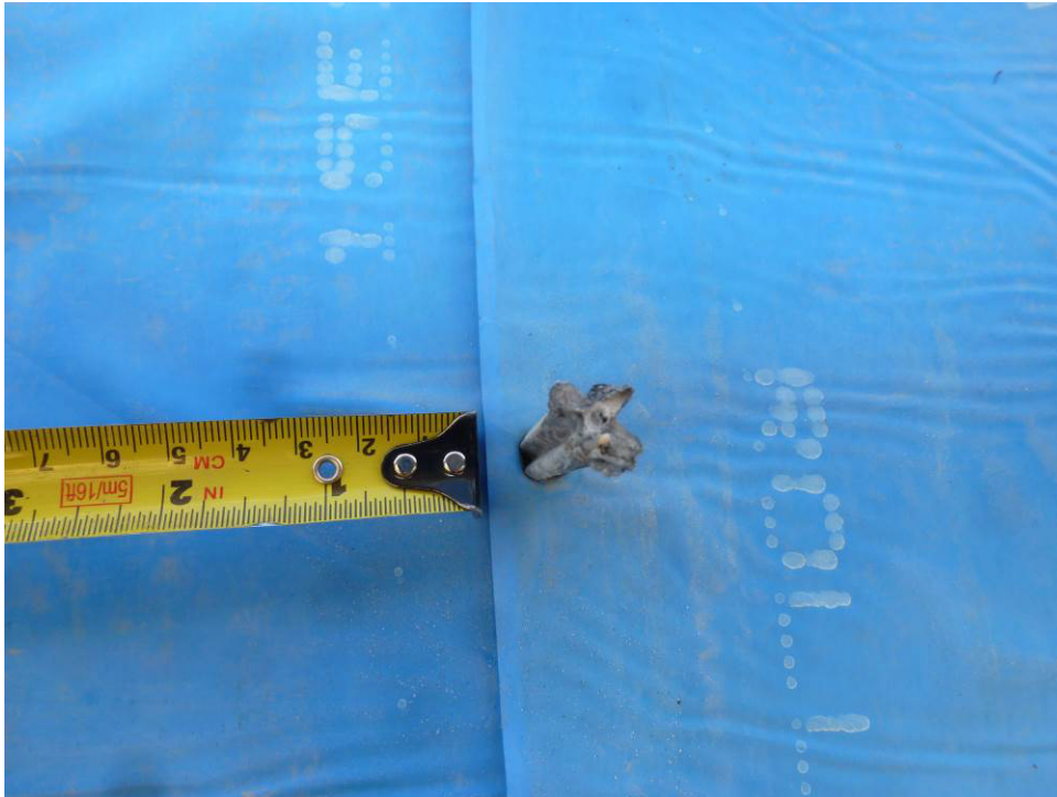
Photograph 19 – Typical Insulation Fastener into Concrete Note: Small unsealed holes through the membrane.
