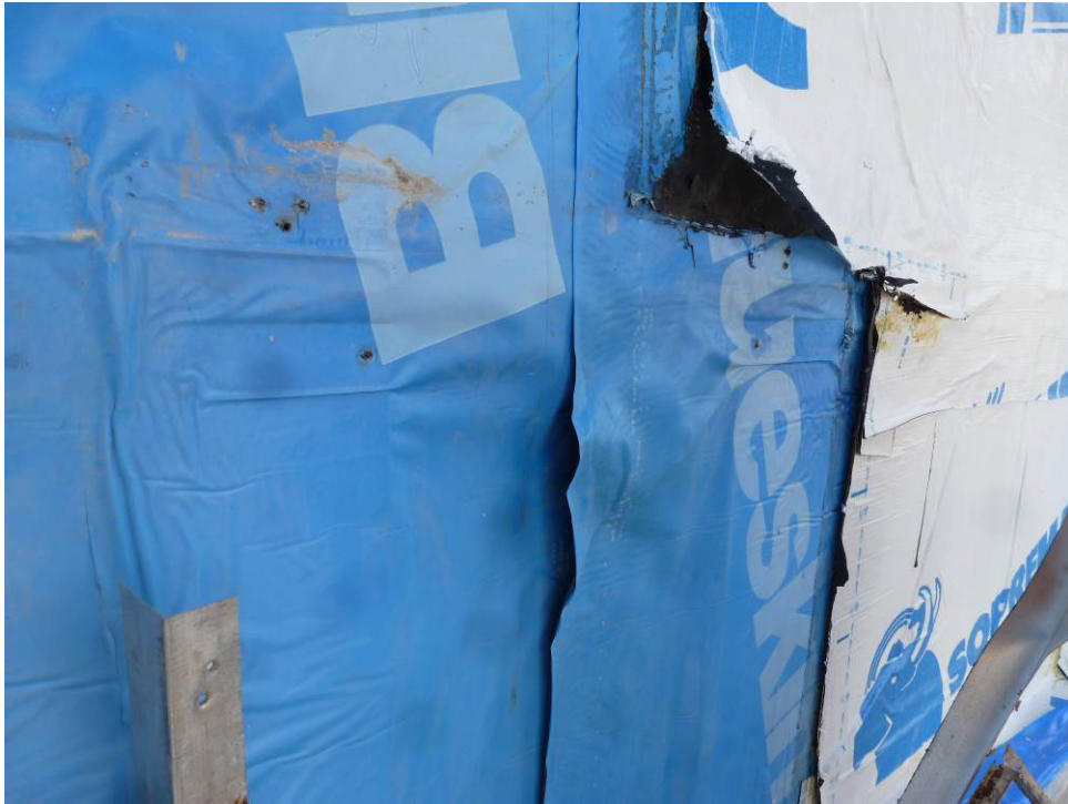
Photograph 13 – Typical Membrane Installation (Blue Membrane Only) Note: Poor bond, open loops at joints, inadequate support at transitions, wrinkles, etc.
