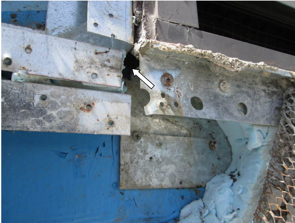
Photograph 17 – East Elevation Louvre Sill Corner Note: Open hole into the wall assembly at the corner.
