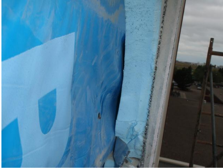
Photo 4: Insulation was not in contact with SBS membrane in some locations.
