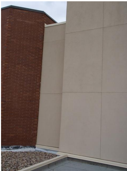
Photo 15, 16: These details provide no indication that the continuity of the air seal or water protection of the original building construction and the newer Annex were joined.
