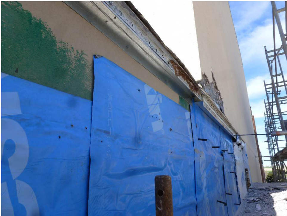
Photograph 14 – Typical Membrane Installation Note: Poor bond at joints, inadequate support at transitions, wrinkles, membrane not continuous to roofing, etc.
