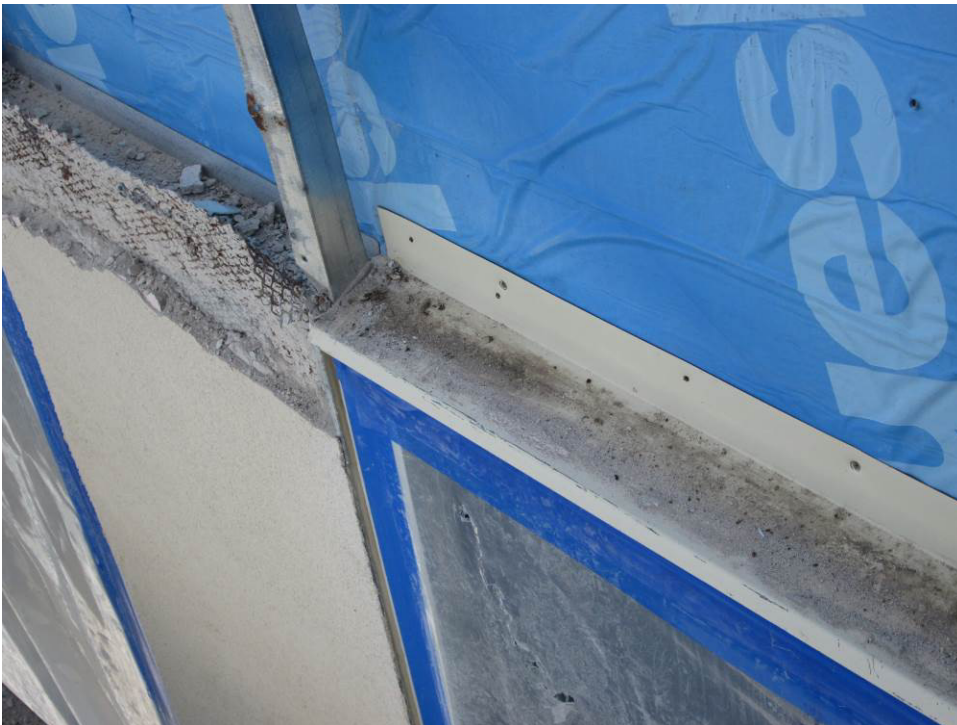
Photograph 22 – Typical Head Flashing Detail Note: Vertical leg of flashing not sealed to the wall, allowing moisture drainage past.
