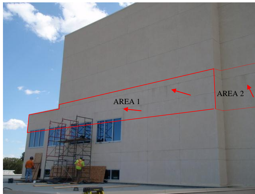
Photo 13: Areas of retrofit 2012. Note staining of the stucco at the horizontal joint in these areas.
