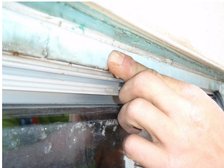
Photo 1: Insulation in glazing rabbet was saturated with water.
