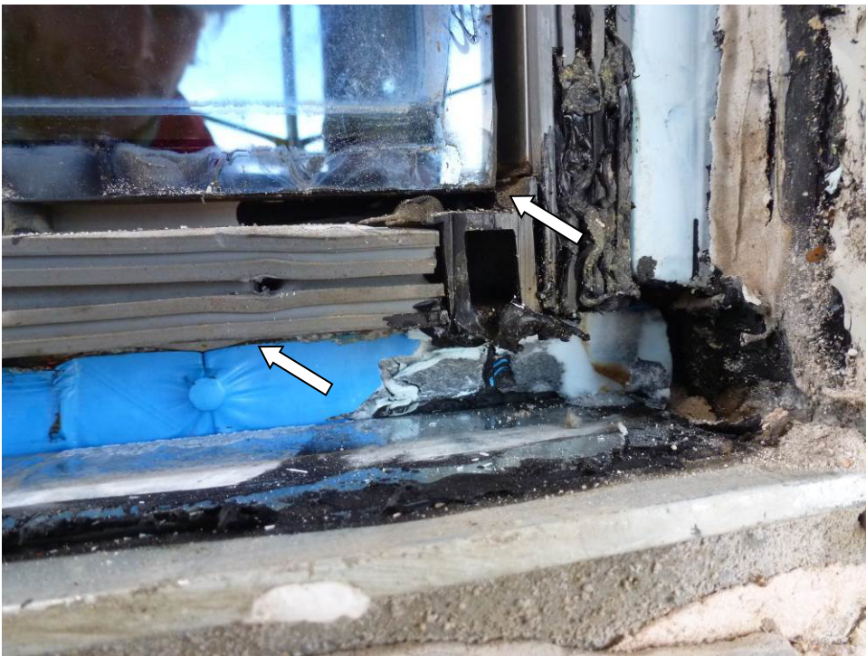
Photograph 26 – Typical Window Sill Corner Note: Excess corner block sealant restricts drainage, and the membrane leading edge not sealed.
