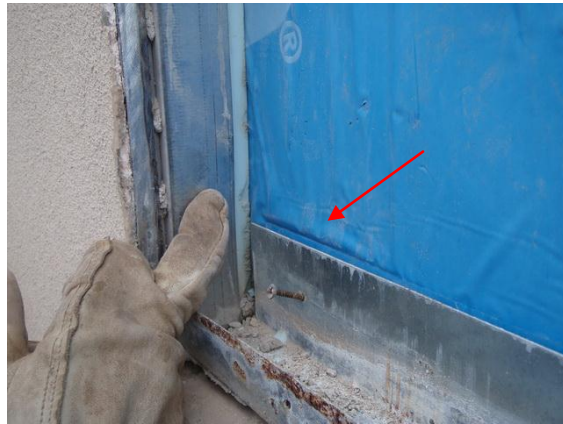
Photo 5, 6: Wrinkles in the membrane means that there is a lack of bond between the gypsum sheathing and the membrane. These voids make increase in time or become collection areas for water to accumulate on the interior of the SBS membrane.
