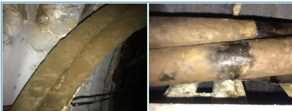
Photo 1 (left) and Photo 2 (right): growth observed along dual unidentified cable, as collected in tape lift sample Tape1, and bulk sample Bulk1
