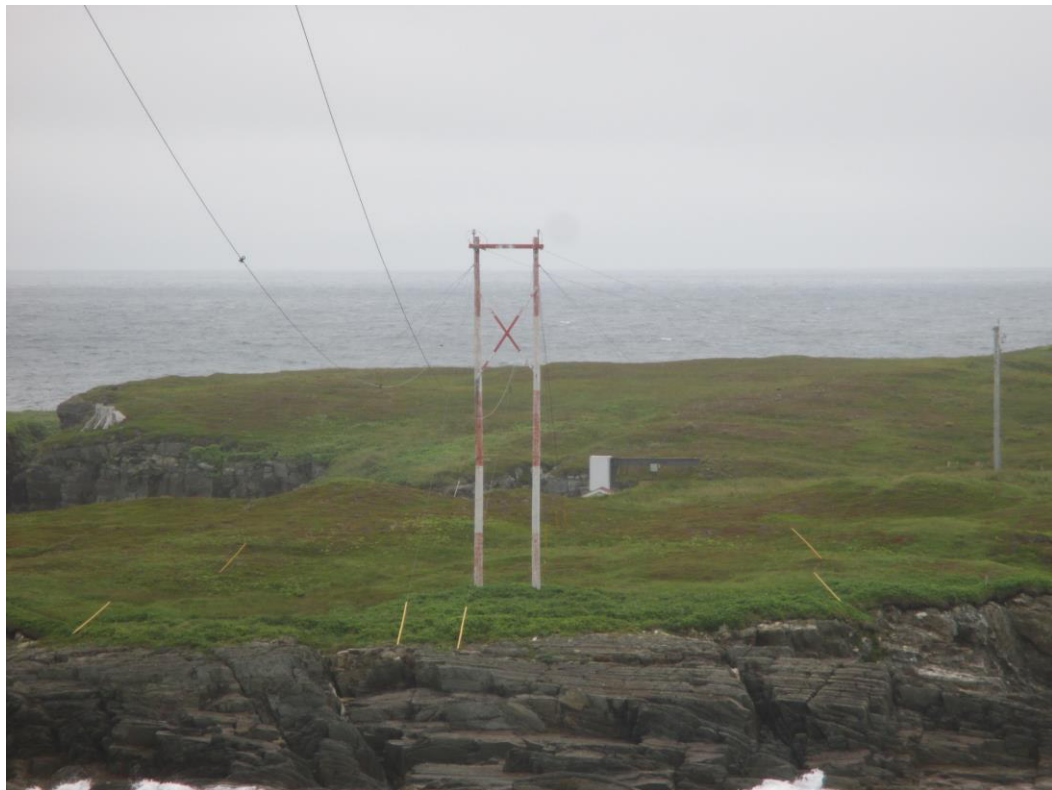
Photo A2: H Frame Structure (Green Island Side)
