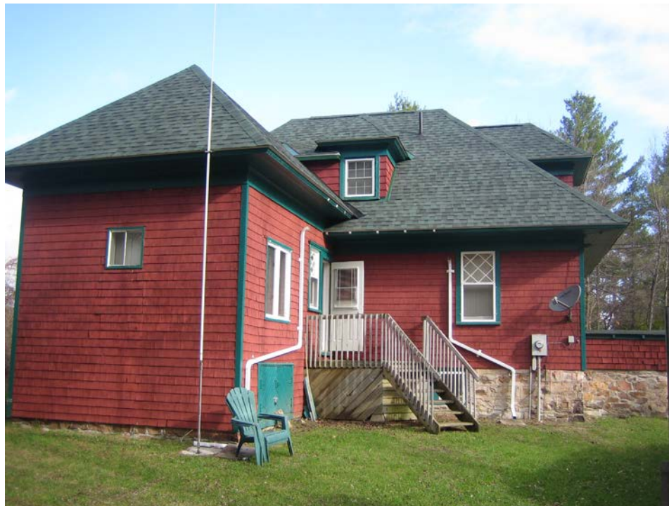
Figure 6: Hill Island IRB Station and Existing Antenna
