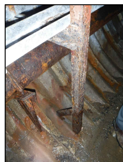
TYPICAL EXISTING ANGLE SUPPORT BRACKET
