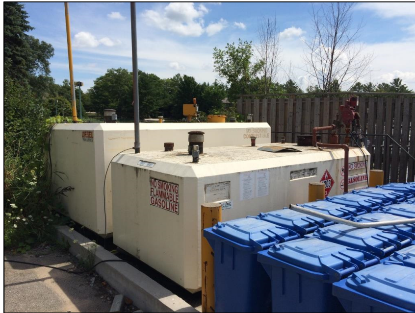
Photo 3 – View looking southeast at existing “Convault” fuel tanks to be removed. Underlying concrete tank dike and bollards to remain.
