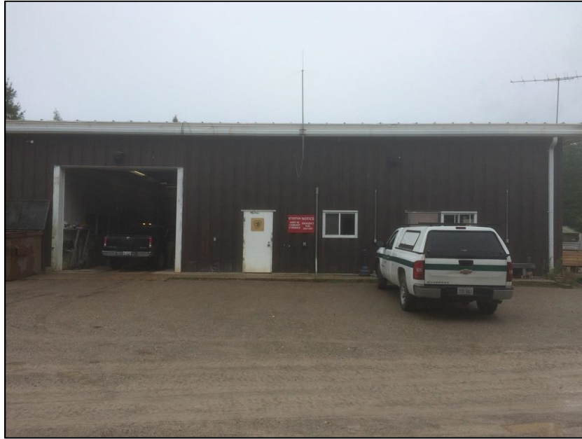
Photo 5 - View looking northeast at Maintenance Building from existing aboveground fuel tank system. Existing fuel pump E-Stop and sign mounted to the right of the white personnel door.
