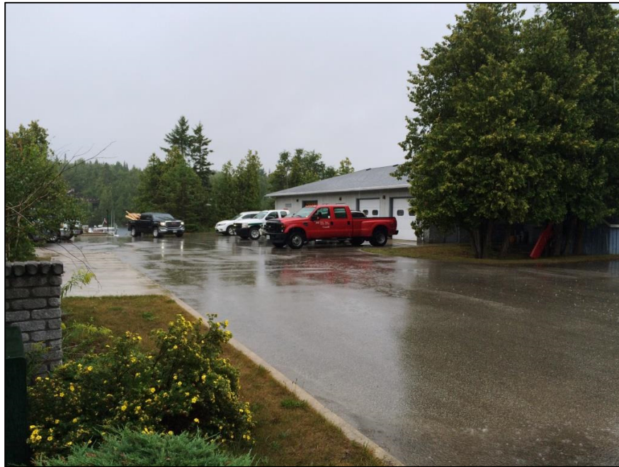
Photo 1 - View looking south towards the Marine Base Operations Storage Building. Existing aboveground fuel tank system to be removed is to the left of the black pickup truck in the photo.
