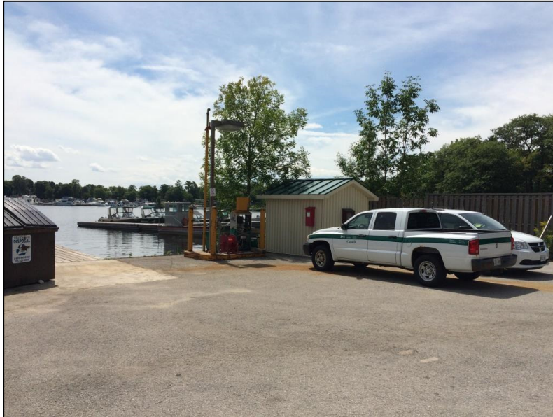
Photo 5 – View looking southwest at existing fuel pump island, bollards, fuel pump, hose reel, light standard and shed to left of dock to be removed. Approximate location of new aboveground fuel tanks corresponds with the location of the two vehicles in the photo.
