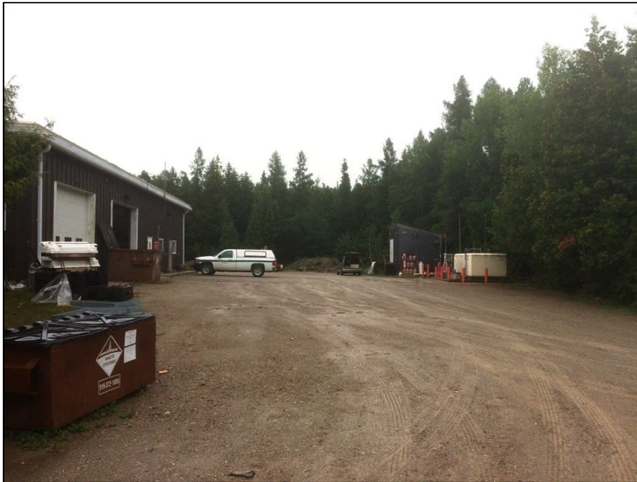
Photo 1 - View looking southeast. Existing aboveground fuel tank system to be removed is to the right. Cyprus Lake Maintenance Building to the left.
