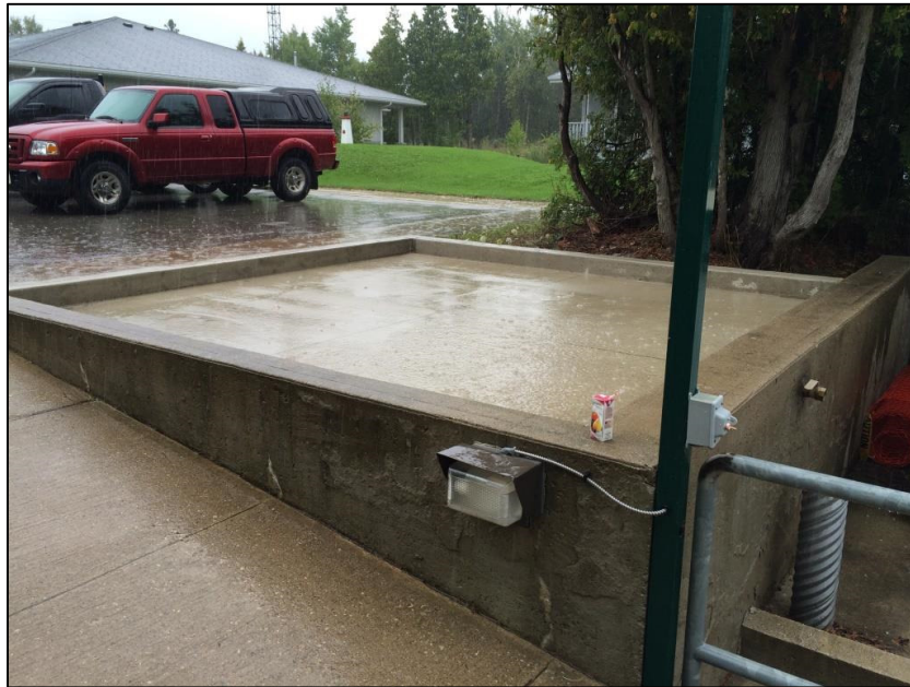
Photo 3 - View looking north at existing concrete product transfer area dike to remain. New aboveground fuel tank system to be installed in background, with approximate fuel tank locations corresponding with the two vehicles visible in the photo.
