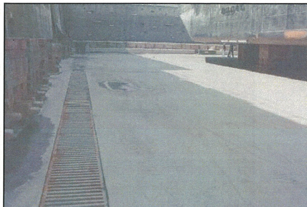
ADEQUATE: Example of a dock floor that would pass inspection.
