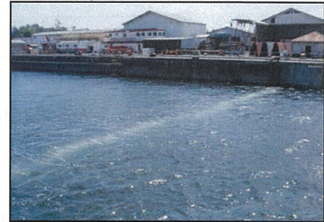
Bubble curtain employed during vessel transfer.
