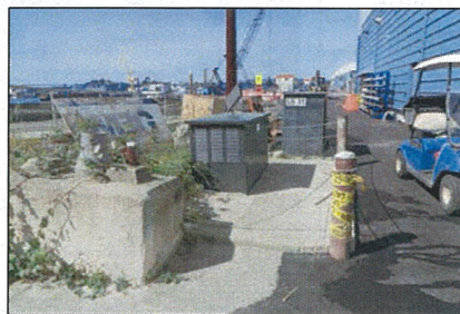
AUTHORIZED Sanitary Sewer Discharge point, Lift Station #11.
