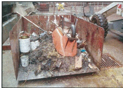
When cleaning dock bottom, skips of waste sandblast grit may leak contaminated water and should be removed as soon as possible.
