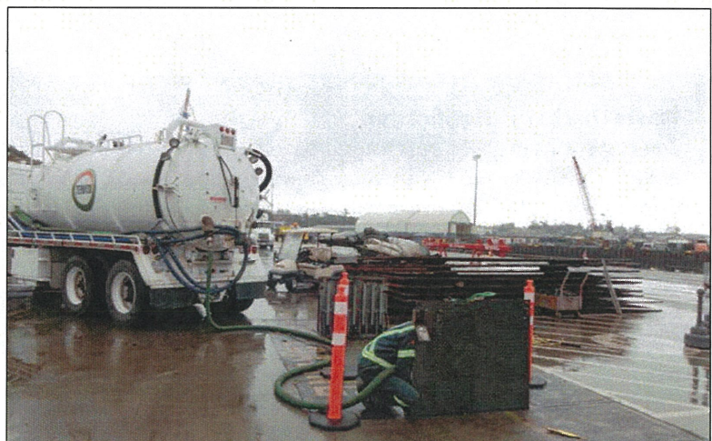
Lift Station Maintenance.
