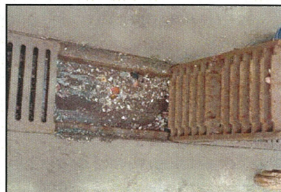
Do not allow trench drains to build up with debris. This helps to prevent flooding during heavy stormwater events.
