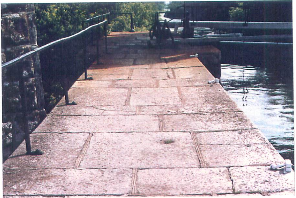
Lock 47 - East Wall Dish-Shaped Settlement Due To Loss Of Fines
