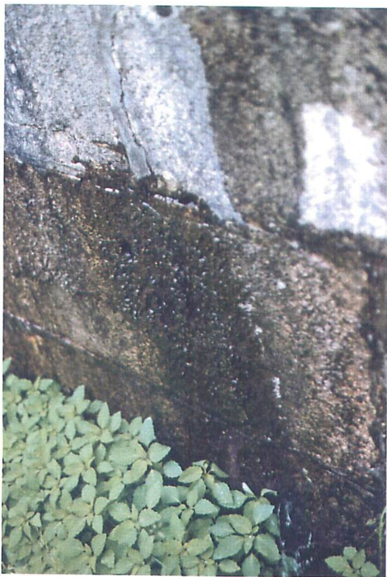
Lock 47 East Wall - External Seepage
