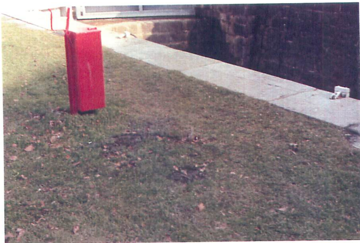
Lock 47 - West Wall Near Test Hole H - 1 Showing Grout Coming To Surface While Grouting
