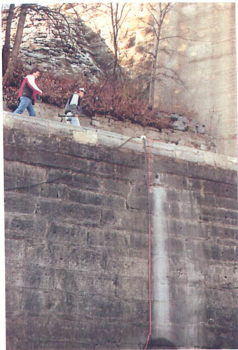
Lock 48 - West Wall Test Hole H - 6 In Vicinity Of Bulge
