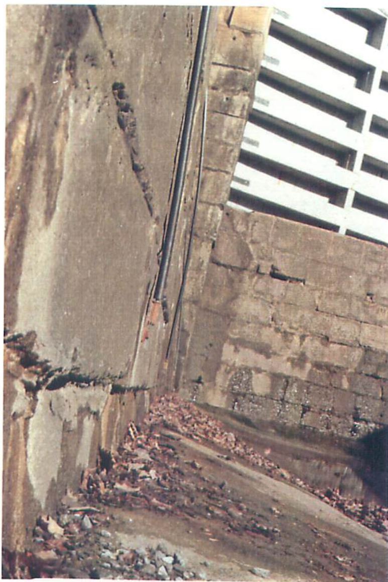
Lock 48 - West Wall Close Up Showing Bulge Due To Freeze/Thaw Action Also Note Movement Of Masonry Blocks And Poor Condition Of Sill With Open Joints & Seepage
