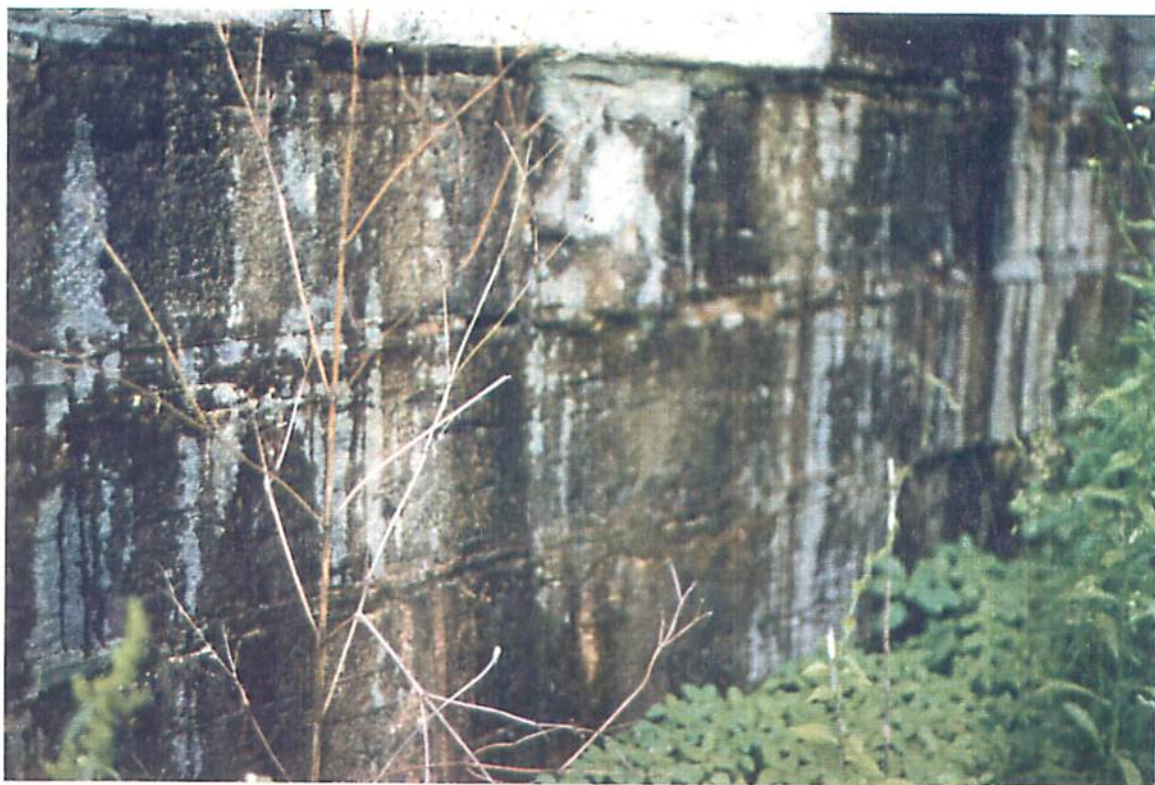
Lock 47 East Wall - External Seepage
