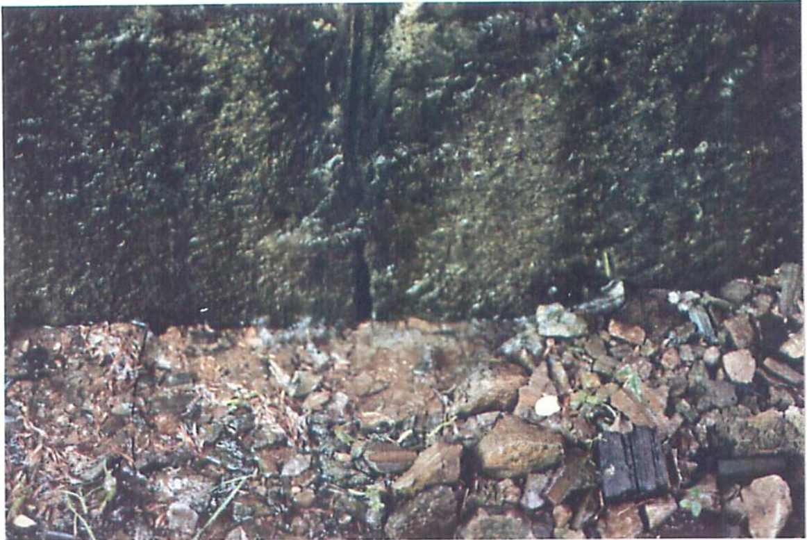
Lock 48 - Exterior East Wall Upstream Abutment Showing Water Leak Through Masonry Prior To Grouting
