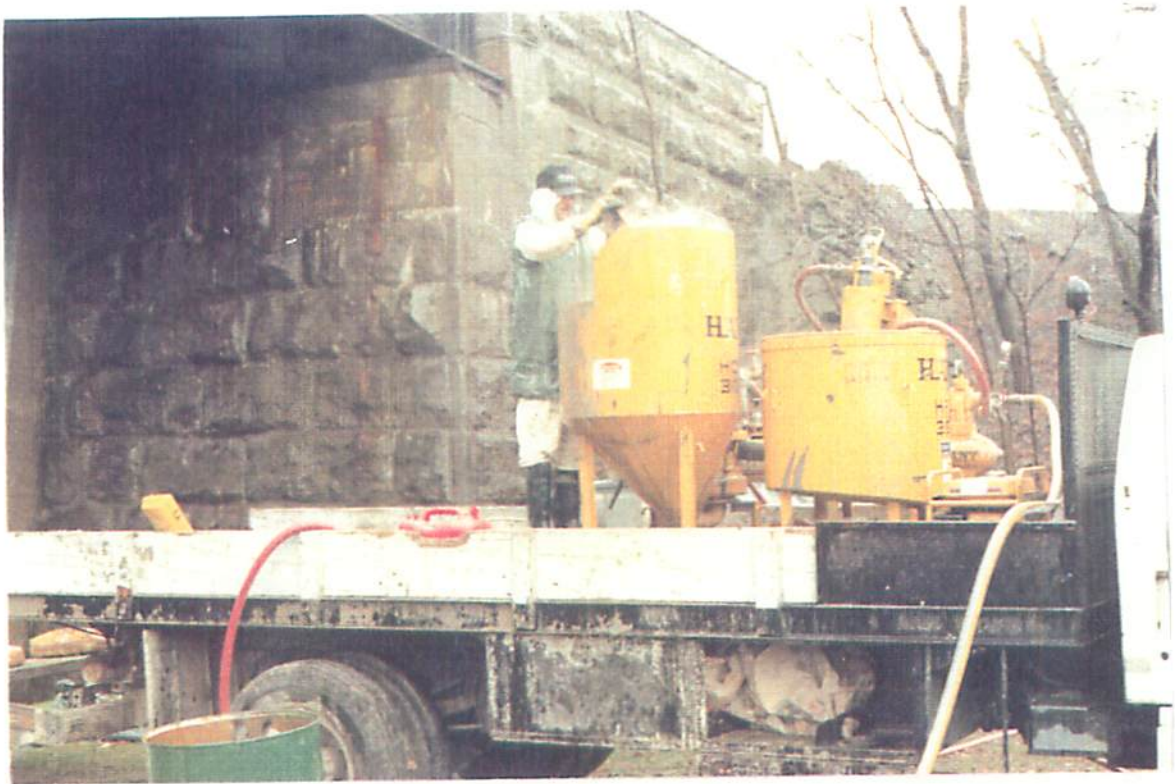
Colloidal Grouting Plant Shown During Test Program Kingston Mills - Nov 1989
