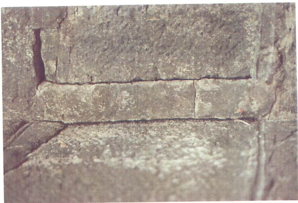
Lock 47 - Showing Open Joints
