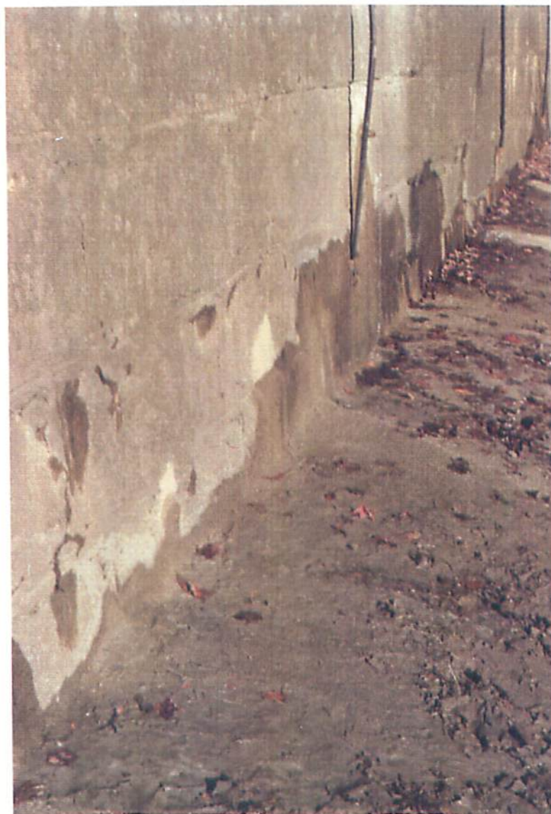
Lock 48 - West Wall Test Hole H - 7 Showing Free Flow Of Water
