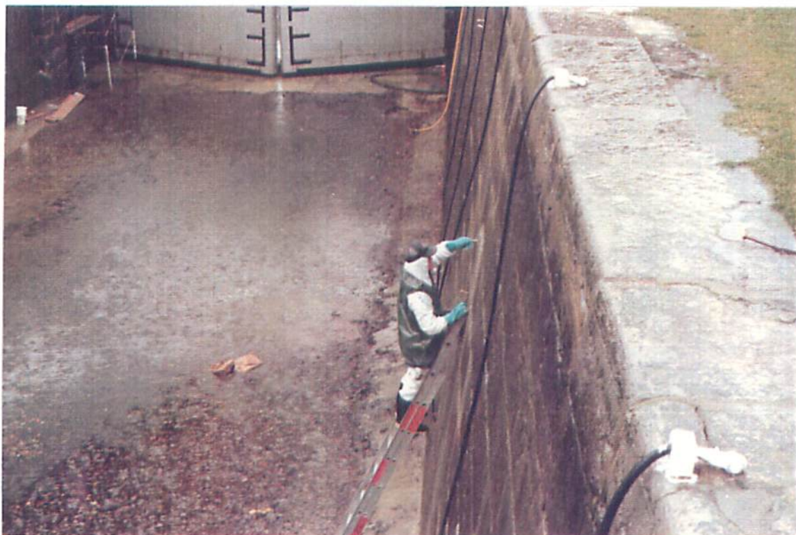
Lock 47 - West Wall Near Test Hole V - 1 Repointing Prior To Grouting With Fast Setting Cement Mortar
