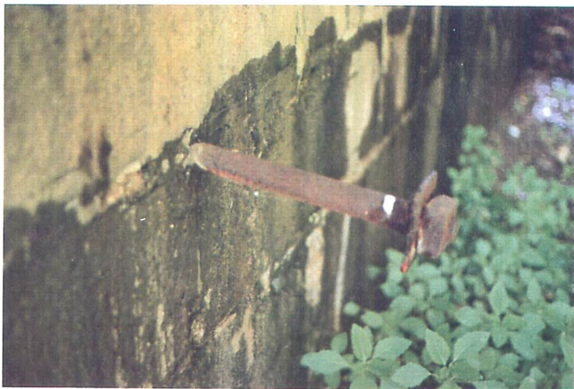
Lock 47 East Wall - External Seepage
