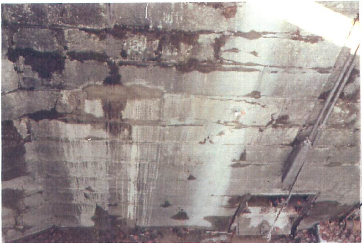
Lock 48 - West Wall Downstream Abutment Showing Grout Leak Through Joint 2 m From Test Hole H - 9
