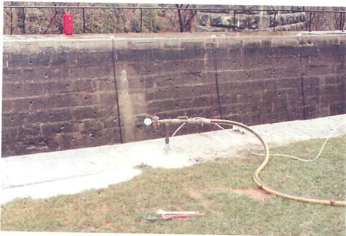
Lock 47 - On West Wall Looking East At Test Hole V - 1 Showing Top Of Hole Assembly & Pressure Gauge While Grouting
