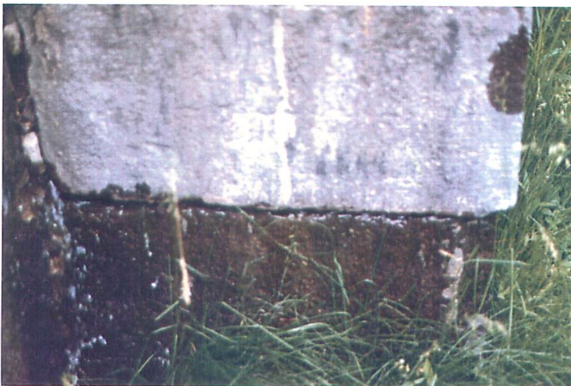
Lock 47 East Wall - External Seepage Note Flowing Water
