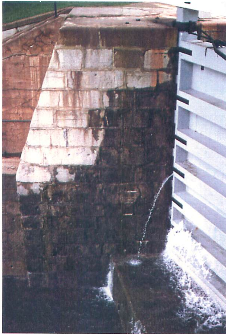
Lock 48 - West Wall At Upstream Gates Showing Seepage Through Abutment from Lock 47
