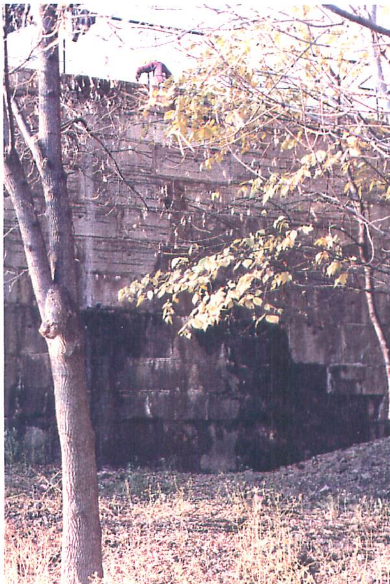
Photograph No. 8 Seepage noted in Run No. 13 - Hole V5
