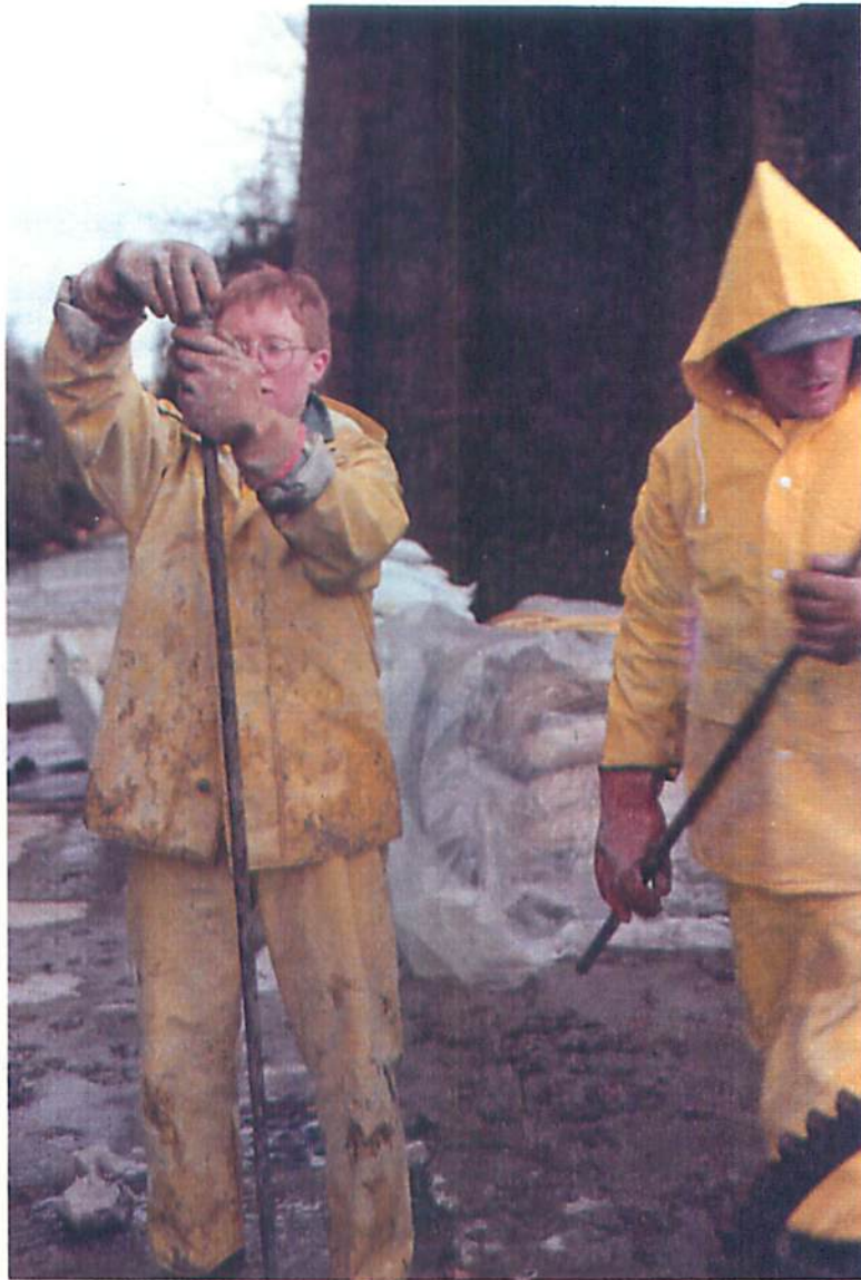
Lock 47 - West Wall Downstream Abutment At Test Hole V - 2 Showing Installation Of Grout Pipes
