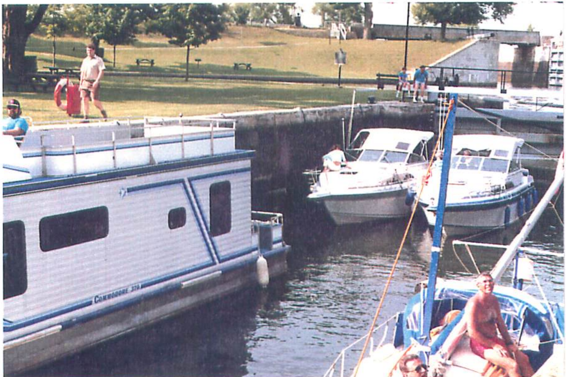
Lock 47 West Wall - Close Up View Note Running Leak Between Boats On West Wall
