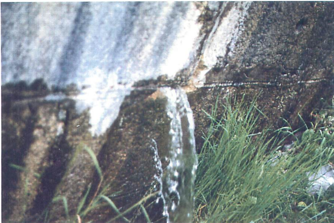
Lock 47 East Wall - External Seepage Note Gushing Leak
