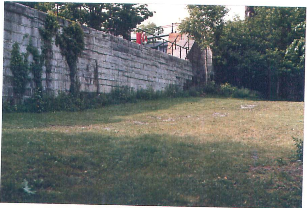
Lock 48 - East Wall Exterior In Much Better Condition Than Lock 47
