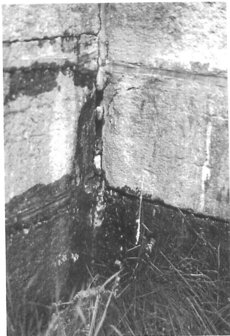
Lock 47 East Wall - External Seepage Close Up Of Flowing Water Leak
