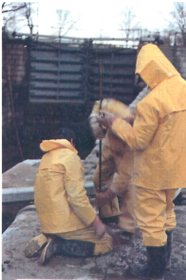
Lock 48 - East Wall Downstream Abutment Pulling Grout Pipe At Test Hole V - 6
