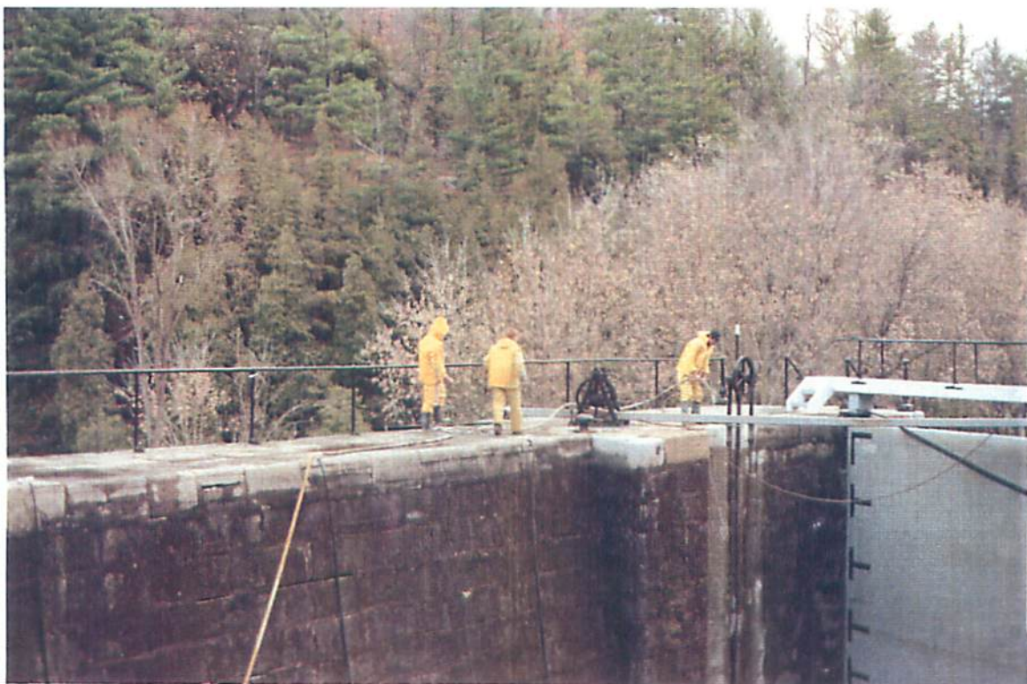
Lock 48 - East Wall Downstream Abutment Grouting At Test Hole V - 6
