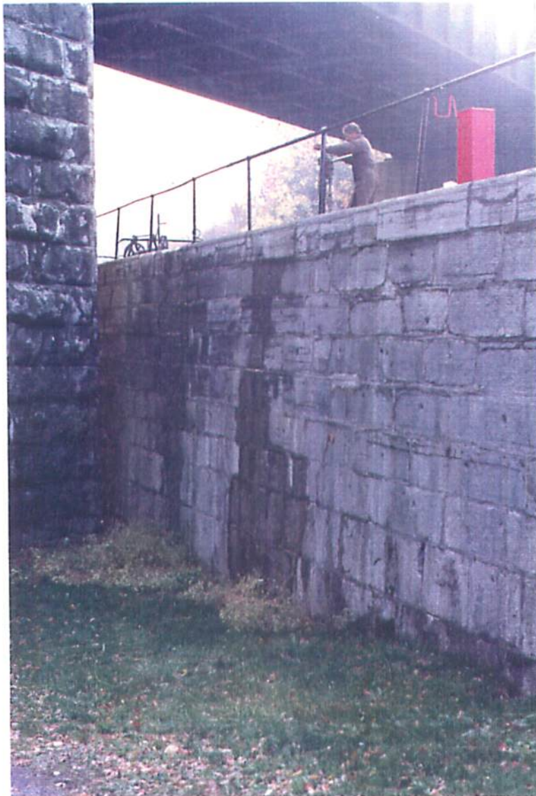
Photograph No. 6 Seepage noted in Run No. 2 - Hole V4
