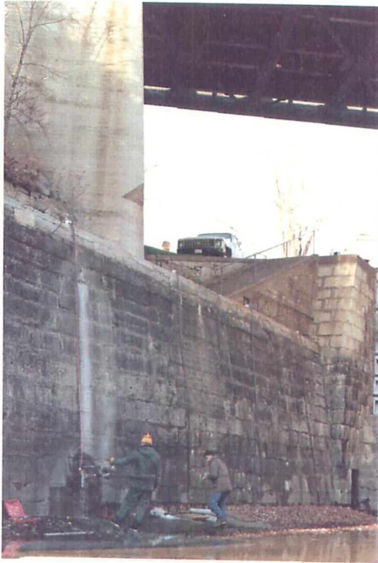
Lock 48 - West Wall Drilling Test Hole H - 7 With H - 6 Above Note Bulge In Centre Of Photograph
