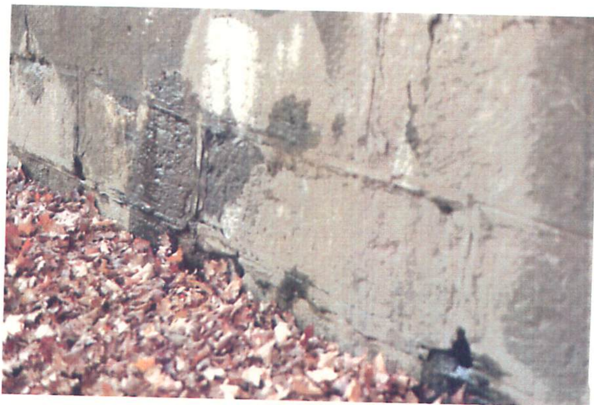
Lock 48 - West Wall Near Test Hole V - 3 Showing Seepage Prior To Grouting
