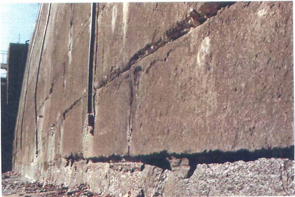
Lock 48 - West Wall Looking South Showing Open Joints and Block Movement In Foreground Note Bulge & Water Draining From Test Hole H - 7 In Background
