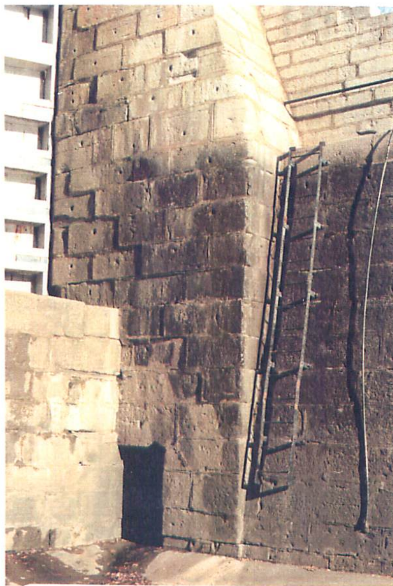
Lock 48 - East Wall Upstream Abutment Note Movement Of Masonry Blocks Due To Freeze/Thaw Action
