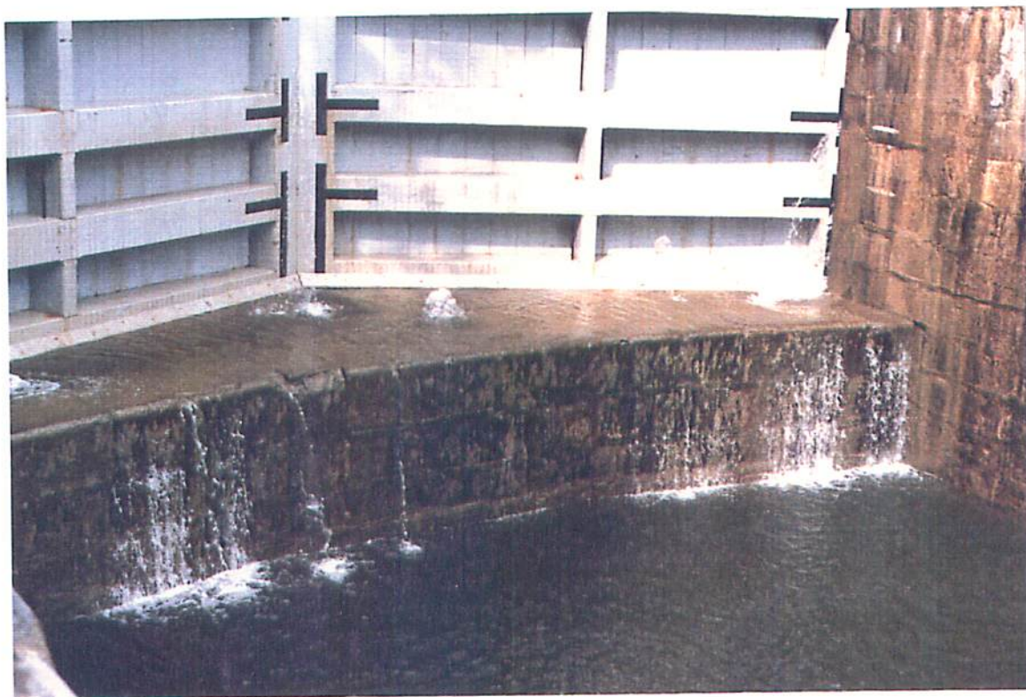
Lock 47 - Upstream Sill Note Water Boils On Top Of Sill
