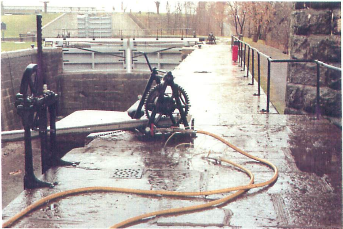
Lock 47 - East Wall Downstream Abutment Grouting Manifold At Test Hole V - 5
