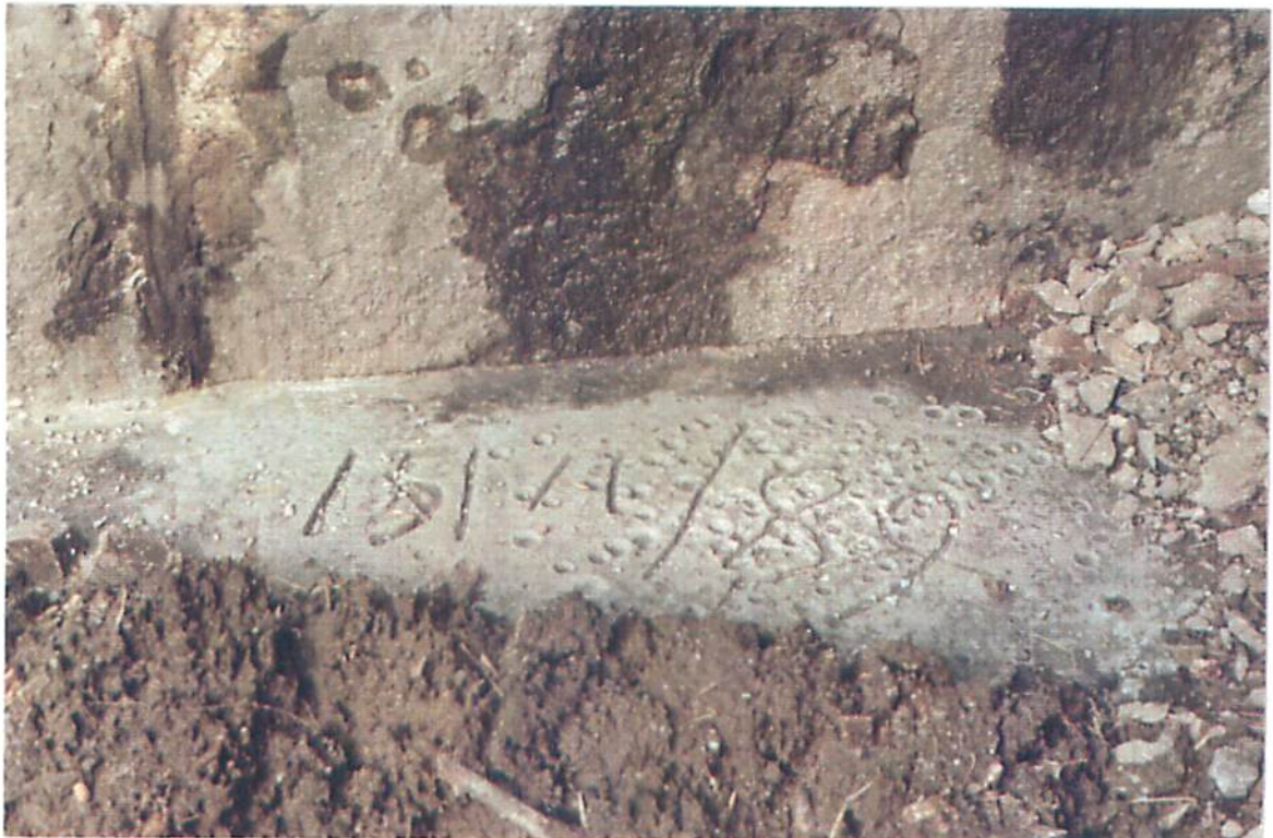
Lock 48 - Exterior East Wall Upstream Abutment Showing Grout From Test Hole H - 15 (125 mm Below Surface)
