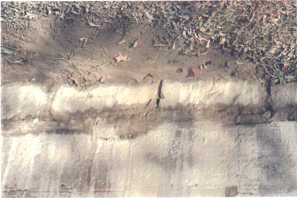
Lock 48 - Exterior East Wall Downstream Abutment Successful Plugging Of Leaks By Grouting At Test Hole H - 20
