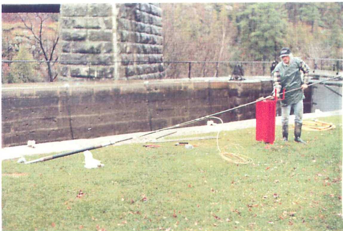
Single Inflatable Packer Assembly Showing Inflatable Packer (At Left) & Grout Pipe (Black) With Inflation Tube (White) Taped To Grout Pipe
