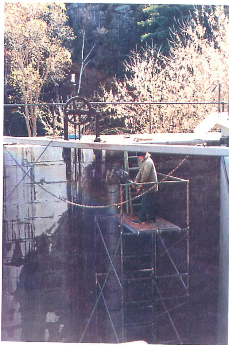
Photograph No. 9 Coring of Hole No. H 18
