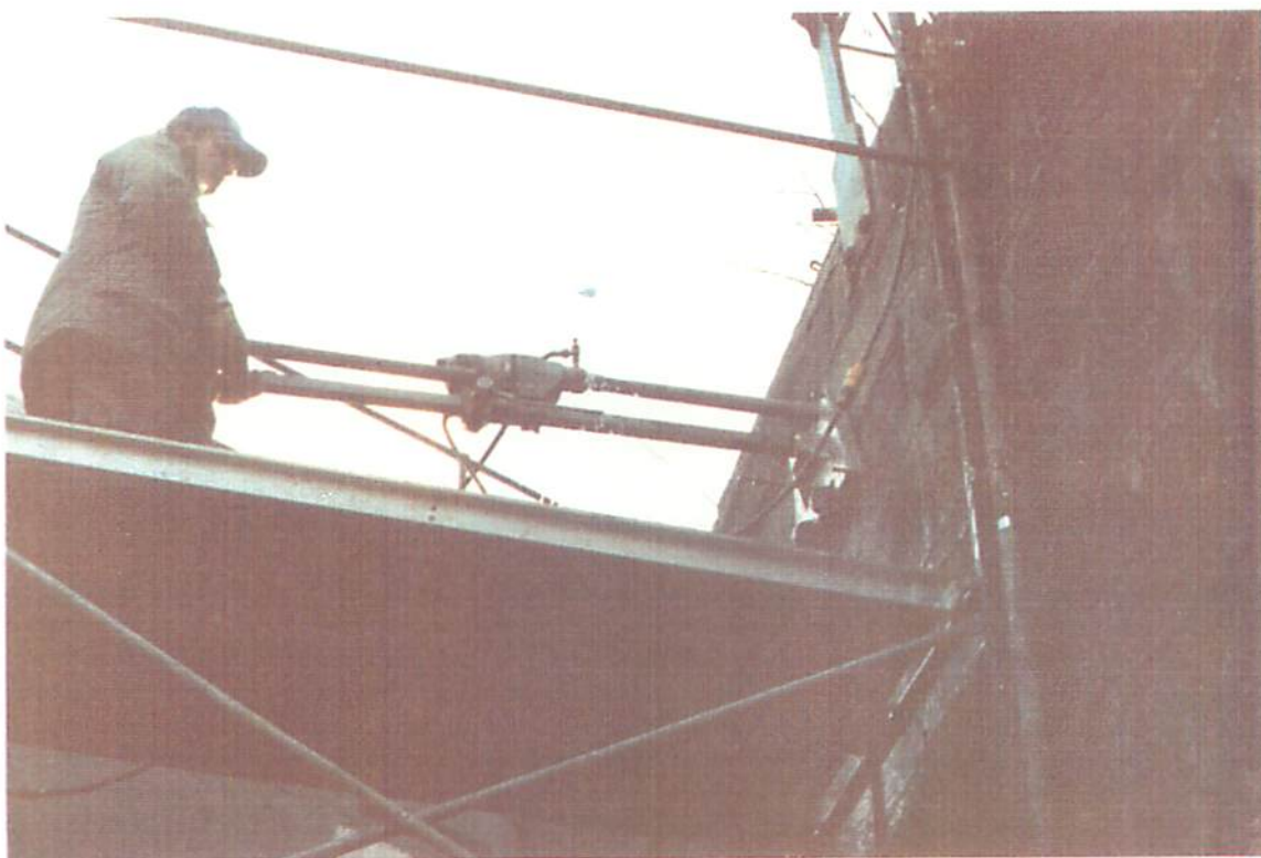
Lock 48 - West Wall Downstream Abutment Drilling Test Hole H - 8
