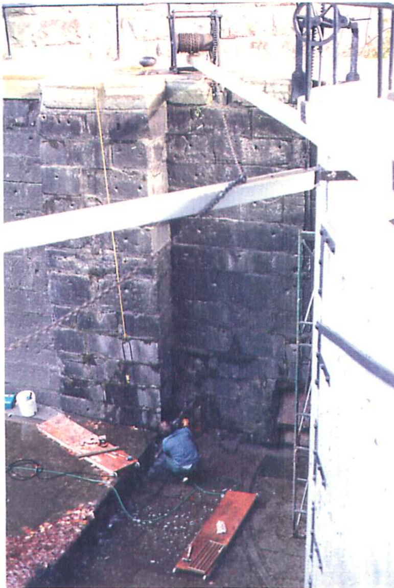
Photograph No. 10 Coring of Hole No. H15
