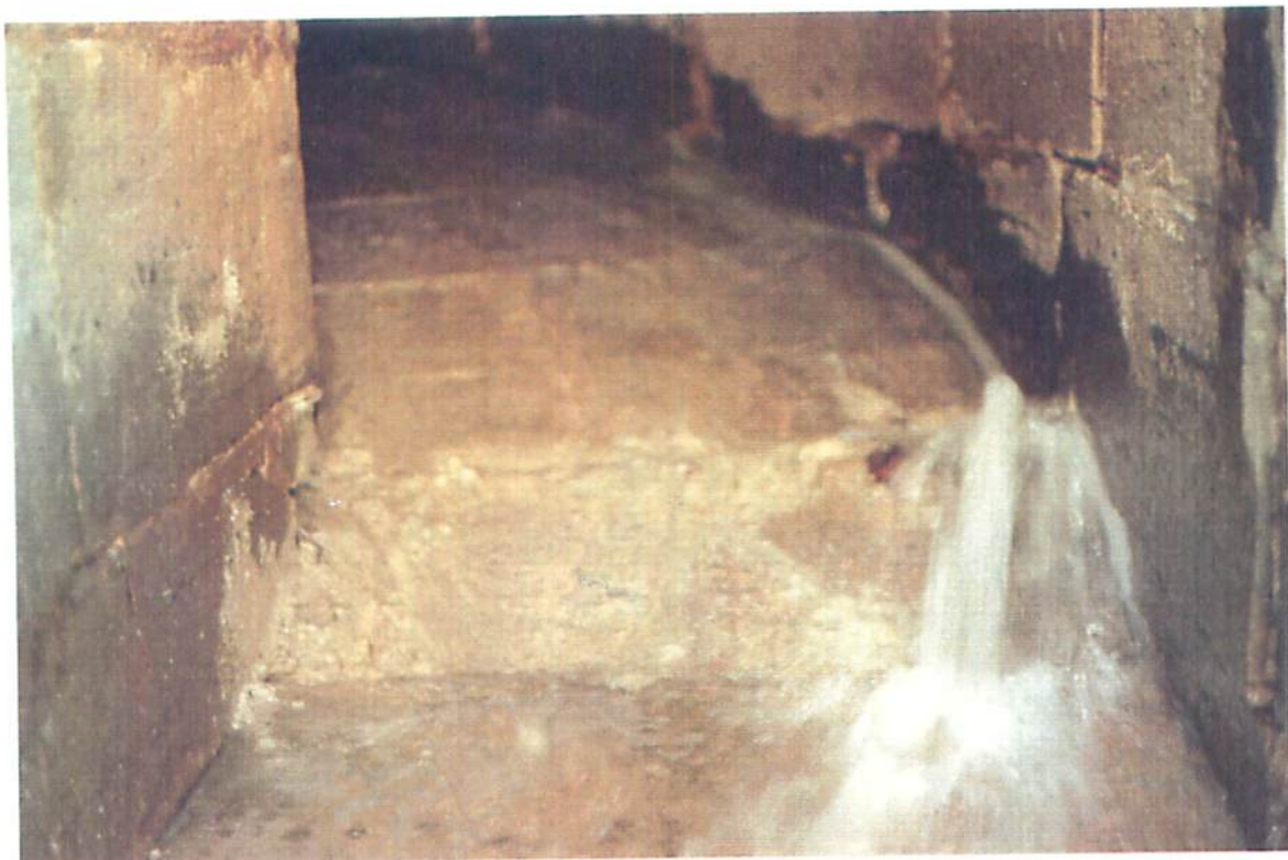
Lock 48 - Flood Gate In East Wall Upstream Abutment Note Open Joints Between Masonry Blocks
