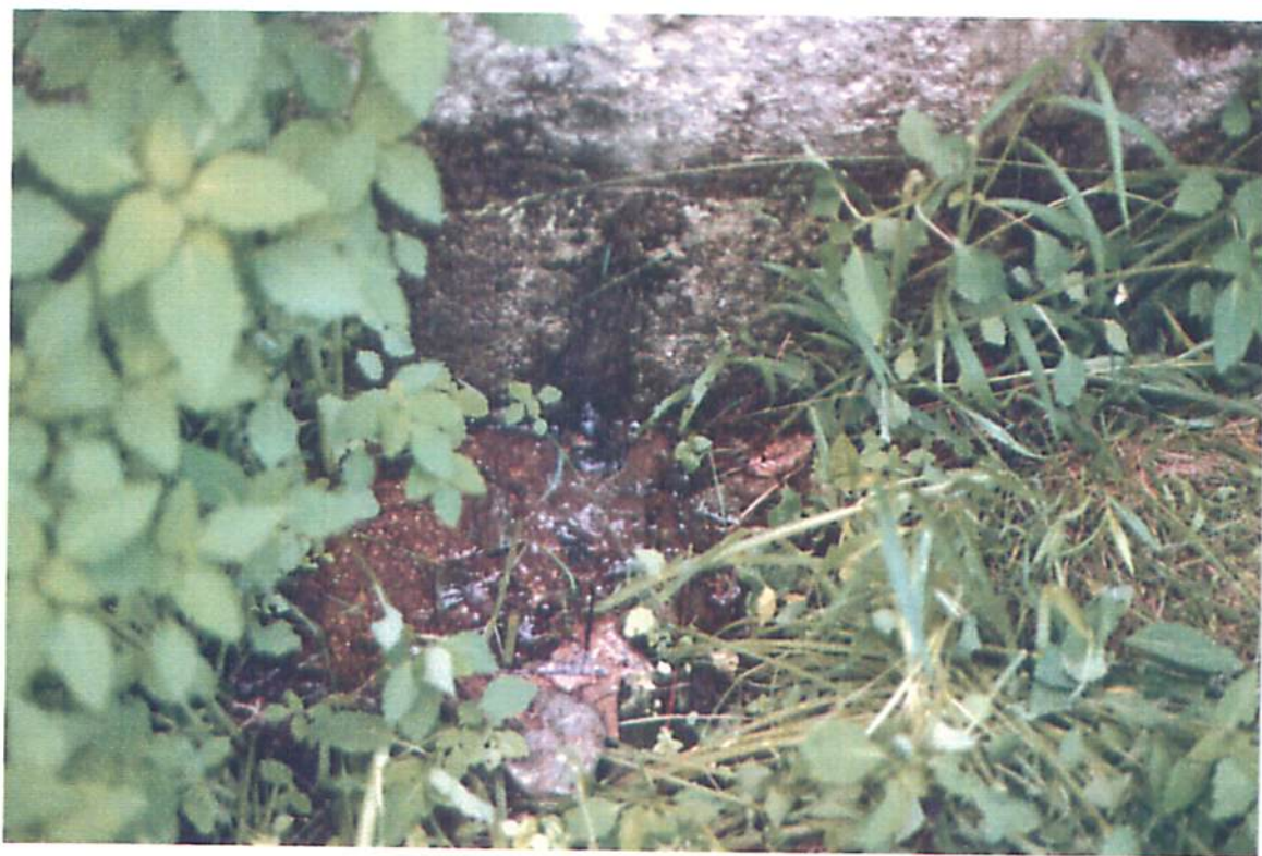
Lock 47 East Wall - External Seepage Note Water Bubbling Up From Below Surface
