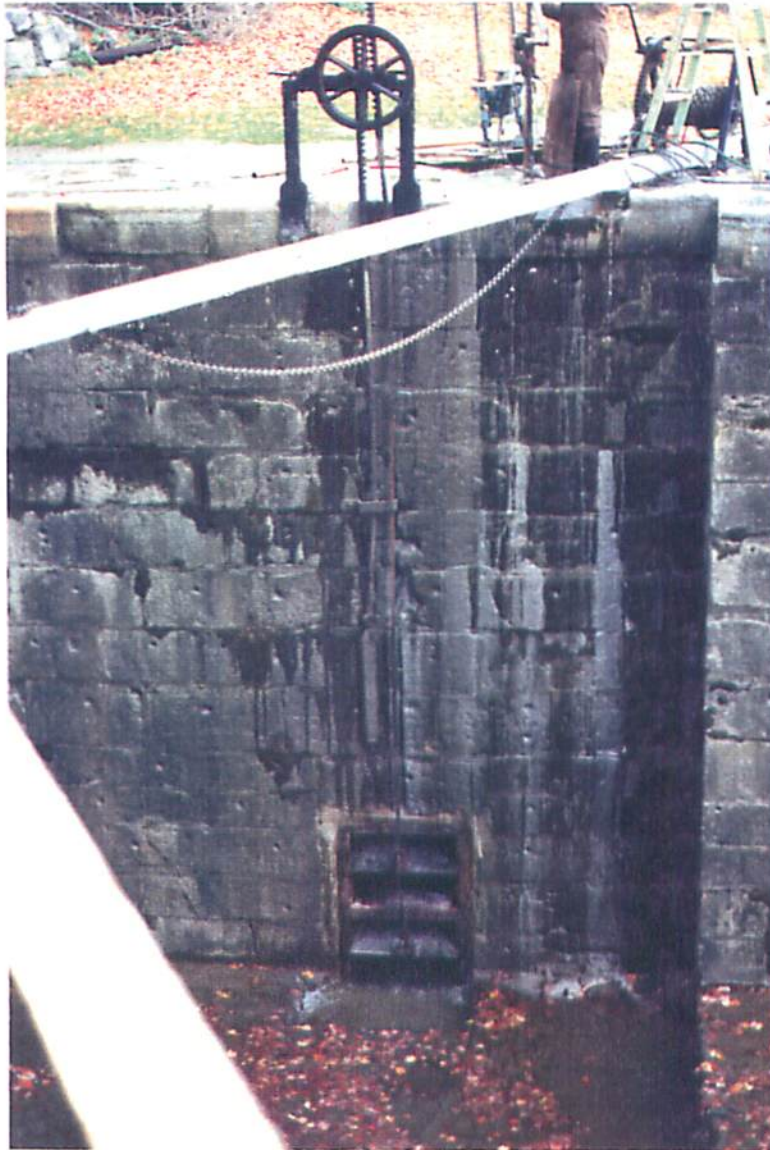
Photograph No. 3 Seepage noted in Run No. 17 - Hole V2
