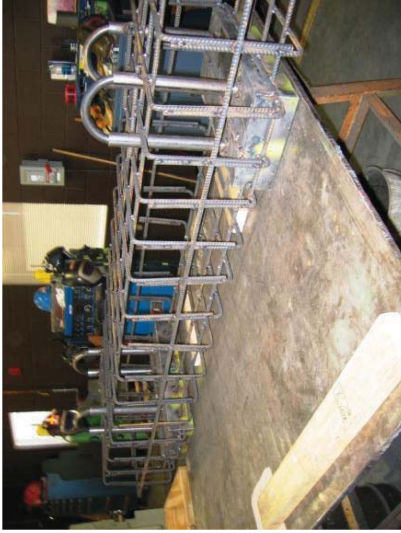
Detail Photo of Reinforcing Bar Assembly
