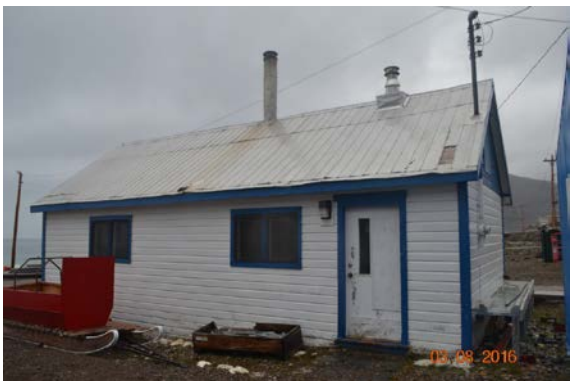
V122 workshop, missing roofing, Repair flashing on roof around new chimney
