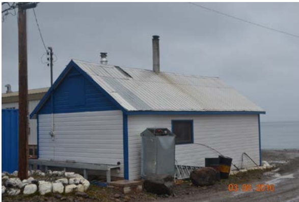
V122 workshop, missing roofing, Repair flashing on roof around new chimney
