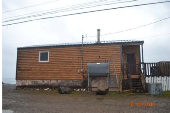
V008 house, chimney requires supports/tie downs.
