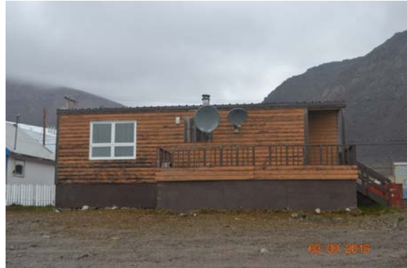
V008 house, chimney requires supports/tie downs.
