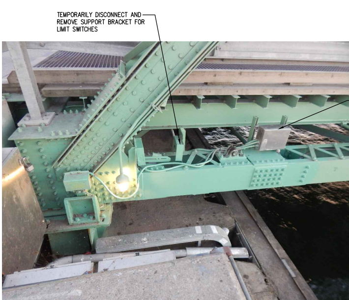
TEMPORARILY DISCONNECT AND REMOVE SUPPORT ELECTRICAL BOX
