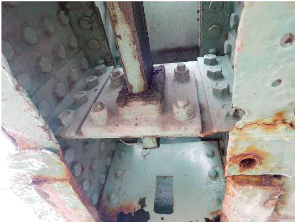
LOOKING UPWARDS AT LOCK BAR GUIDE SHOWN IN SECTION C-C, DWG. S-10
