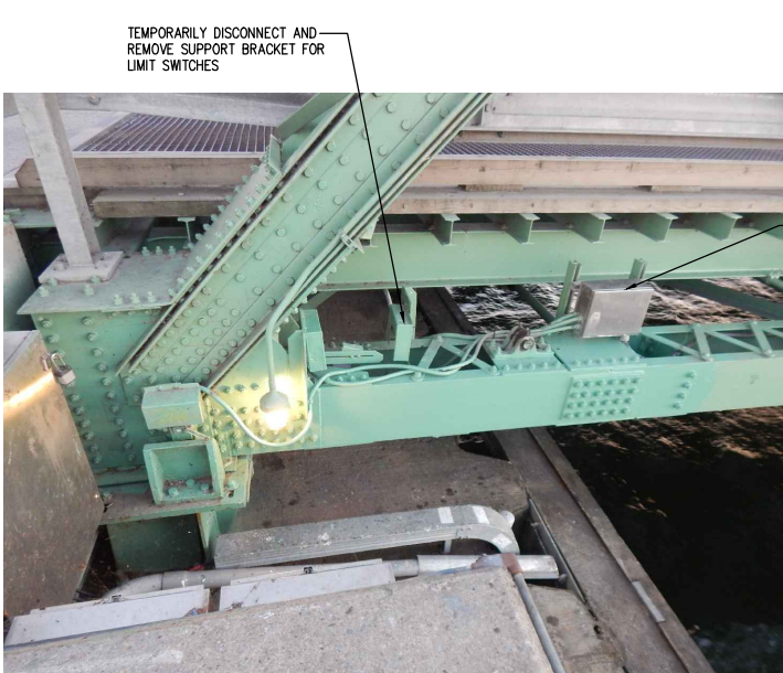
PARTIAL ELEVATION VIEW OF EXISTING NORTH BOTTOM CHORD (EXTERIOR) (SOUTHSIDE)
