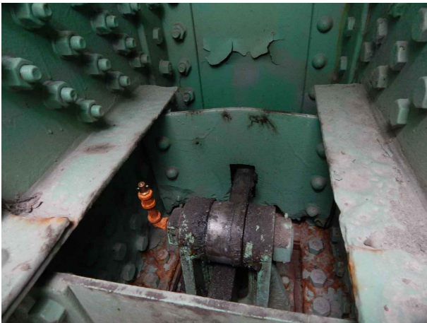
LOOKING DOWN AT TRANSVERSE STIFFENER INSIDE BOTTOM CHORD STIFFENER AT TOP SHOWN IN SECTION B-B, DWG. S-10
