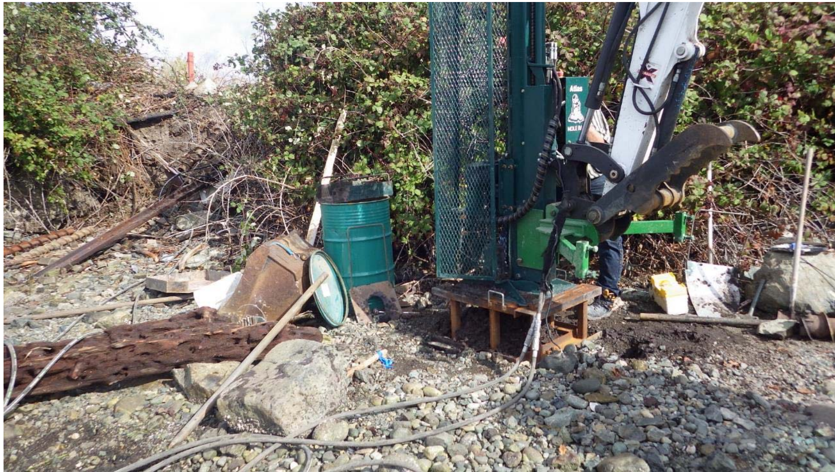
Photograph 4: Setting up the excavator-mounted auger rig for BH15-12.
