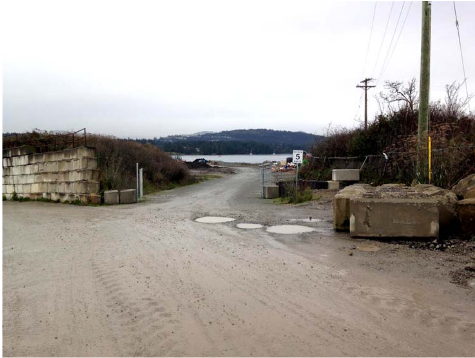
Photo 5: A view of the exit of the Trio Ready-Mix yard and the road to the site, looking west.
