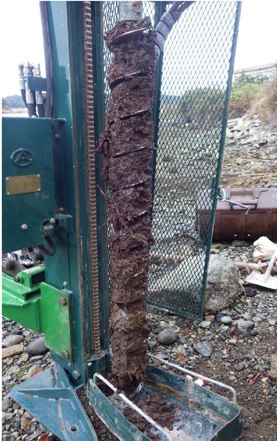
Photograph 6: Surficial fill material on auger flight prior to collection of a bulk sample.
