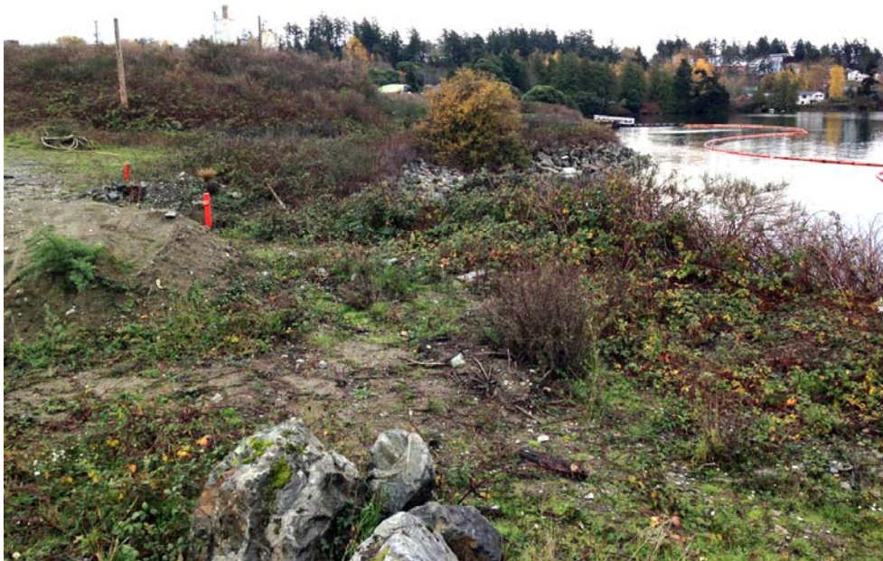
Photo 6: A view of the site from the western side, looking east.
