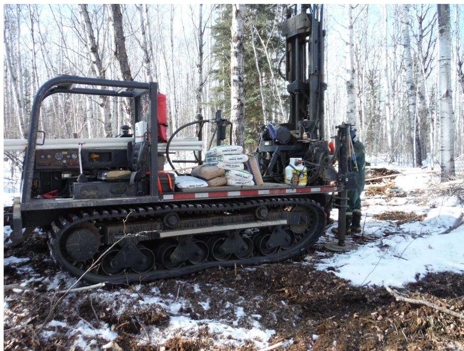
Photo 4: View of drill rig during borehole drilling and monitoring well installation program at landfill (March 2014).
