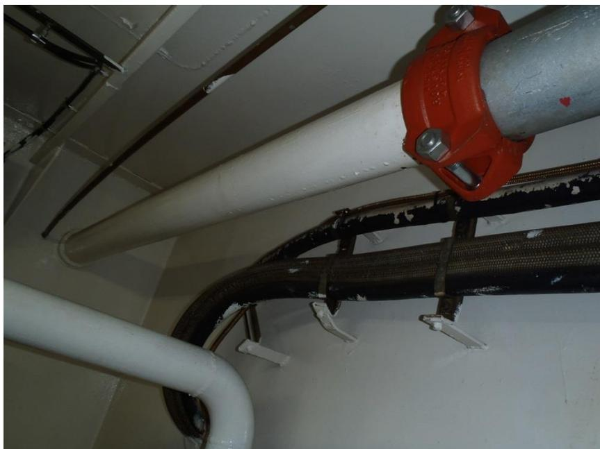
**Sewage vent pipe extending from roust about to port sewage Compartment bulkhead**
