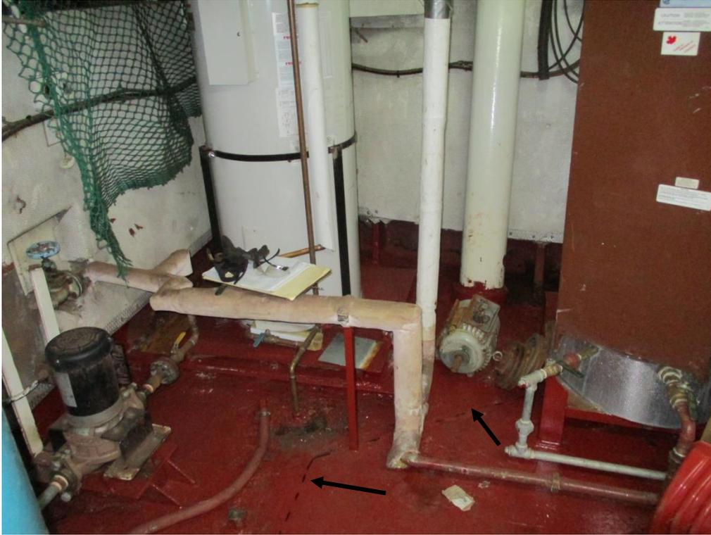
Photograph #7: General view of Aux. Machinery Room - Note interference items. Arrows indicate cut lines
