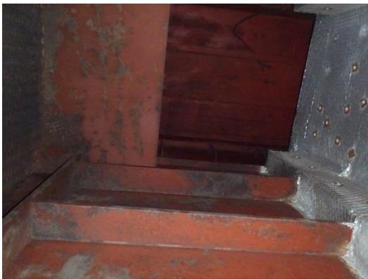
Inside of plenum showing insulation on top and screen on bottom.
