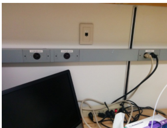
E-Figure 17 Power Bars Being Used Where Insufficient Receptacles Of The Required Type
