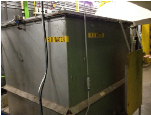
M-Figure 7 RO tank
