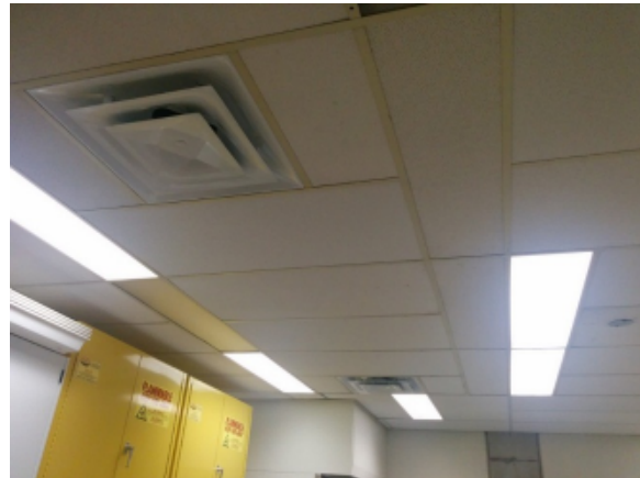
E-Figure 12 Recessed Lab Lighting, Inconsistent Light Levels
