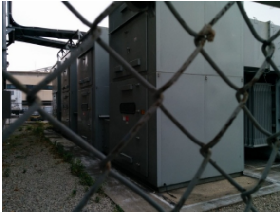
E-Figure 1 Incoming 27.6kV Switchgear
