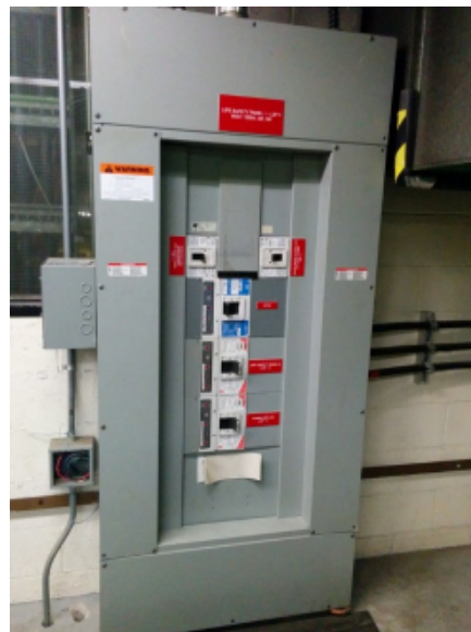
E-Figure 7 Main Life Safety Panel
