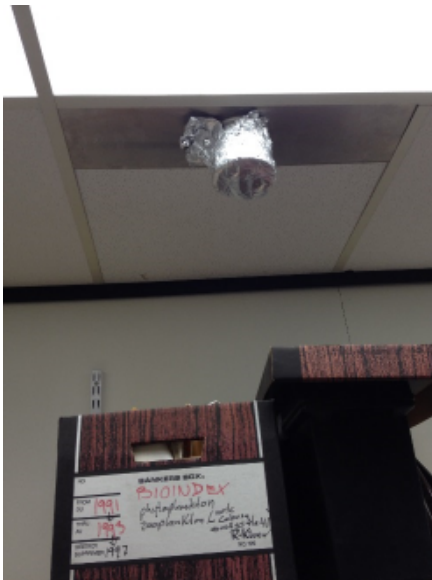
M-Figure 41 Poorly capped snorkel rough-in
