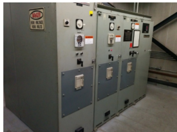
E-Figure 4 5kV Switchboard, Aging
