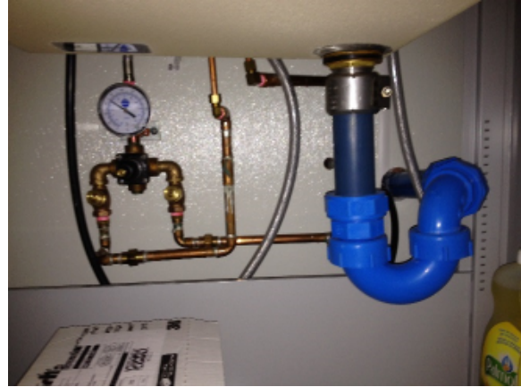
M-Figure 2 Plastic pipe serving laboratory sink
