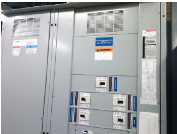
E-Figure 6 Main Critical Power Panel, New
