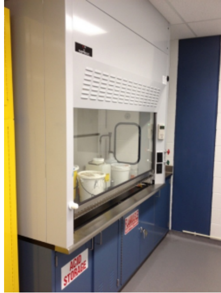
A-Figure 37 New Fume Hood
