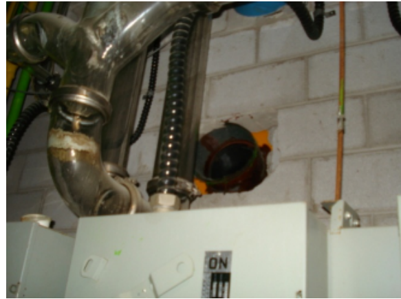
A-Figure 50 Service Core penetration without fire stopping
