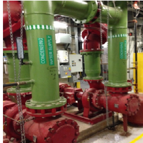
M-Figure 26 Condensing water pumps
