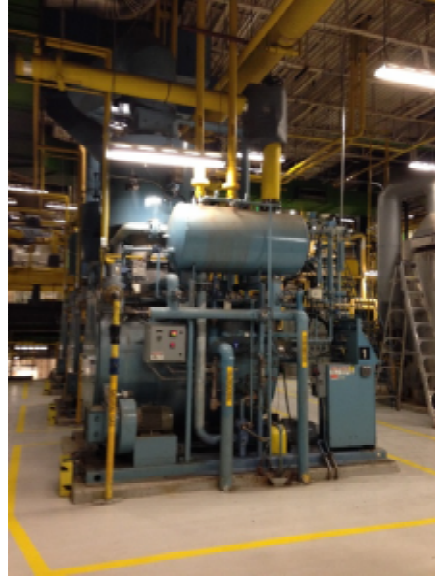
M-Figure 21 Steam boiler
