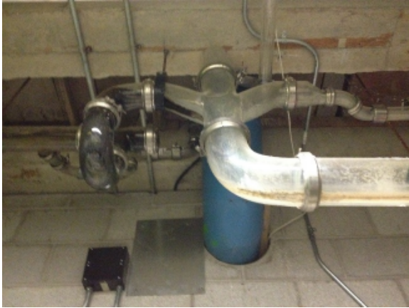
M-Figure 1 Acid resistant piping
