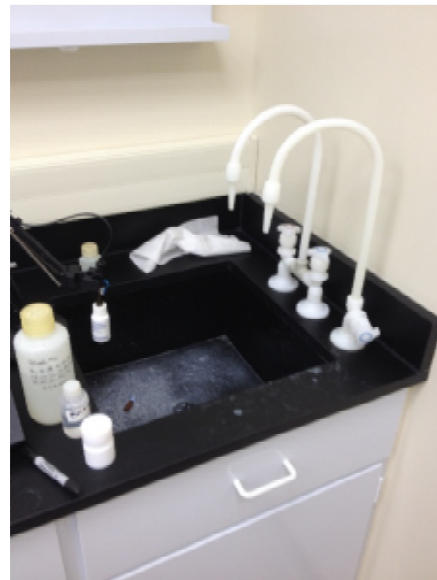
M-Figure 18 Polypropylene faucet (renovated lab)
