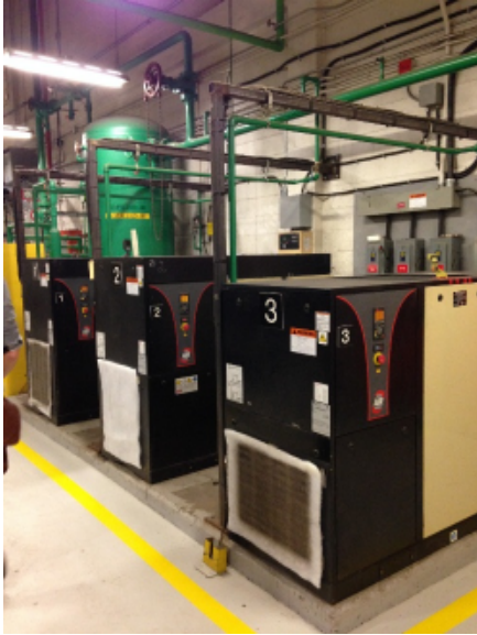
M-Figure 9 Air compressors and receiver
