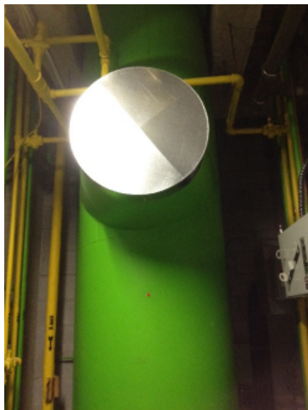
M-Figure 29 Systems 29 and 30 capped make up air duct distribution to exhaust hoods
