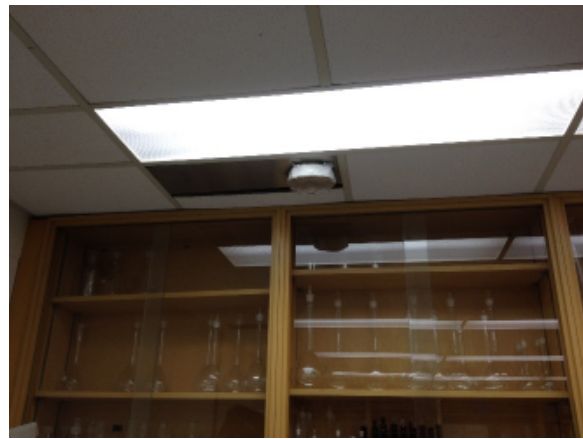
M-Figure 40 Snorkel rough-in uncapped
