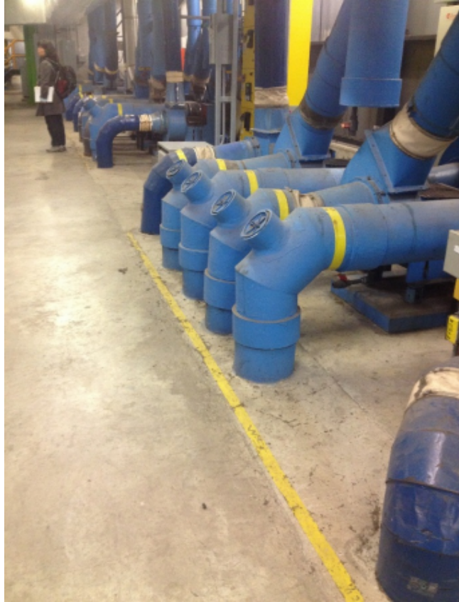
S-Figure 3. Pipe penetrations above the service corridors at the Mechanical Penthouse level
