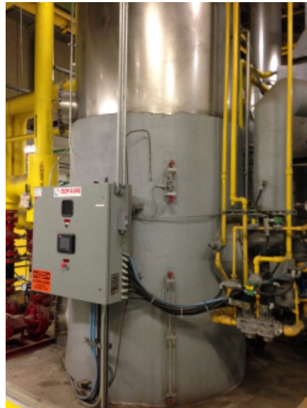
M-Figure 23 Direct contact hot water heating boiler (Sofame)
