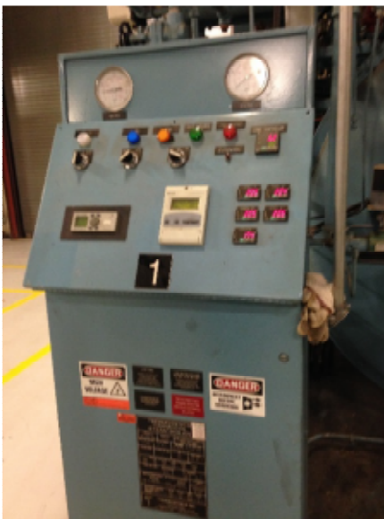
M-Figure 22 Steam boiler operator's station
