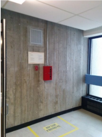
E-Figure 18 Pull station and Firefighters Handset at Stairwell Entrances
