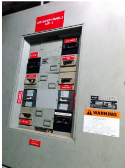
E-Figure 8 Example of Aging Emergency Distribution Equipment
