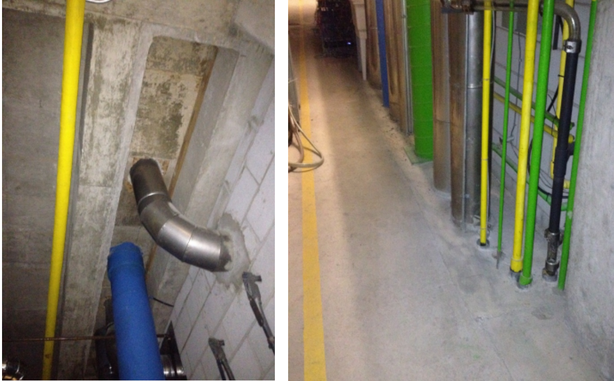
S-Figure 1. Typical low strength concrete slabs within the service corridors accommodating Pipe penetrations above (shown on the left) and below each level (shown on the right)
