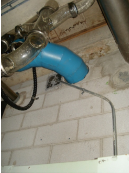
A-Figure 49 Service Core penetration without fire stopping
