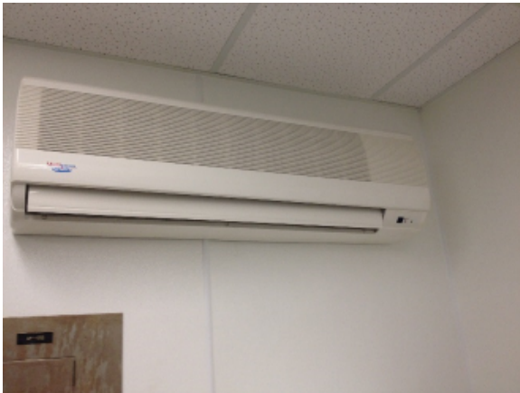
M-Figure 37 Split air conditioning indoor unit
