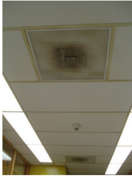
A-Figure 18 Typical Lab acoustic tile ceiling in poor condition
