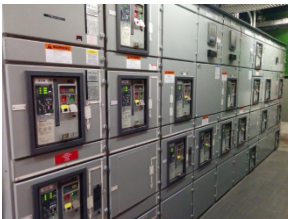
E-Figure 3 Main 600V Twin Switchboard
