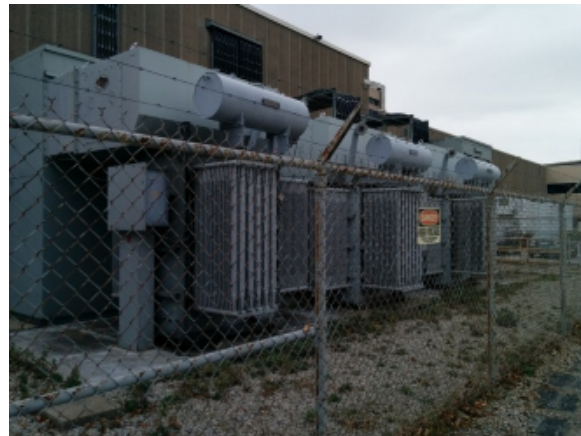
E-Figure 2 Outdoor Service Transformers
