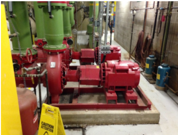
M-Figure 27 Condensing water pumps
