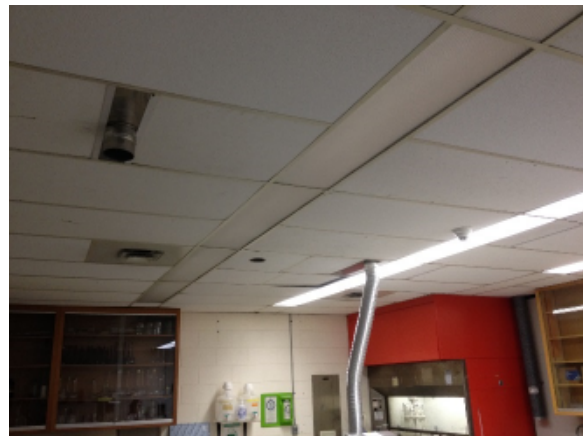
M-Figure 42 Poorly capped snorkel rough-in
