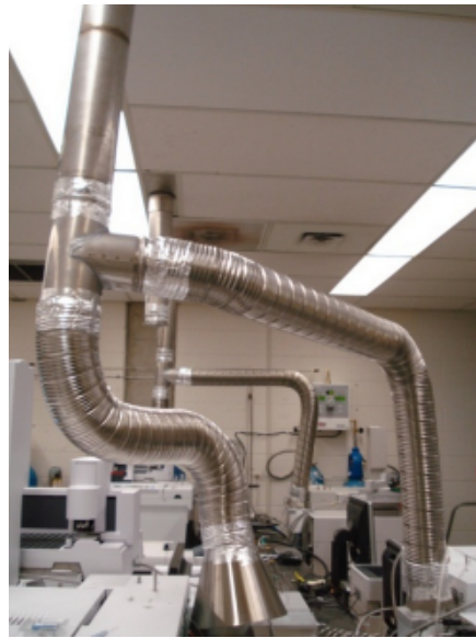
A-Figure 39 Gooseneck Fume Hood
