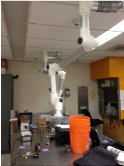
M-Figure 39 Laboratory snorkel
