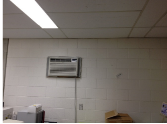
M-Figure 36 Packaged air conditioning unit
