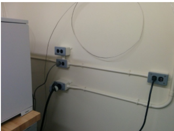
E-Figure 16 Surface Mounted Conduit
