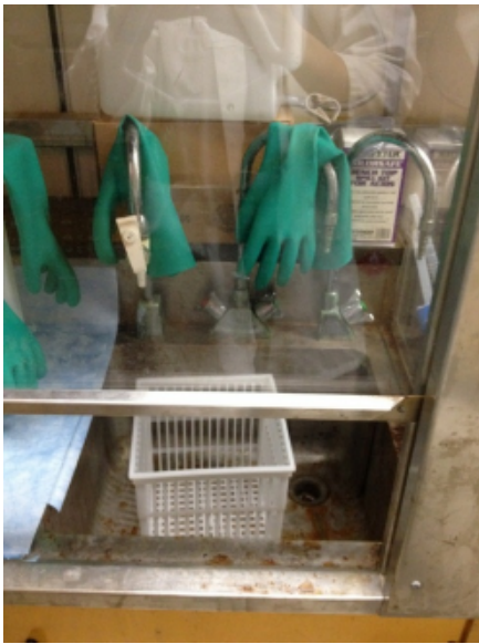
A-Figure 38 Corroded sink in acid contamination unit
