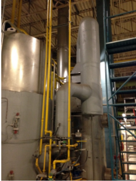
M-Figure 24 Direct contact hot water heating boiler (Sofame)
