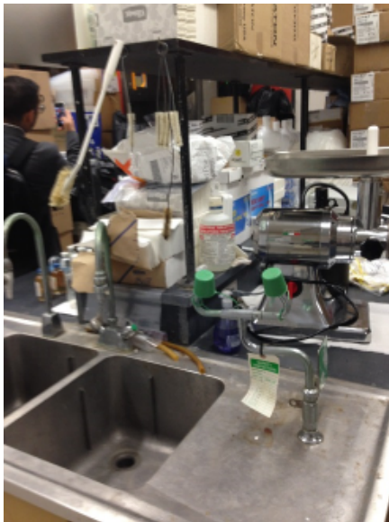
M-Figure 17 Laboratory stainless steel sink and eye wash in poor condition
