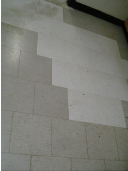
A-Figure 21 12"x12" Vinyl composite tile with new patches
