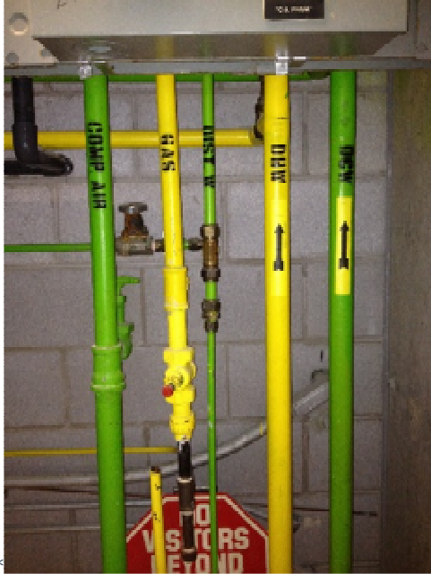
* M-Figure 5 Typical plumbing risers
