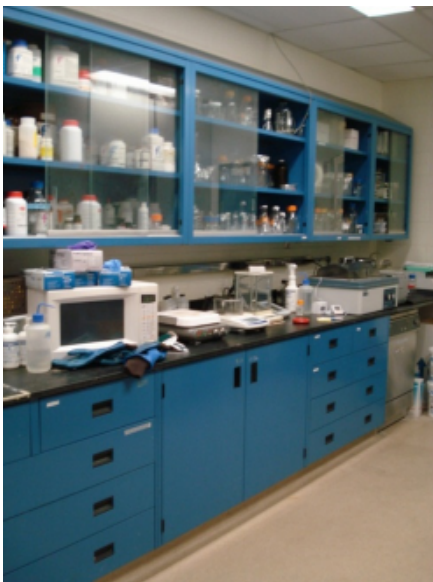
A-Figure 34 New Metal and Laminate Millwork
