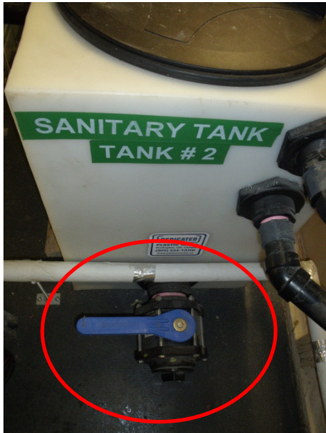
Sewage transfer tank drain
