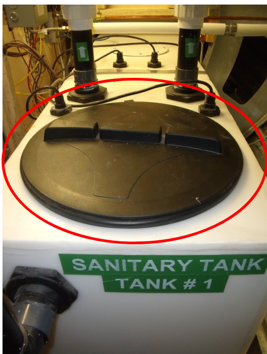
Top hatch of sewage holding tank
