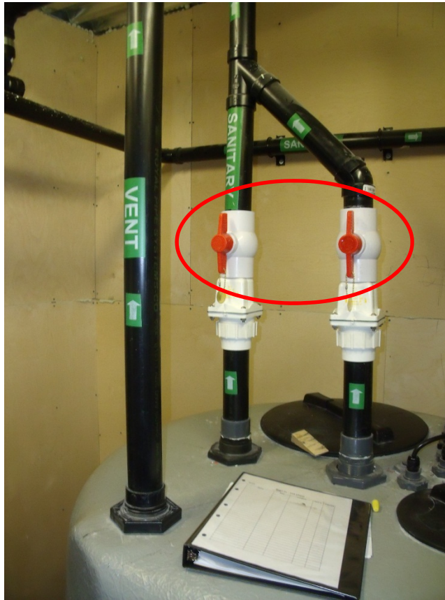
Valves on the sewage line shown in the open position
