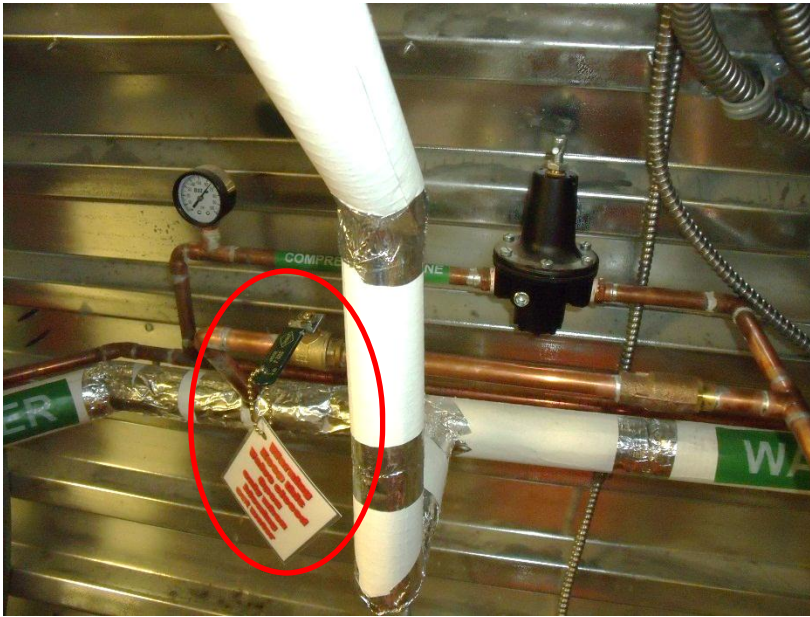
Air line valve connecting air line to water line
