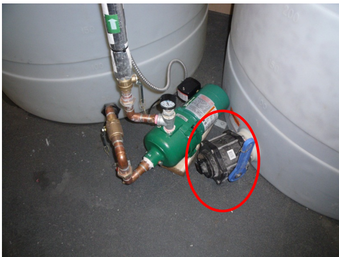
Sewage storage tank drain valve and drain
