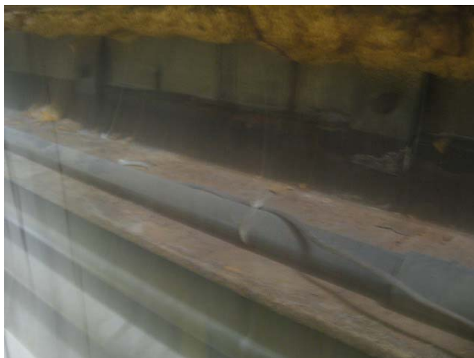
AR-039 – Water and rusting metal structure from active leak in Boiler Plant north wall (upper level).
