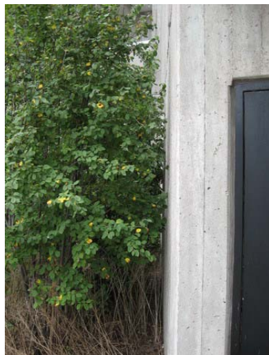
AR-073 – Proximity of vegetation to building face restricts air flow and holds moisture in building envelope.
