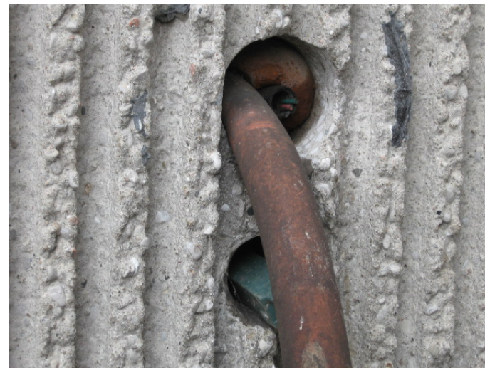
AR-008 – Unsealed wall penetrations.
