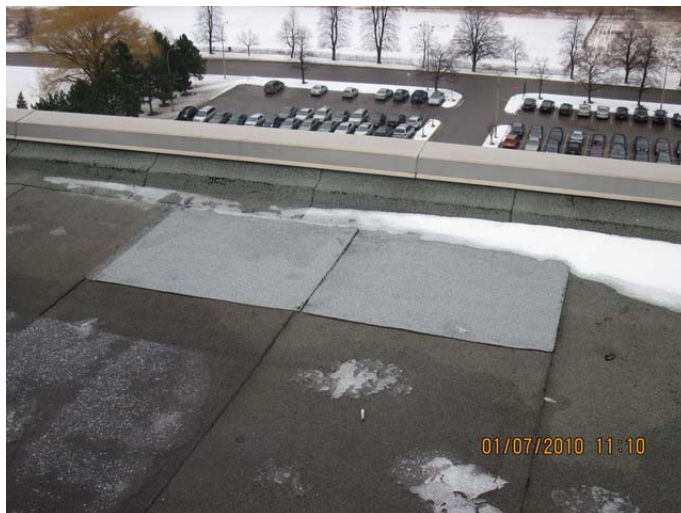
AR-065 – Recently repaired/patched area at SBS membrane roofing.
