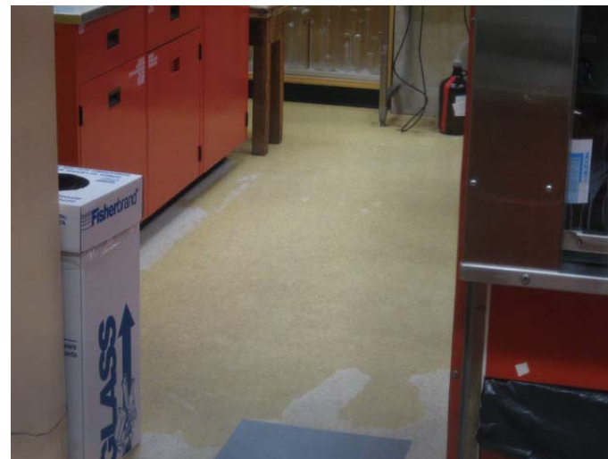
AR-096 – Vinyl sheet flooring standing-up poorly at this particular lab – surfaces badly stained and degraded.
