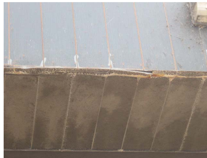
AR-038 – Deteriorated paint finish and damaged components at overhead door canopy siding/soffit.
