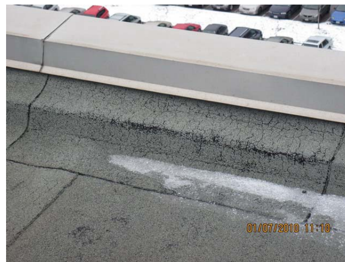
AR-064 – Cracking of membrane and loss of granular material at SBS membrane roof flashing.
