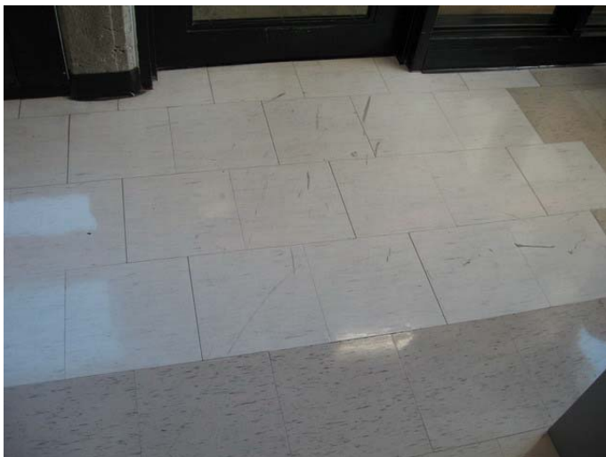
AR-093 – Newer vinyl tile not holding-up as well as older tile.
