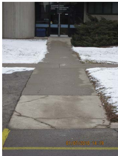
AR-087 – Cracked/broken concrete at walkway curb ramp.
