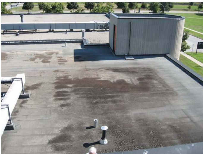
AR-039 – Staining and sediment build-up indicating standing water areas throughout SBS roof.
