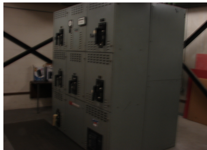
ELE-004 – Typical main 600 V electrical distribution switchboard.
