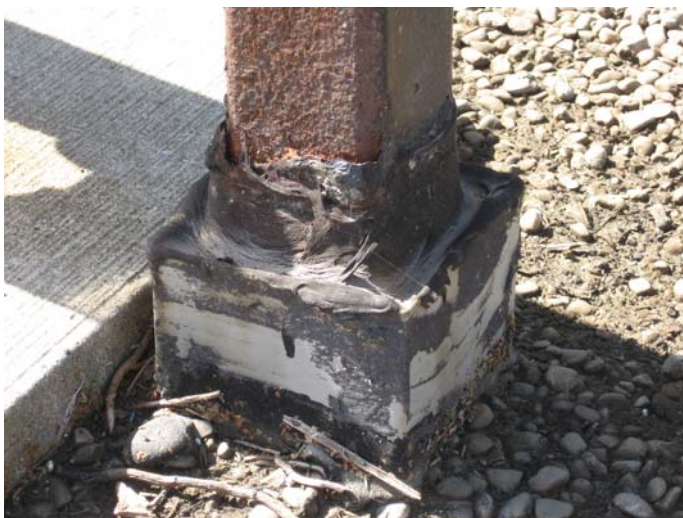
AR-043 – Deteriorated filler in equipment support frame pitch pockets.
