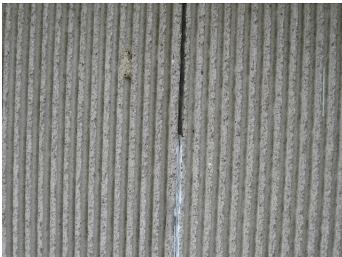
AR-021 – Missing sealant at precast concrete panel joints.
