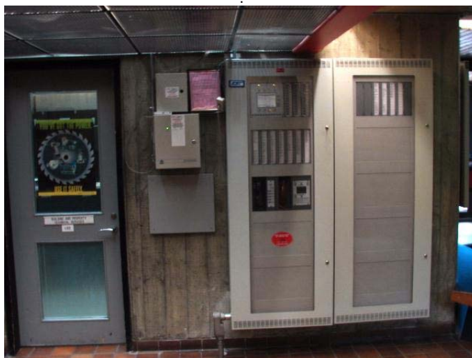
ELE-039 – Main fire alarm panel.
