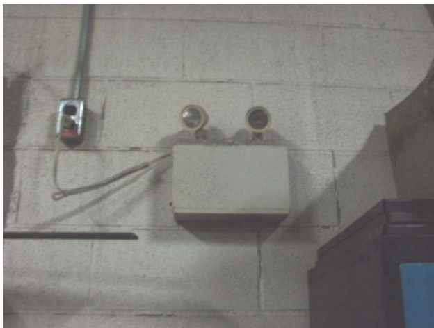
ELE-033 – Typical emergency battery pack.
