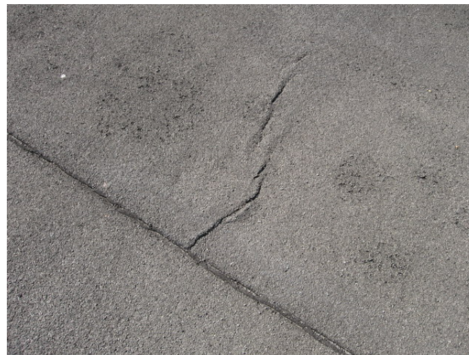
AR-050 – Fracture of SBS membrane.
