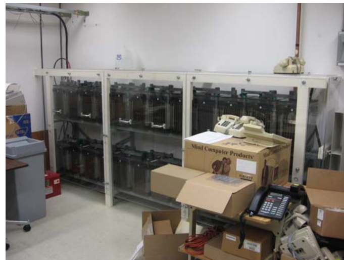
ELE-050 – Main telephone battery rack.
