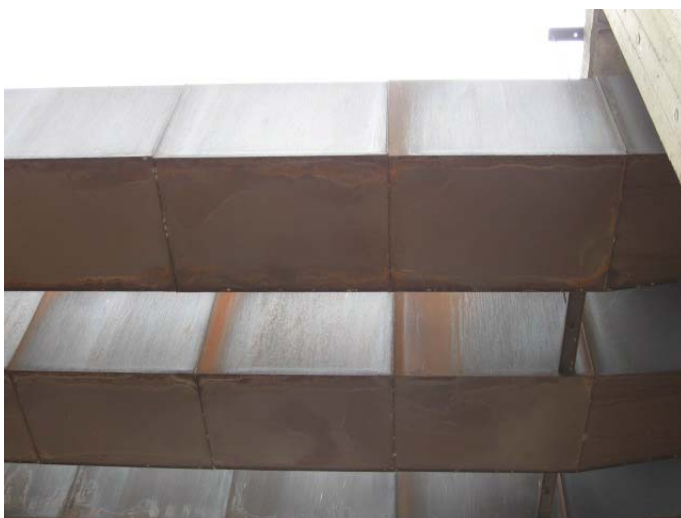
AR-019 – Underside of rusting metal breechings at Boiler Plant.
