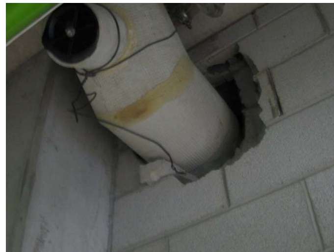
AR-118 – Unsealed penetration in fire separation between lab and service core.
