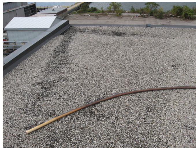
AR-022 – Areas of asphalt bleed-through and exposed bitumen at BUR.
