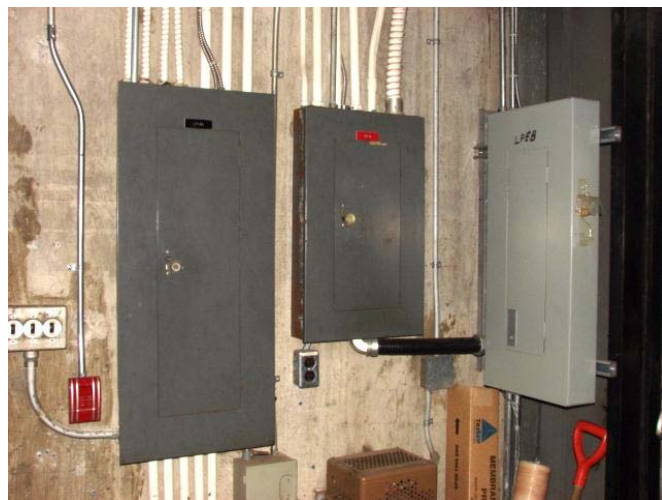
ELE-011 – Mechanical area older panelboards.
