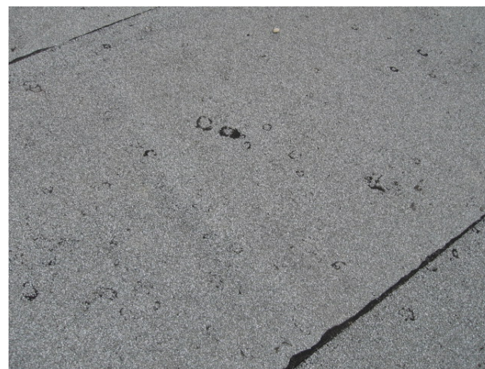
AR-020 – Damage to granular surface of SBS membrane - cause of marks unknown.
