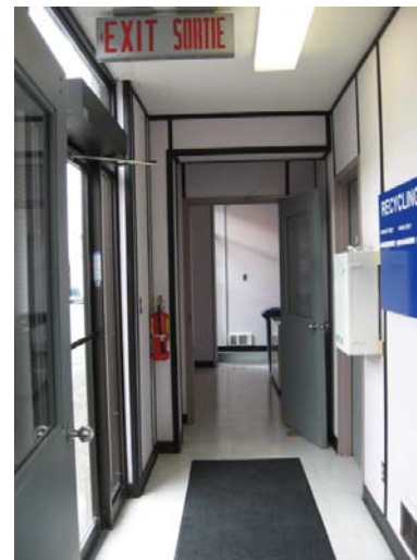
AR-026 – Fire door wedged in open position at 1st floor entrance lobby.
