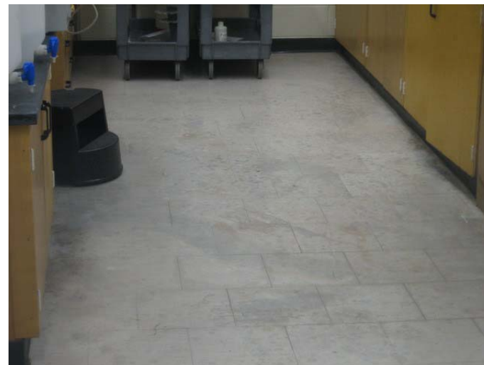
AR-092 – Vinyl tile flooring standing-up poorly at this particular lab – surfaces badly stained and degraded.
