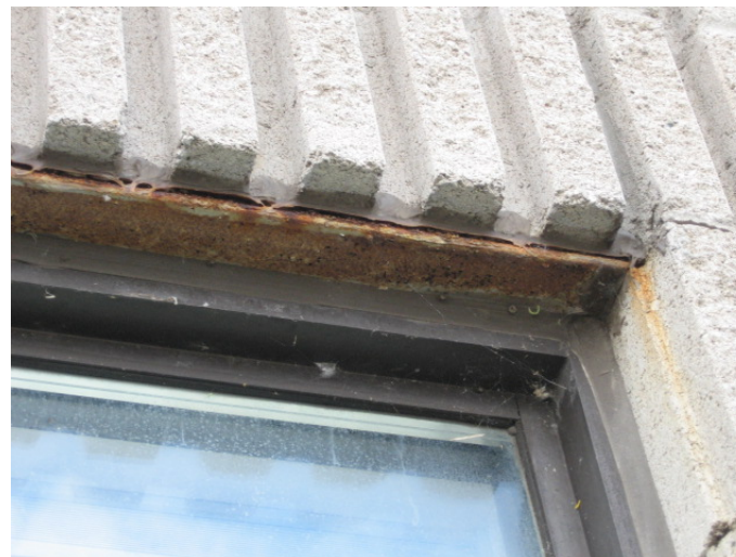
AR-014 – Rusting metal lintel at window opening.
