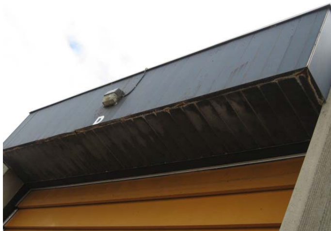
AR-037 – Deteriorated paint finish and rusting metal surfaces at Overhead door canopy siding/soffit.
