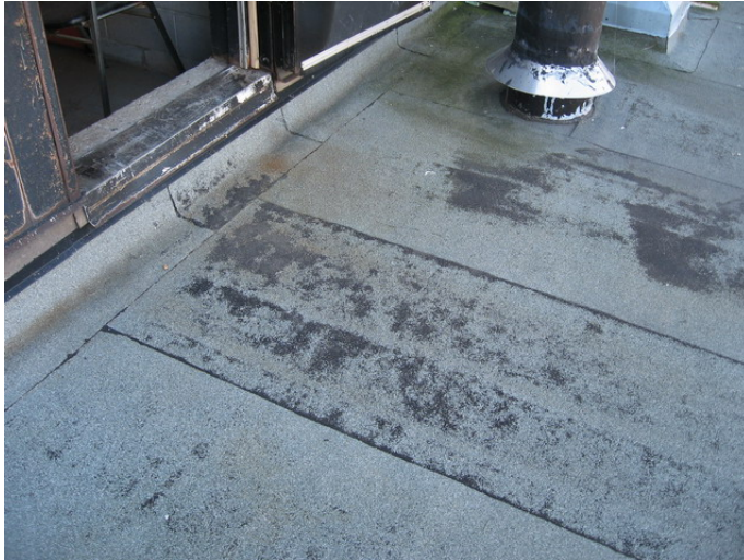
AR-053 – Loss of granular surfacing at SBS membrane roll at access door location.
