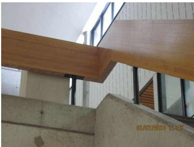
AR-115 – Guards with unprotected openings at Mall 2 nd floor.
