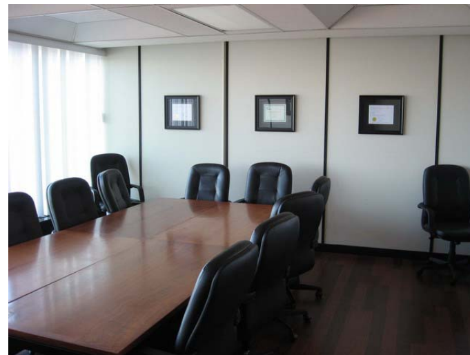
AR-108 – Conference room ceiling with part of original coffered type replaced with conventional flat type.
