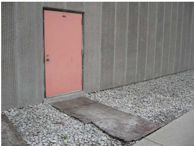
AR-089 – Plywood surfacing used at exit stair (WN) exterior door (Door 45) to compensate for uneven surface.
