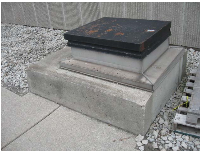
AR-021 – Tunnel access hatch cover with deteriorating paint finish.
