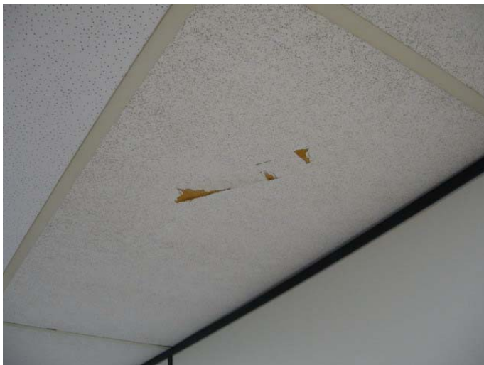
AR-103 – Acoustic ceiling tile with surface damage – cause unknown.
