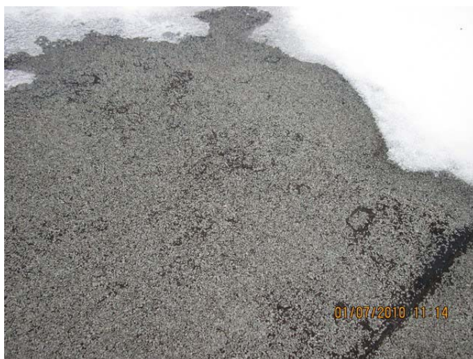
AR-067 – Blister in SBS membrane roofing.
