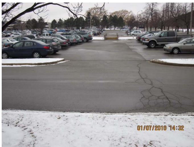
AR-083 – Cracking/alligating of asphalt pavement at driveway and throughout parking area.
