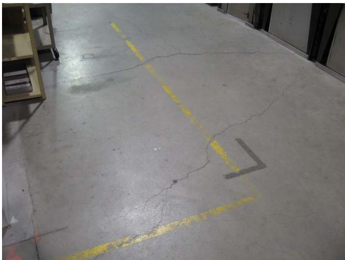
AR-017 – Cracks in concrete floor slab.
