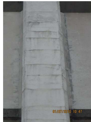
AR-034 – Cracks in cementitious coating on exposed column at A&L east elevation.
