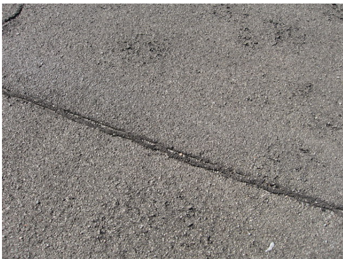
AR-051 – Asphalt bleed-out at SBS membrane roll edges.
