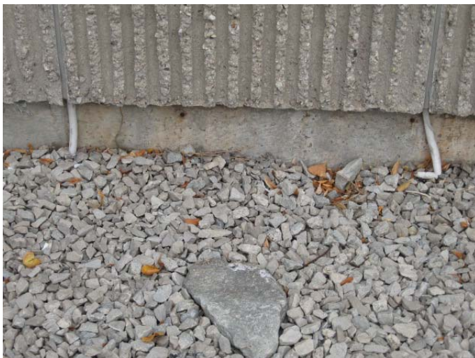
AR-029 – Undersized sealant backer rods falling out of concrete sandwich panel joints.
