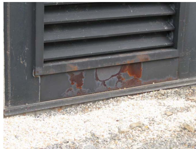
AR-032 – Deteriorated paint finish and rusting metal surfaces at Boiler Plant wall metal panel.
