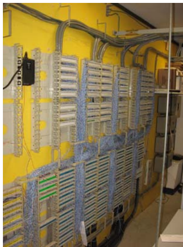
ELE-049 – Main telephone BIX board.
