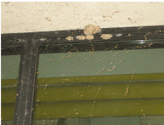
AR-019 – Dirty surfaces (nests, webs, debris, etc.) at walls and soffits.
