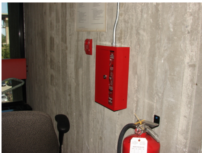
ELE-043 – Pull station and emergency voice telephone.
