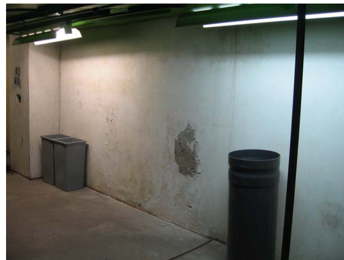
AR-044 – Moisture damaged interior finish at A&L 3 rd floor east wall.
