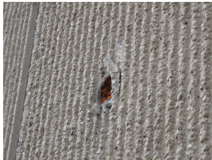
AR-014 – Sealed hole with spalling concrete at wall panel.
