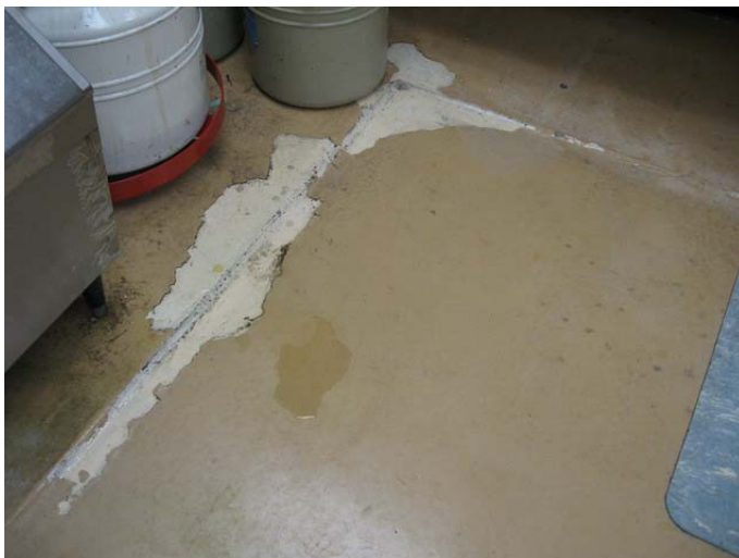
AR-097 – Epoxy flooring standing-up poorly at this particular lab – localized deterioration.
