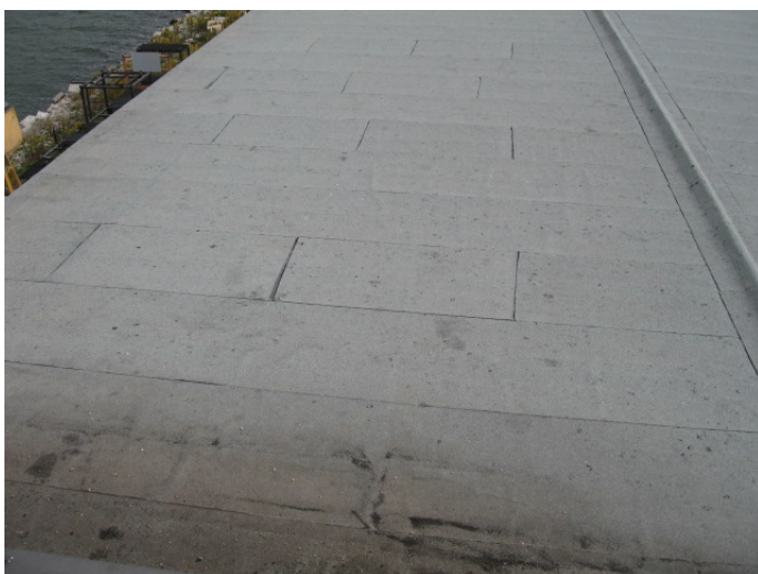
AR-019 – Roofing at northwest corner of warehouse completed with 'end cuts'.
