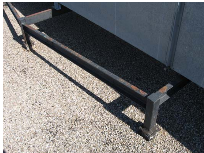
AR-042 – Deteriorating paint finish and rusting metal surfaces at equipment support frame.
