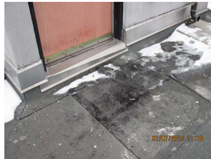
AR-066 – Severe loss of granular material at SBS membrane roofing at roof access point.
