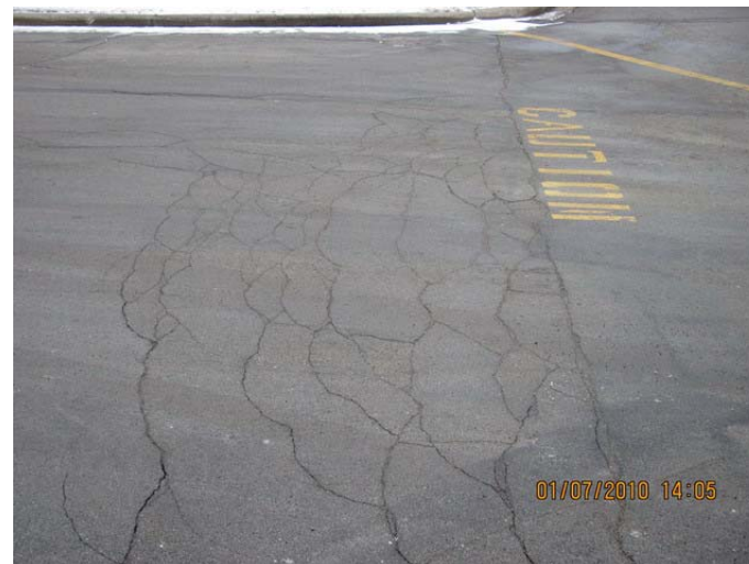
AR-082 – Cracking/alligating of asphalt pavement at driveway.
