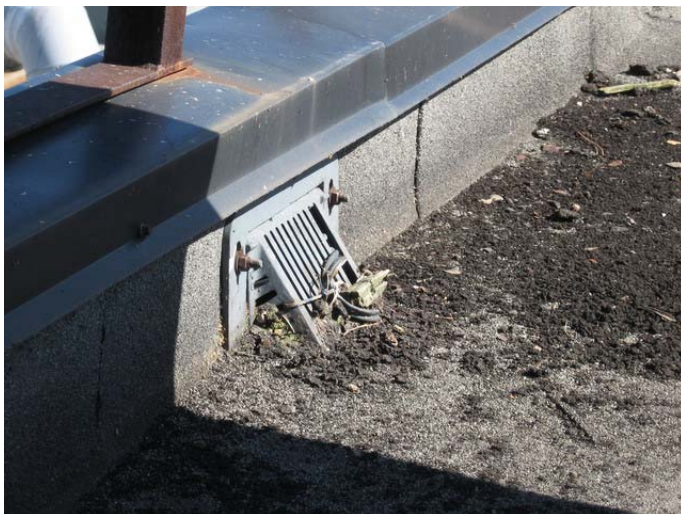
AR-033 – Broken strainer and debris/sediment build-up at stairwell roof.
