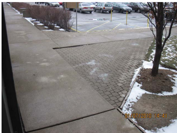
AR-077 – Settled/sunken unit pavers at Mall north entrance creating tripping hazard.
