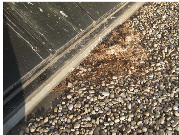
AR-060 – Debris accumulation at EPDM membrane roofing.
