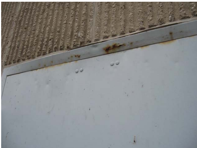
AR-055 – Deteriorated paint finish and rusting metal surfaces at door lintel.
