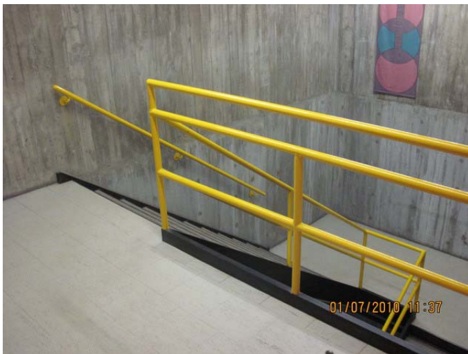
AR-117 – Exit stair guards with unprotected openings and handrails without extensions and returns.
