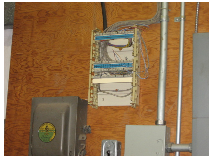
ELE-008 – Telephone communications main.
