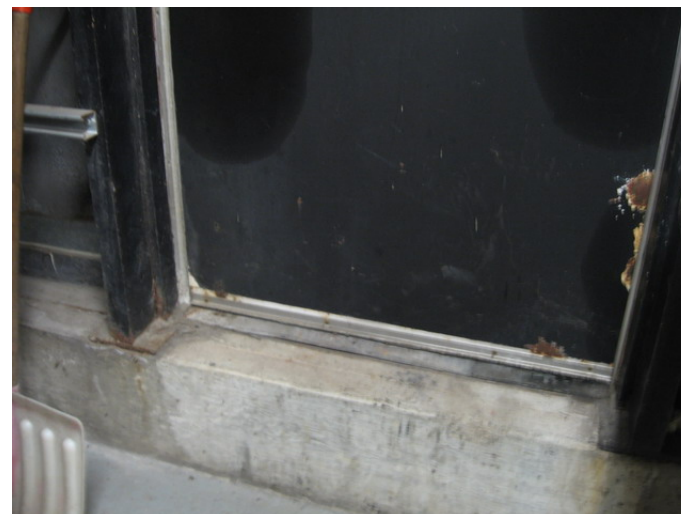
AR-064 – Deteriorating paint finish and rusting metal surfaces at PH/rooftop access door and frame.
