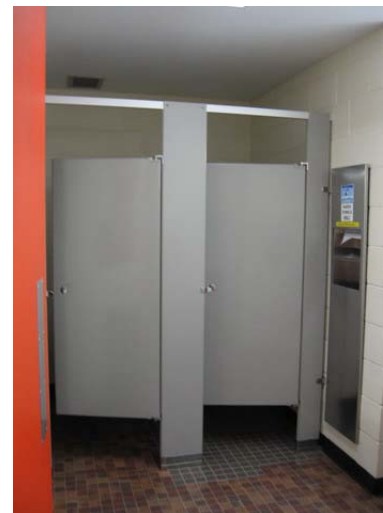
AR-098 – Mismatched ceramic floor tile at localized area replacement in washroom.
