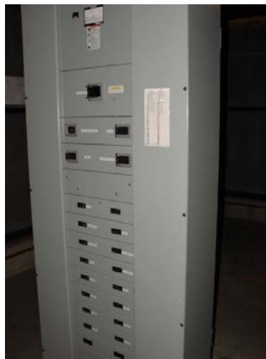
ELE-001 – Main 600V distribution for Labs and Offices.
