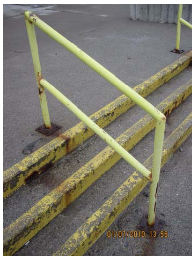
AR-079 – Deteriorated paint finish, rusting metal and stained surfaces from Guards and exposed rebar at R&D west-centre entrance stair.
