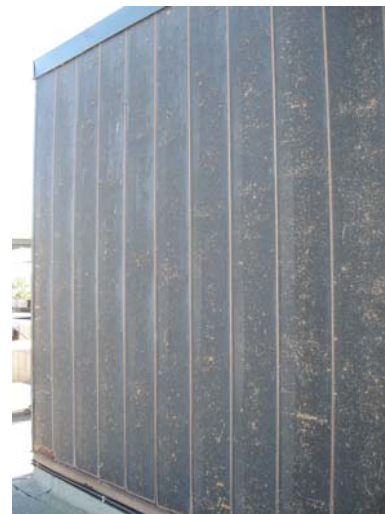
AR-030 – Deteriorating paint finish and rusting surfaces at mechanical penthouse siding.
