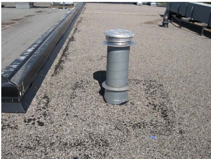
AR-041 – Asphalt bleed-through along/around flashings on BUR.
