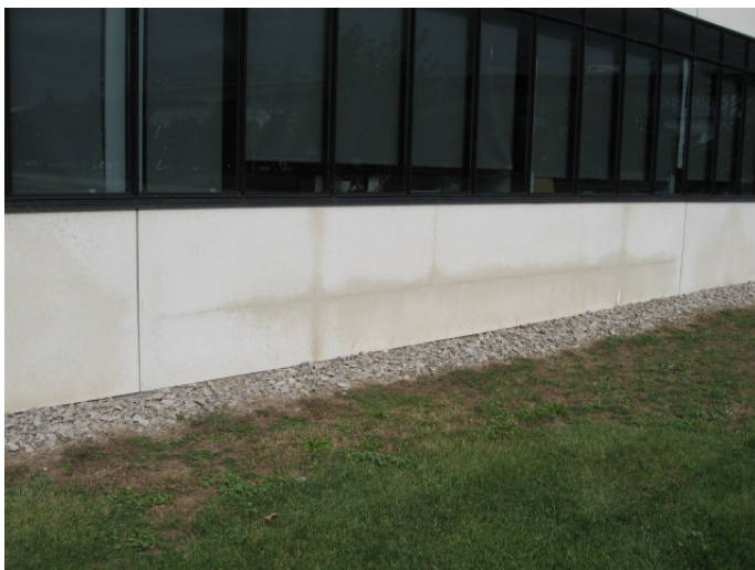
AR-023 – Defective precast concrete panel at 'east-end' addition.
