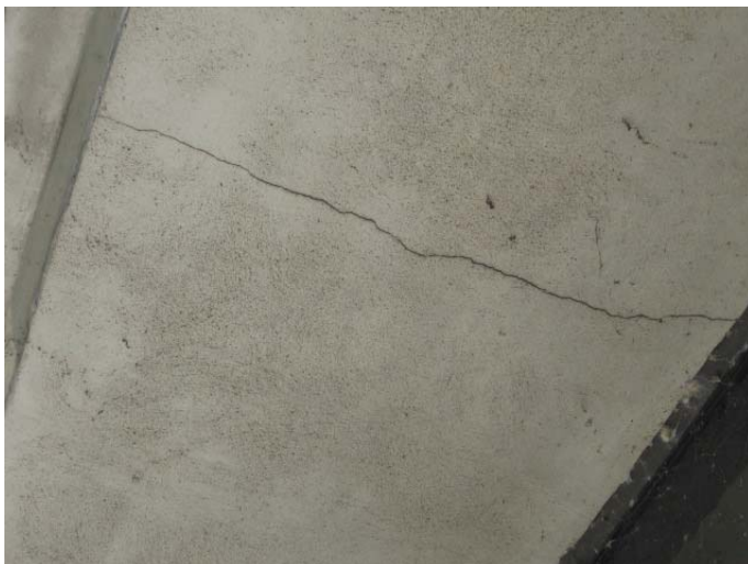
AR-025 – Cement plaster soffit with localized crack.
