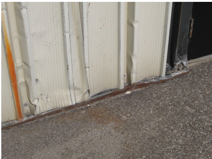
AR-009 – Damaged metal siding at south elevation.
