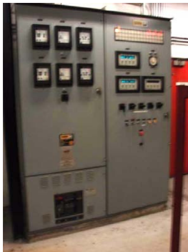
ELE-021 – Cogeneration control and transfer switch.
