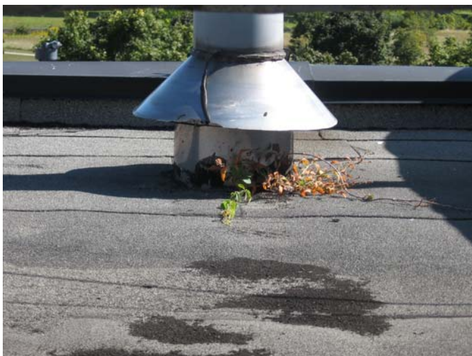
AR-031 – Vegetation growth at SBS membrane stack flashing.
