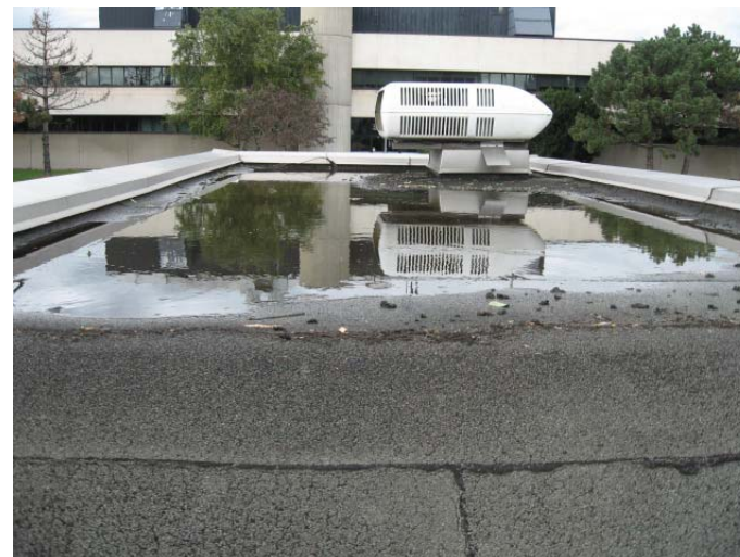
AR-058 – Standing water throughout old guardhouse roof.
