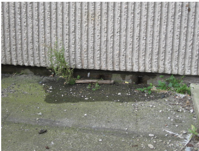
AR-007 – Moisture leakage through wall.
