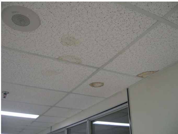
AR-105 – Several acoustic ceiling tile with water stain – cause(s) unknown.
