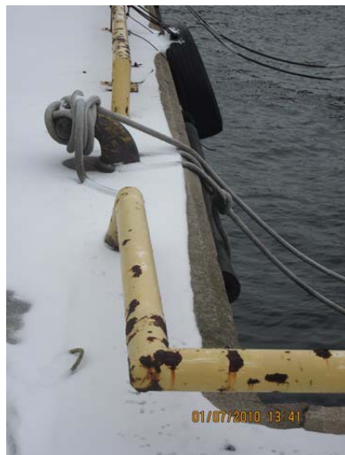
AR-081 – Deteriorated paint finish and rusting metal surfaces at wharfside guards.
