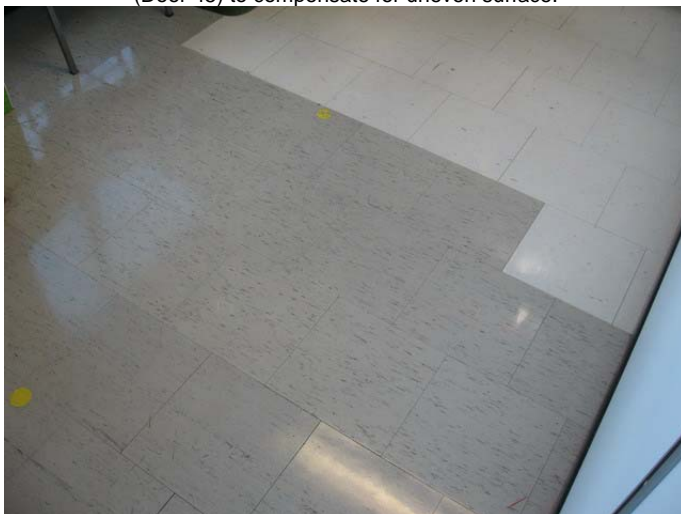
AR-091 – Close-up of vinyl tile used in localized area replacement shows 3 distinct tile colour/patterns used.
