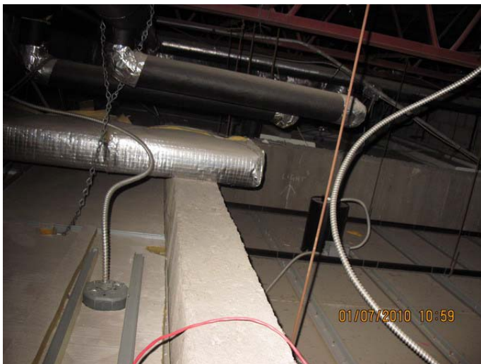
AR-121 – Fire separation between corridor and exit stairwell (HE) only extends to above suspended ceiling.
