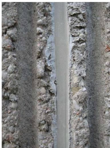
AR-027 – Sealants at concrete sandwich panel joints – old sealant visible.
