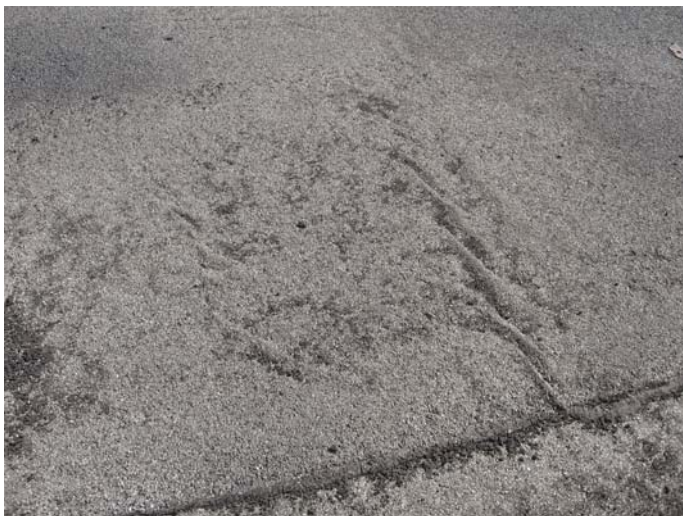
AR-037 – Wrinkling/distortion of SBS membrane.
