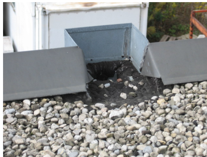
AR-024 – Exposed bitumen/membrane at BUR scupper drain.
