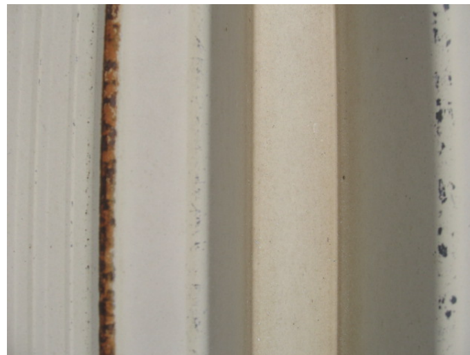
AR-006 – Deteriorating paint finish (flaking and rusting) at metal siding.
