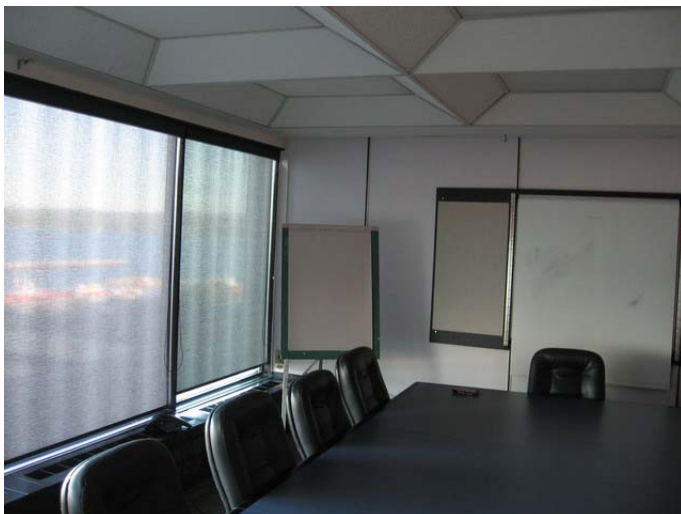
AR-107 – Coffered ceiling in conference room – components no longer commercially available.
