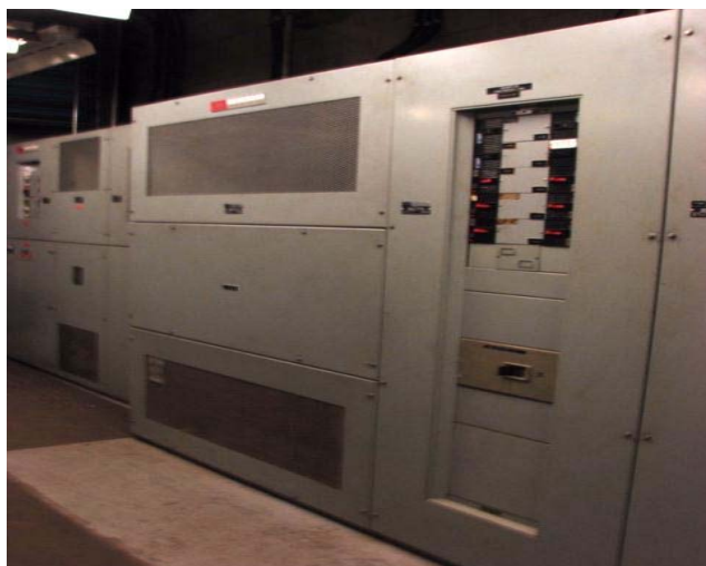
ELE-007 – Typical main 120/208 V electrical distribution switchboard.
