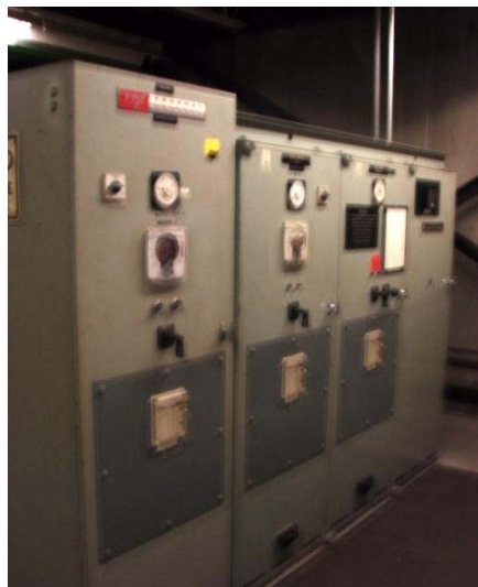
ELE-005 – Main 4160 V switchgear.
