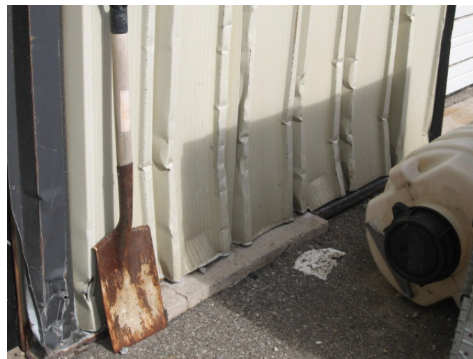
AR-008 – Damaged metal siding at south elevation.
