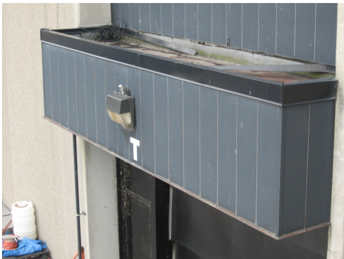
AR-013 – Rooftop debris and tangled heat trace wire at canopy drain.
