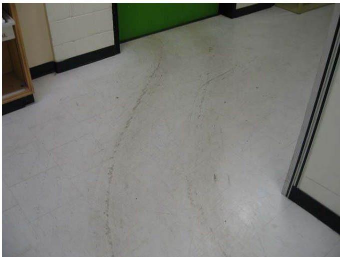
AR-095 – Vinyl tile flooring heavily worn in heavy traffic area adjacent to freight elevator.
