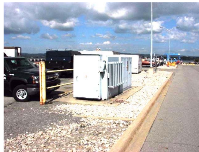
ELE-016 – Wharf Kiosk and WTC supply transformers.
