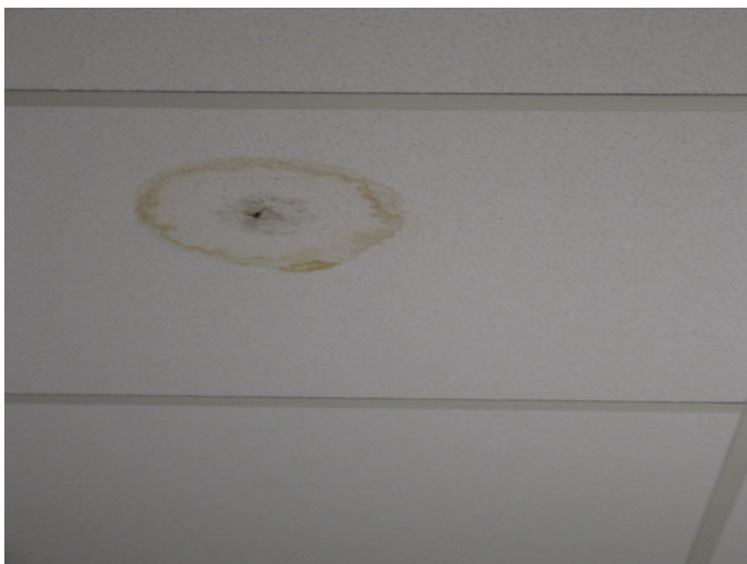
AR-063 – Water damaged/stained acoustic ceiling tile.
