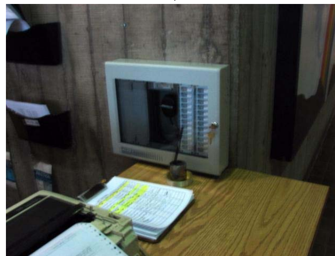
ELE-040 – Security Desk fire alarm annunciator.
