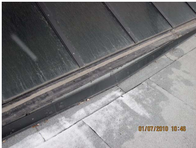
AR-061 – Loose/displaced metal flashing at SBS membrane roofing.
