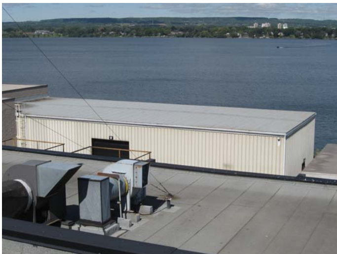
AR-017 – Modified bitumen roofing at warehouse area (view looking north from WTC Building).
