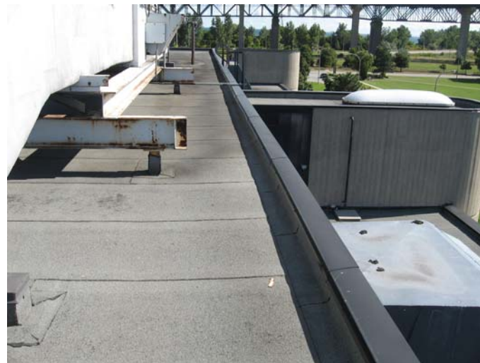
AR-034 – PH roof (south side) looking east - rusting metal equipment supports and stained SBS membrane.
