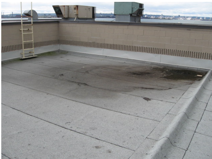
AR-021 – Staining and debris at warehouse area roof from standing water.
