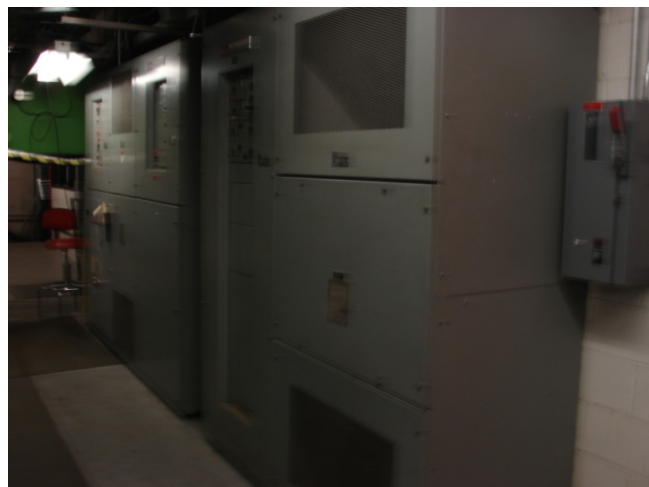
ELE-003 – Typical main 120/208 V electrical distribution switchboard.
