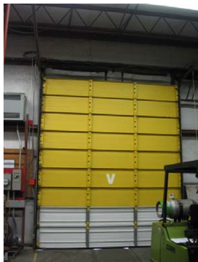
AR-031 – Uneven surface at bottom of overhead door, with daylight at several spots.
