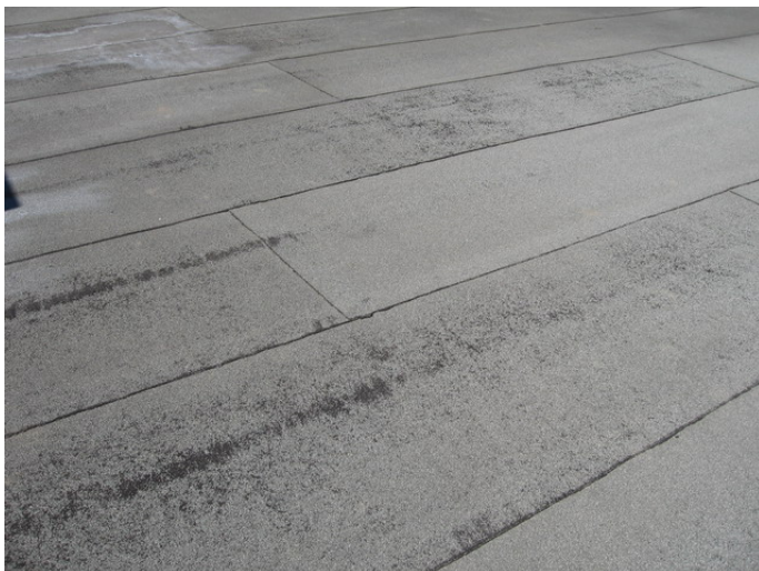
AR-049 – Ridging throughout SBS membrane at insulation joint locations.
