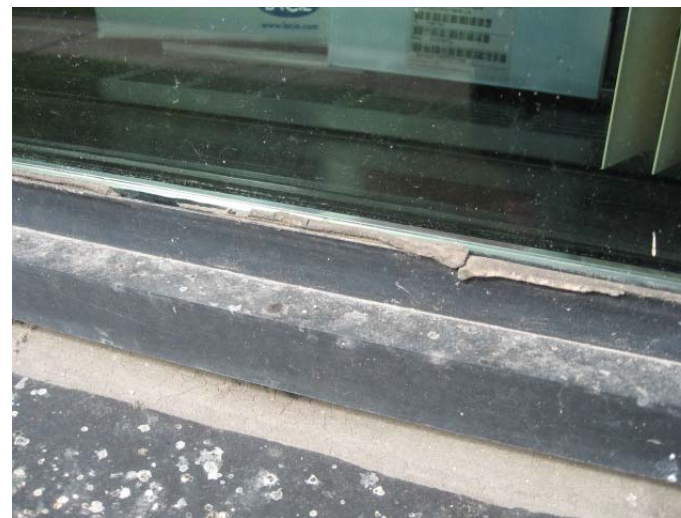
AR-046 – Deteriorated window sealants, both at frame and glazing.
