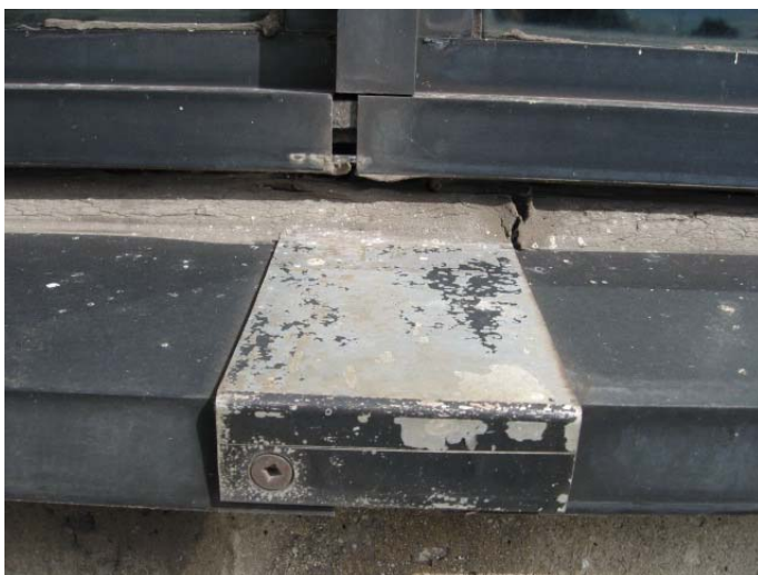
AR-047 – Open joints, deteriorated sealants and deteriorated paint finish at window framing.
