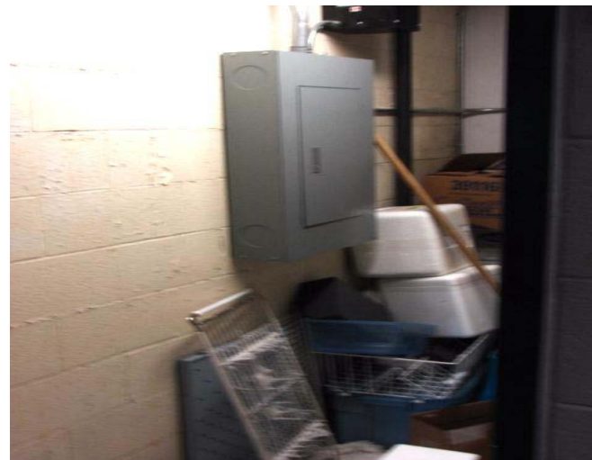
ELE-010 – Stored materials around electrical equipment.
