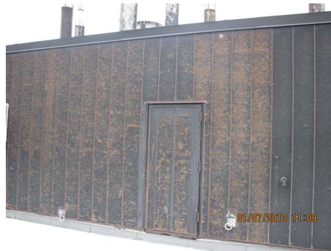
AR-040 – Deteriorated paint finish and rusting metal surfaces at A&L Mechanical penthouse west elevation metal panel wall.
