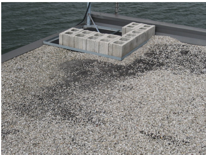
AR-023 – Exposed bitumen/membrane at BUR corner.
