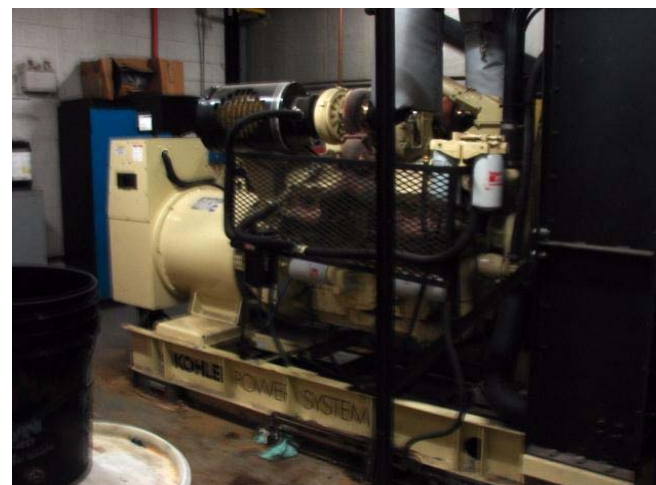
ELE-020 – Emergency power Diesel Generator.
