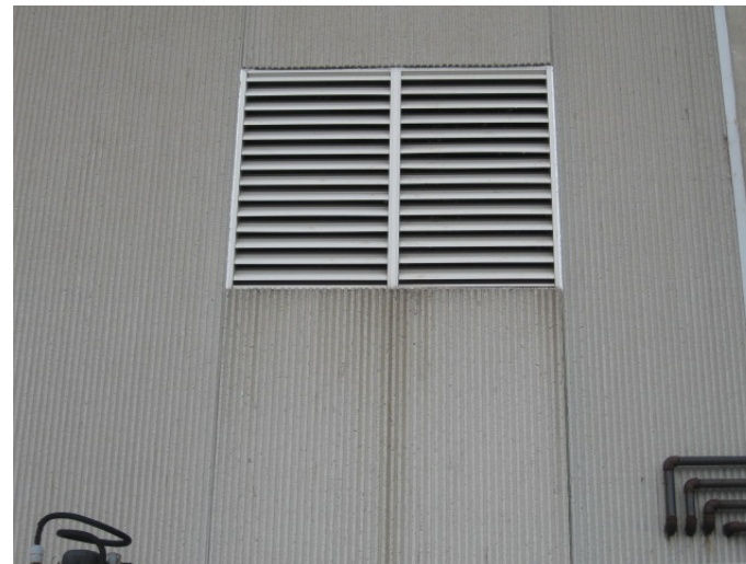
AR-006 – Stained wall surfaces below louver without sill.
