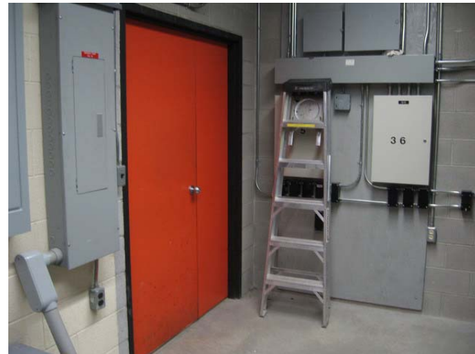
AR-128 – Equipment stored in service room – aluminum ladder with electrical equipment no less.
