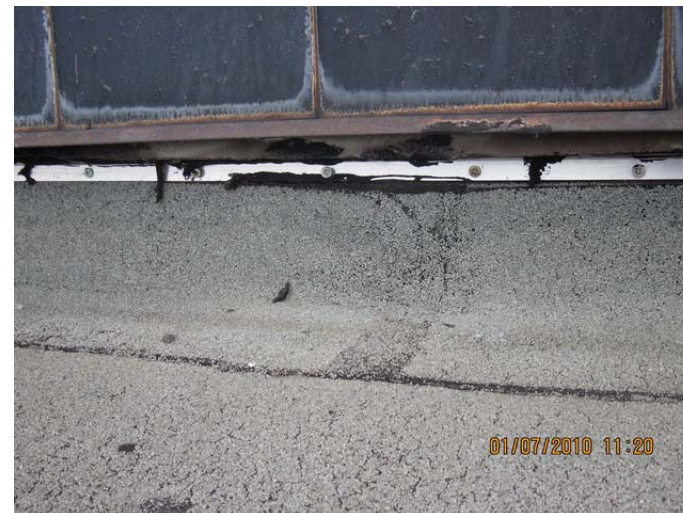
AR-070 – SBS membrane roofing pulled out from behind termination bar at penthouse flashing.
