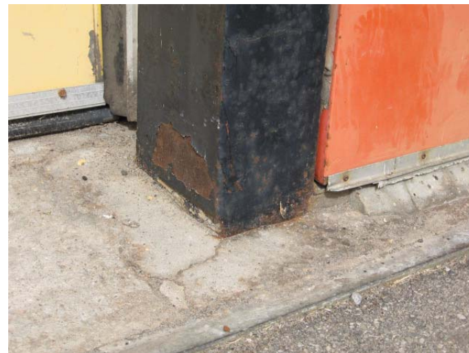
AR-050 – Deteriorated paint finish and rusting metal surfaces at door/overhead door framing.
