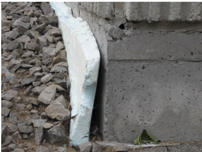
AR-029 – Exposed, shifted and deteriorating foundation insulation.
