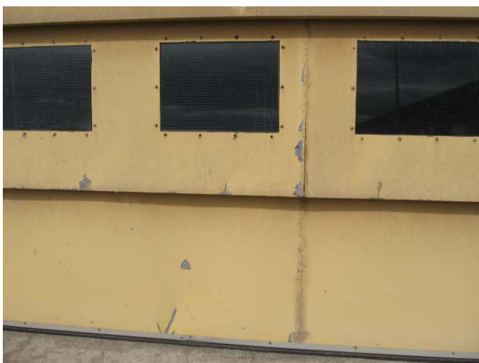
AR-051 – Deteriorated paint finish and rusting metal surfaces at overhead door panels.
