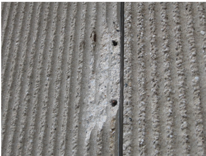
AR-015 – Holes and deteriorated concrete surface at wall panel.
