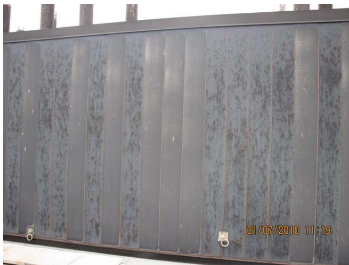
AR-041 – Deteriorated paint finish and rusting metal surfaces at A&L mechanical penthouse east elevation metal panel wall.
