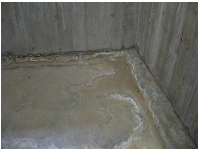
AR-057 – Water stained surfaces at basement level.
