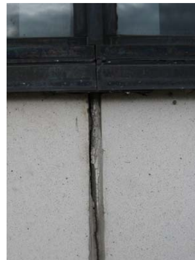
AR-026 – Deteriorating sealants at 'east-end' addition wall panel and window.
