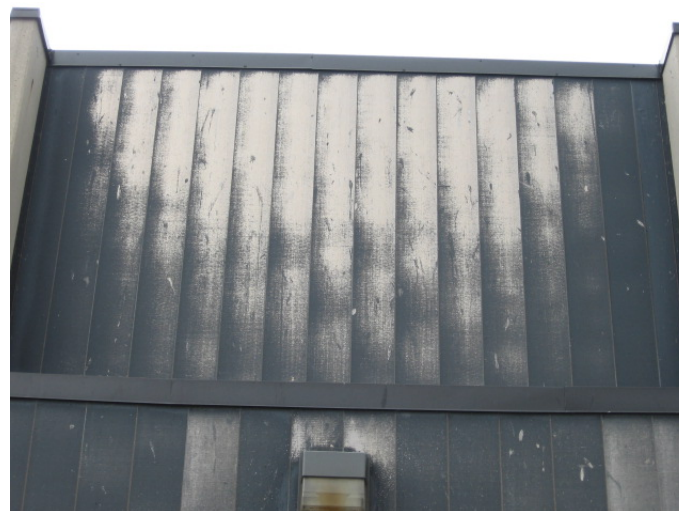
AR-016 – Deteriorated paint finish at metal siding above canopy.
