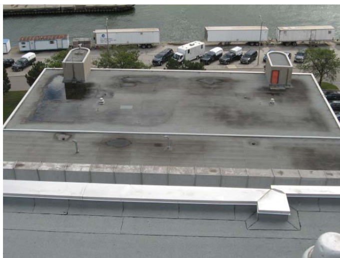
AR-063 – Darker stained locations indicate locations of standing water throughout roof areas.
