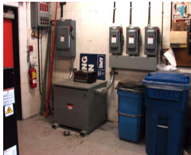
ELE-006 – Stored materials around electrical equipment.
