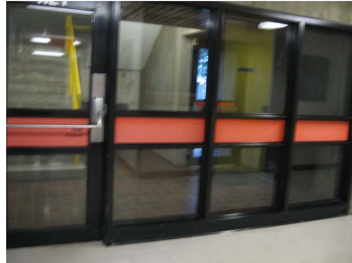
AR-126 – Glazing at exit stair vestibule may exceed allowable limits.
