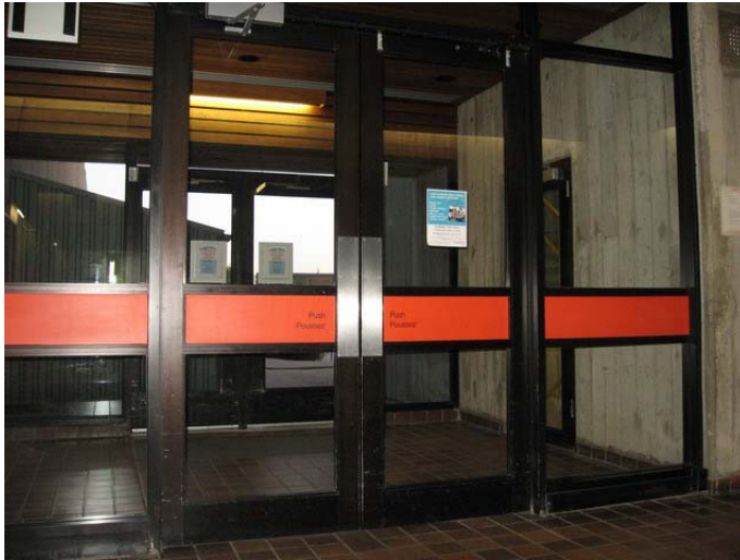
AR-125 – Vestibule at exit stair (NW) with clear glazing and no latching hardware.
