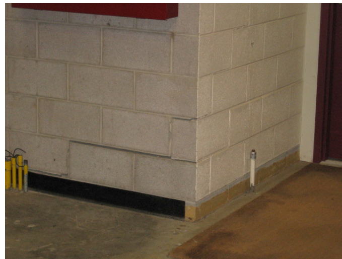
AR-058 – Open block joints at wall in high-bay area.
