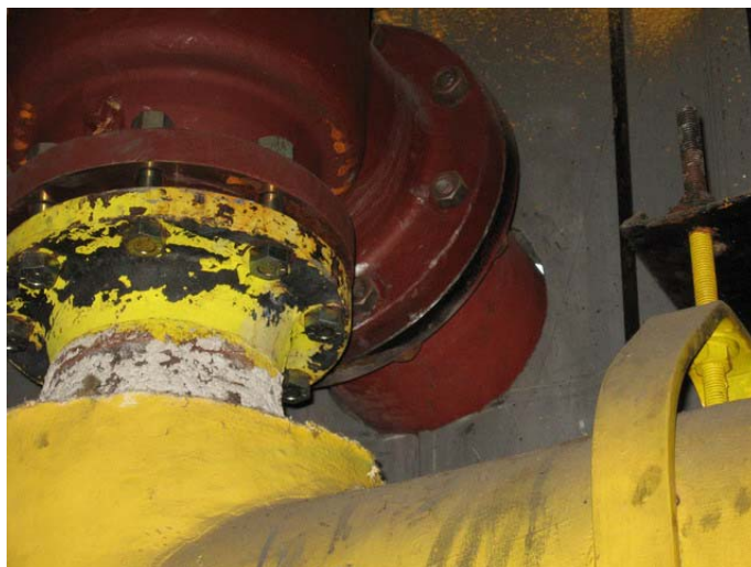
AR-043 – Unsealed penetration in R&D mechanical penthouse metal panel wall.
