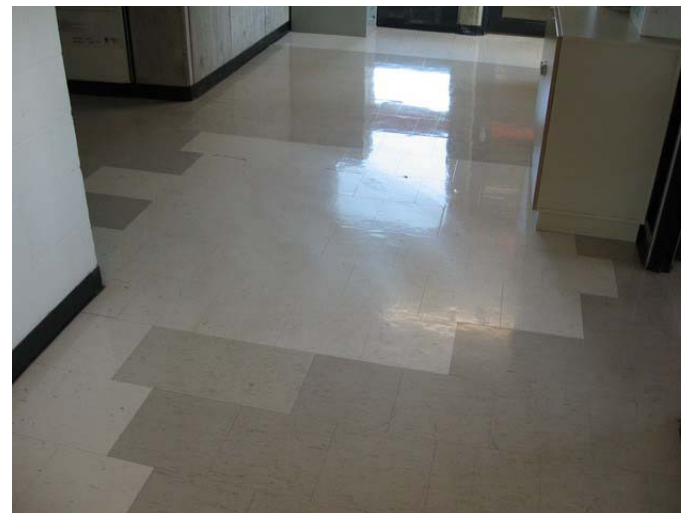
AR-090 – Mismatched vinyl tile used in localized area replacement.
