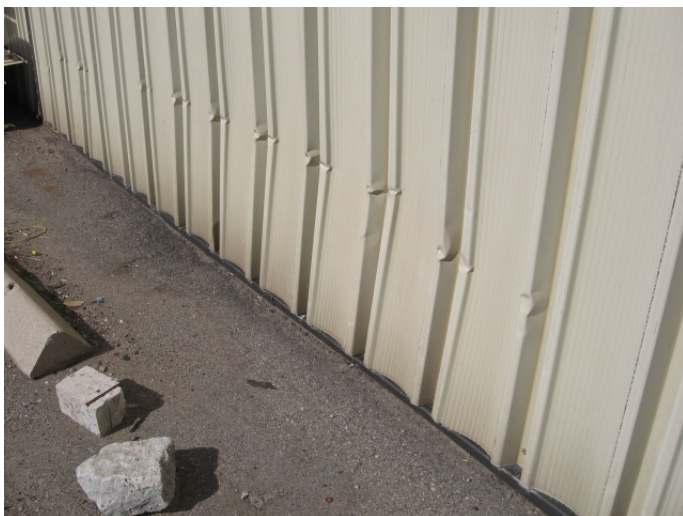
AR-007 – Damaged metal siding at south elevation.
