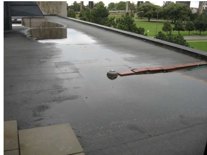
AR-056 – Ponding and blocked drain at main roof.
