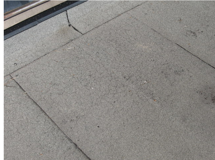
AR-054 – Cracking of SBS membrane surface in field.
