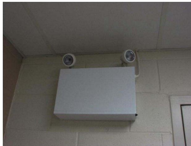
ELE-034 – Typical emergency battery pack.
