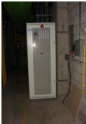
ELE-041 – Additional fire alarm booster panels.
