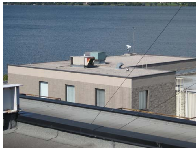
AR-016 – Built-up roofing at office area (view looking north from WTC Building).
