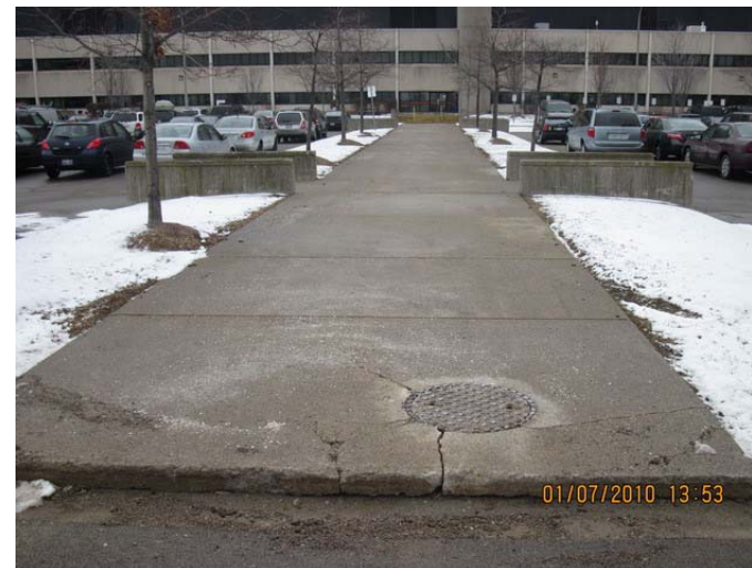
AR-086 – Cracked/broken concrete at walkway through parking area.
