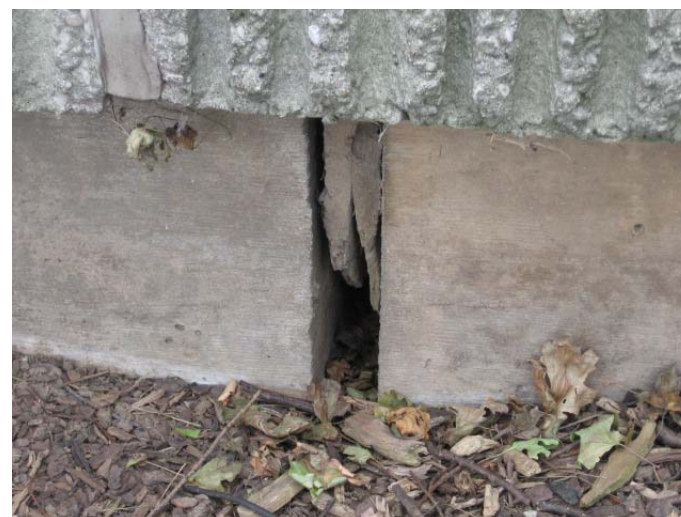
AR-016 – Unexplained void in foundation at Hydraulics lab north elevation.
