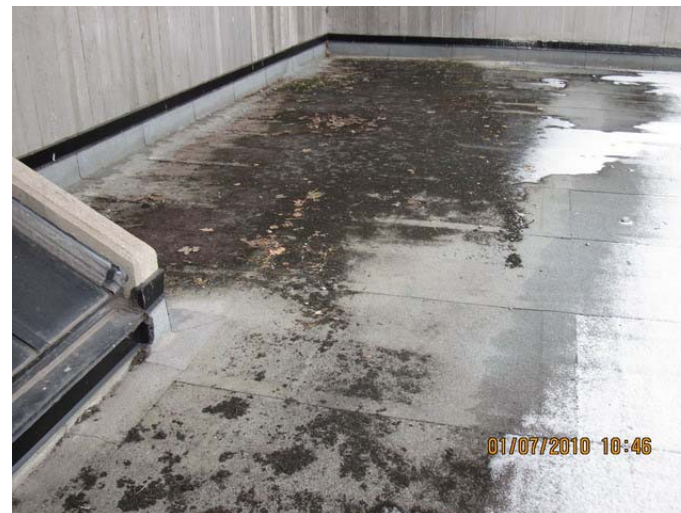
AR-062 – Debris and sediment from standing water accumulation at SBS membrane roofing.
