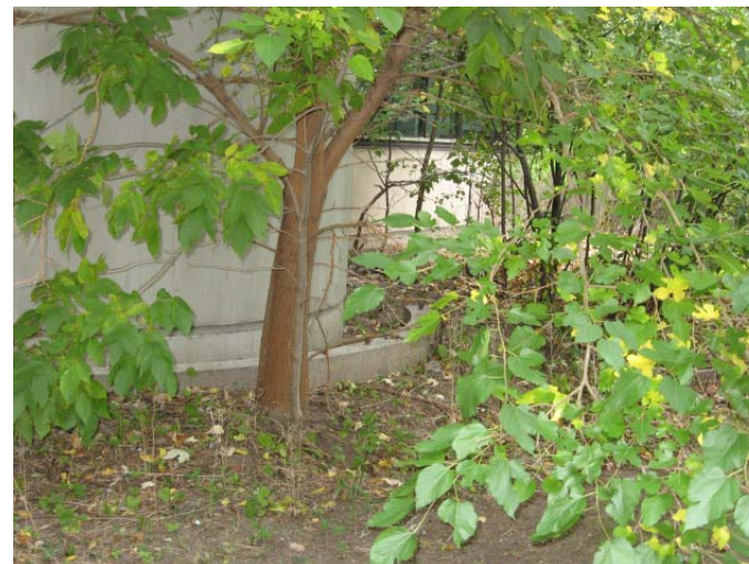
AR-074 – Proximity of vegetation to building face invites foundation damage from roots.
