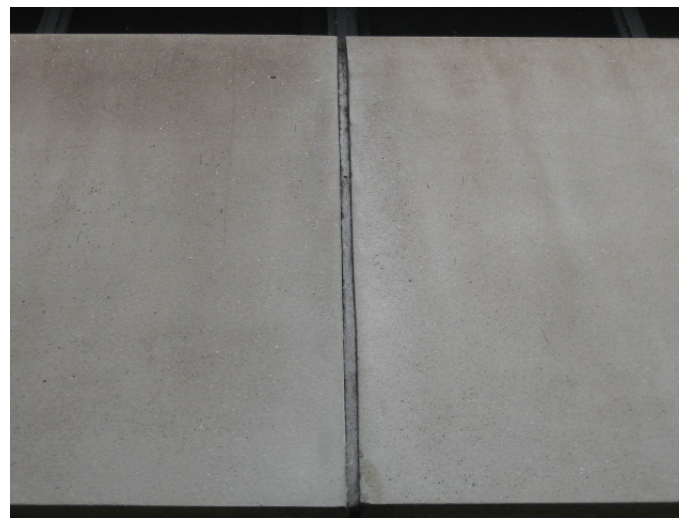
AR-020 – Debonded sealant at precast concrete panel joints.
