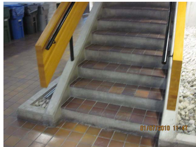
AR-114 – Mall open circulation stair guards with unprotected openings and handrails without extensions and returns.
