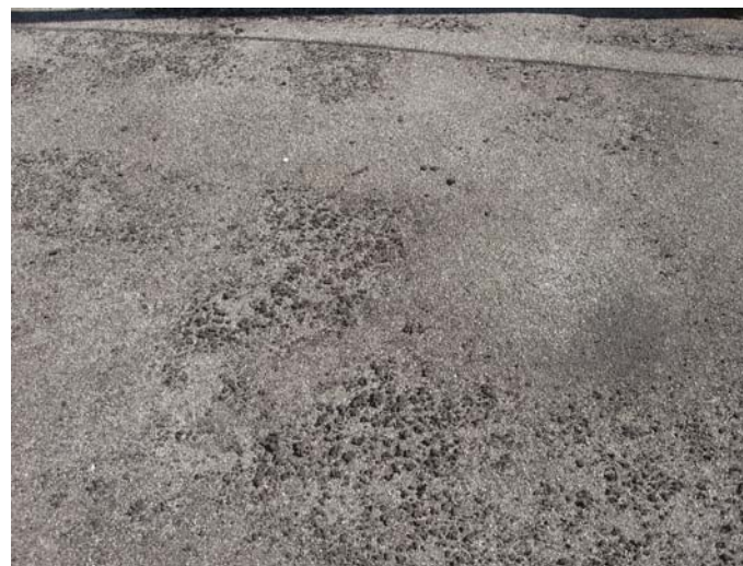
AR-036 – Sediment/debris build-up on SBS membrane source from standing water.
