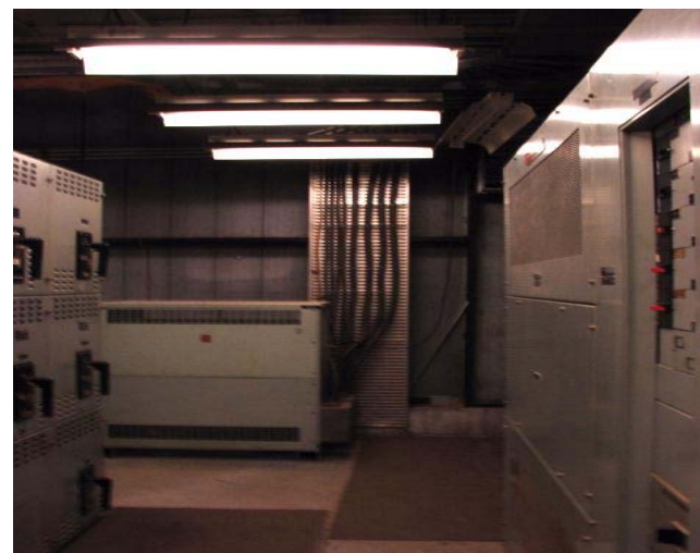
ELE-008 – Typical main 120/208 V electrical distribution switchboard.
