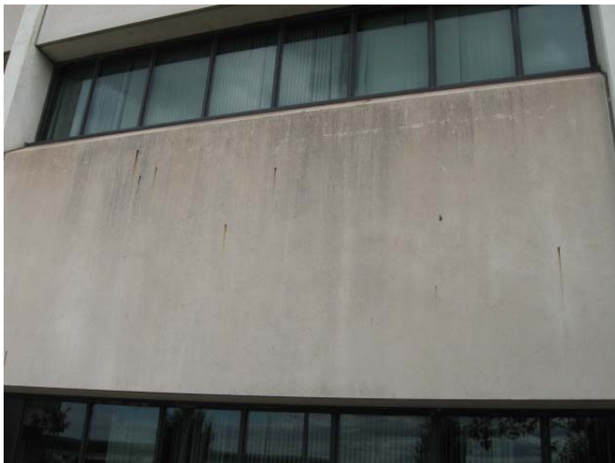
AR-033 – Rusting at exposed rebar and general surface staining/ Discolouring of concrete panels at Hydraulics Lab offices.
