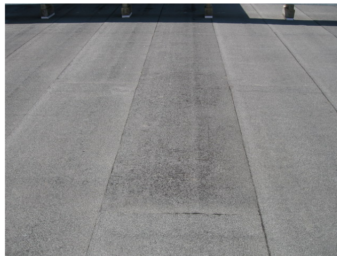
AR-052 – Loss of granular surfacing of SBS membrane roll in field.
