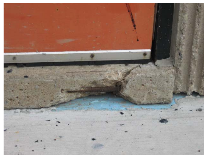
AR-052 – Deteriorating concrete door sill at Boiler Plant (Door 15).
