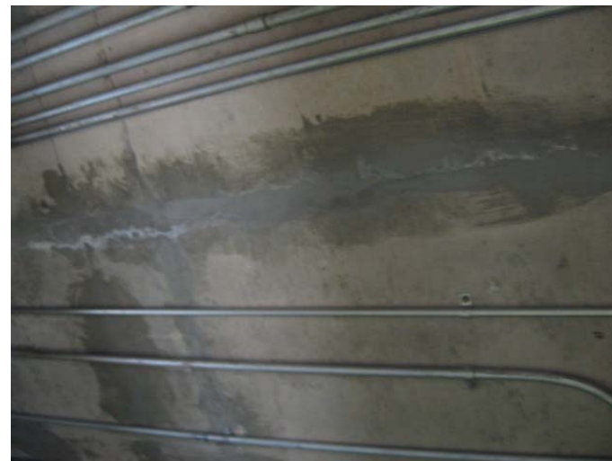
AR-022 – Water staining and efflorescence along ceiling crack in tunnel.
