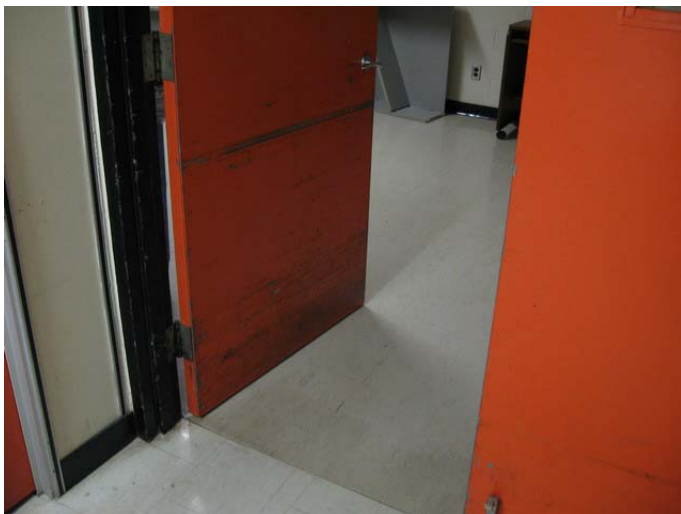
AR-111 – Deteriorated paint finish at metal door in high-traffic location.
