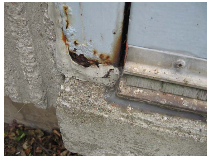
AR-056 – Deteriorated sealant, deteriorated paint finish and rusting metal surfaces at door frame.
