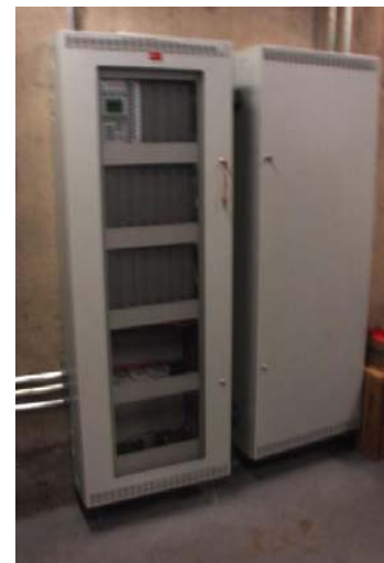
ELE-042 – Additional fire alarm booster panels.
