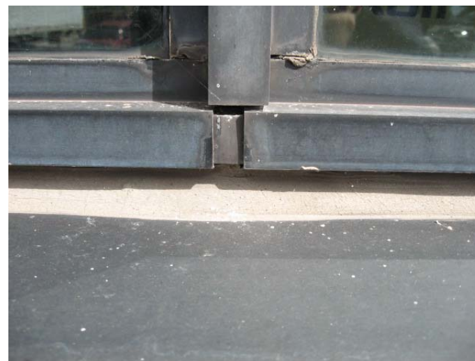
AR-048 – Open joints and deteriorated sealants at window framing.
