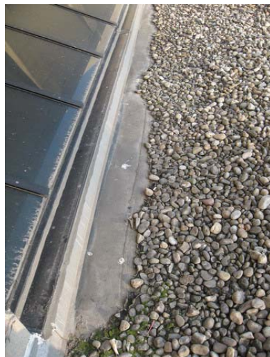
AR-059 – Tenting membrane and displaced ballast at EPDM membrane roofing.
