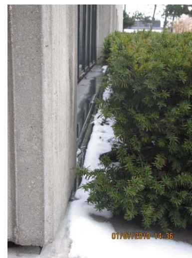
AR-072 – Proximity of vegetation to building face inhibits access for inspection and maintenance.
