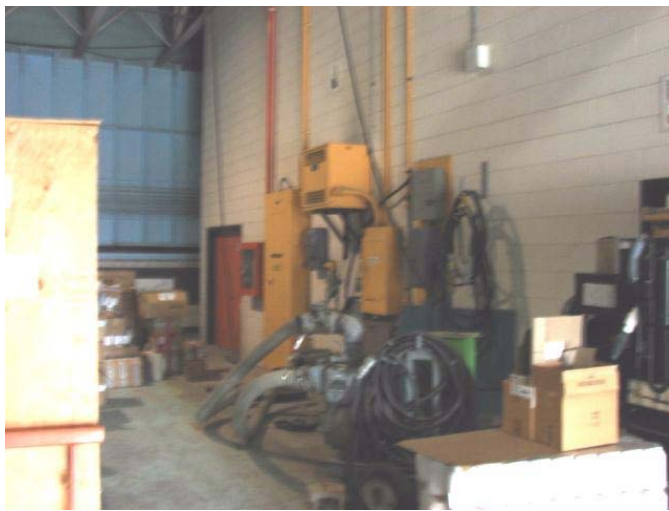
ELE-017 – Stored material around electrical equipment and no guarding.
