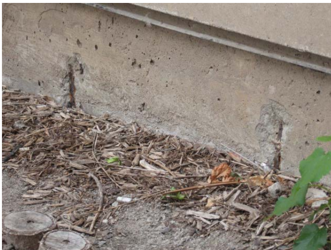
AR-013 – Exposed rebar with deteriorated concrete at foundation.
