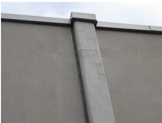
AR-035 – Cracks in cementitious coating on exposed column at R&D west elevation.
