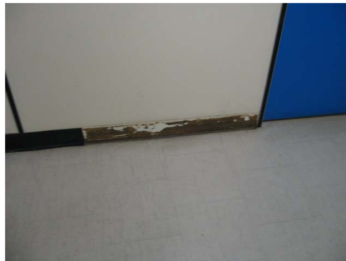
AR-102 – Missing vinyl base – localized throughout.
