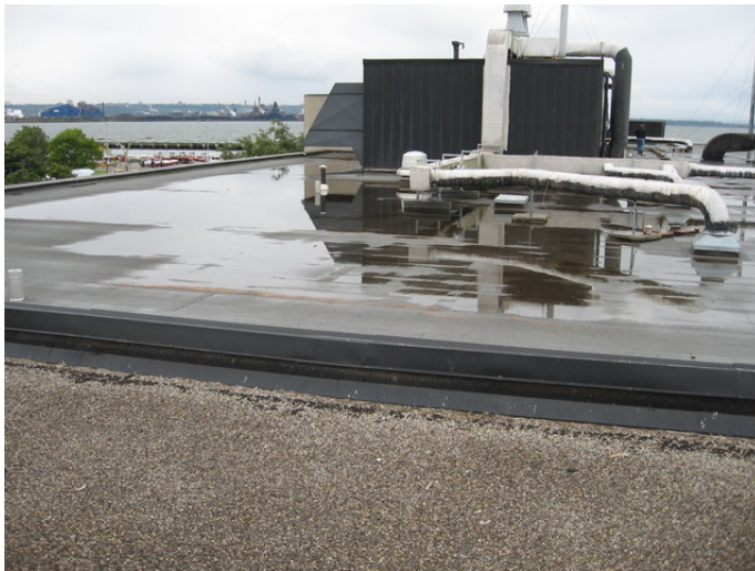
AR-055 – Ponding throughout main roof.
