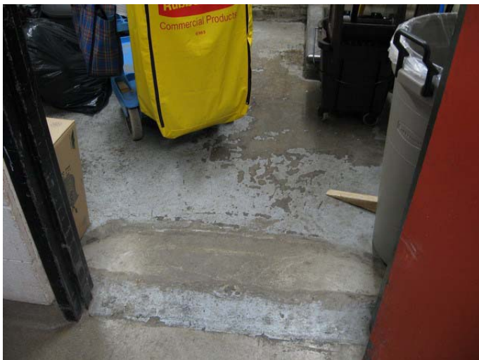
AR-101 – Deteriorated paint finish at janitor room floor.
