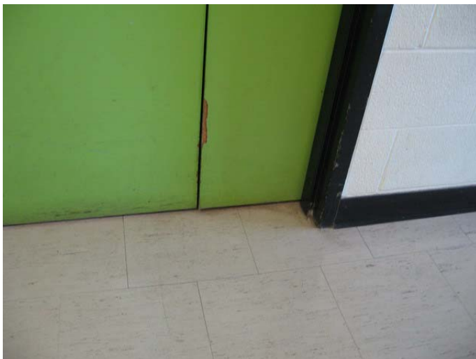
AR-109 – Damaged plastic laminate door finish.
