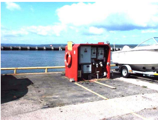
ELE-015 – Typical Wharf Kiosk for ship power.
