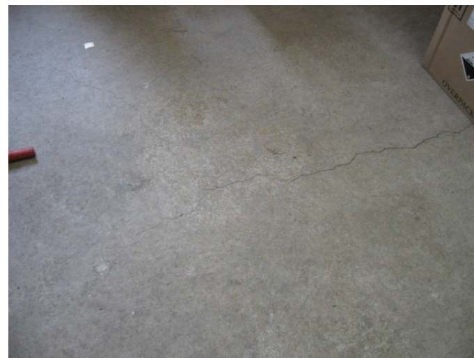
AR-032 – Cracked concrete floor slab in warehouse area office.
