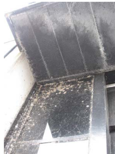
AR-012 – Dirty surfaces (webs, debris, etc.) and deteriorated paint finish at underside of canopy.
