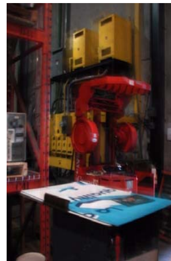
ELE-018 – Stored material around electrical equipment and no guarding.
