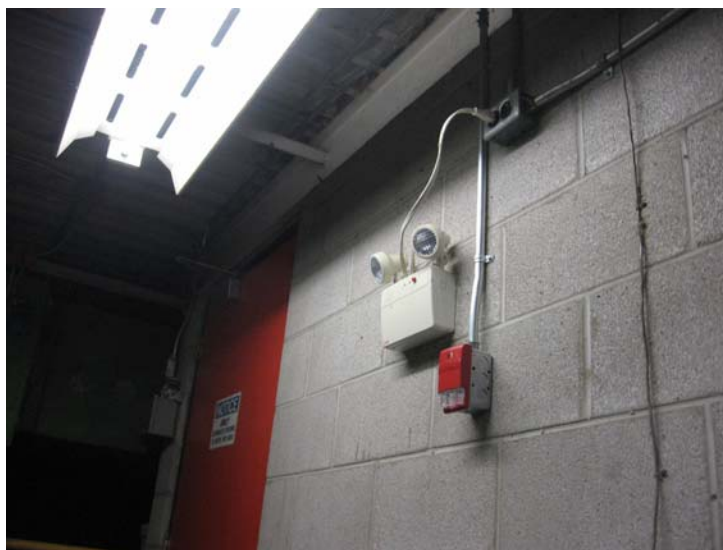
ELE-011 – Typical emergency power battery pack.
