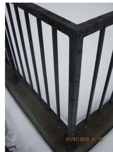
AR-068 – Deteriorated paint finish and rusting metal surfaces at rooftop guard.
