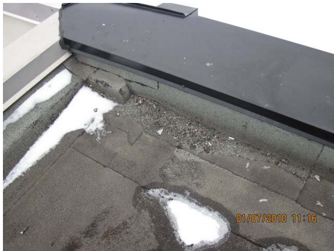
AR-069 – Debris accumulation at SBS membrane roofing.
