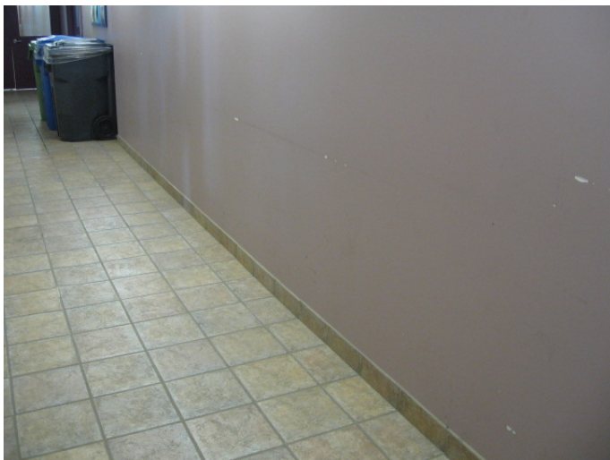
AR-061 – Damaged wall surfaces in 1st floor corridor.
