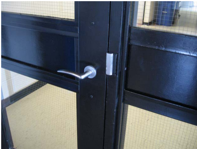
AR-127 – Electric door strike in fire separation – unconfirmed if operation is 'fail secure' or 'fail safe'.
