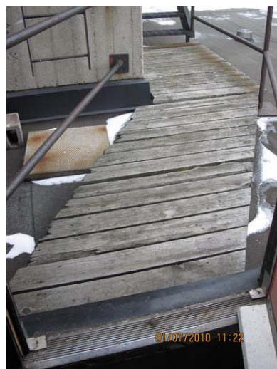
AR-071 – Deteriorated paint finish, rusting metal surfaces and deteriorating wood at rooftop guards and walkway.
