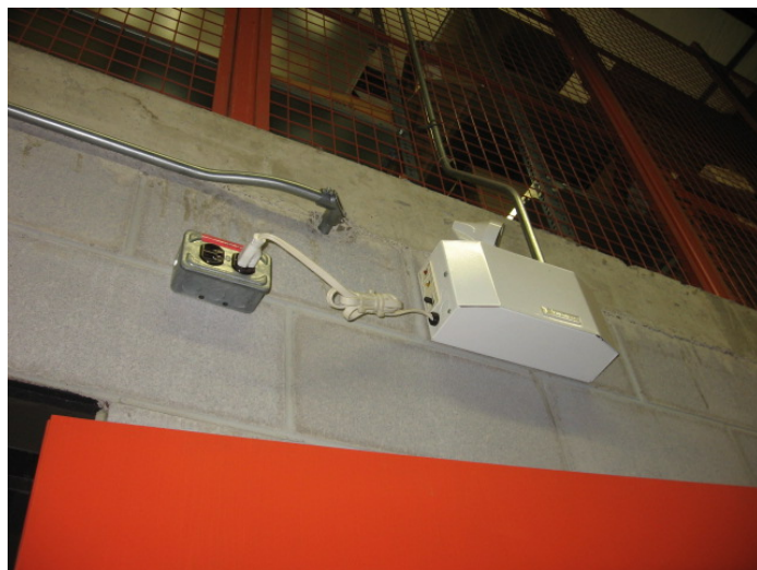
ELE-007 – Typical emergency battery pack.
