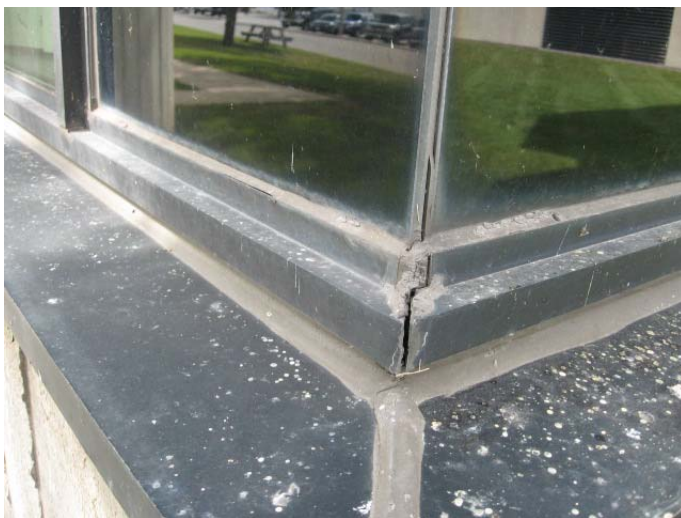
AR-045 – Open joints at window glazing/finishing at Hydraulics Lab office.
