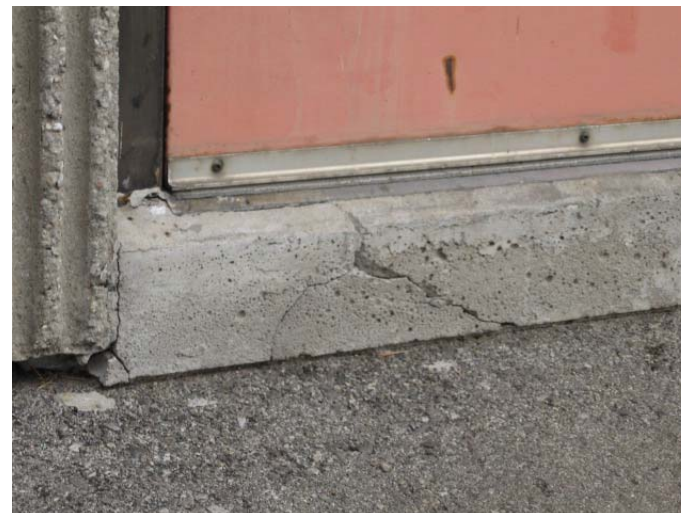
AR-054 – Deteriorating concrete door sill at Warehouse (Door 30).
