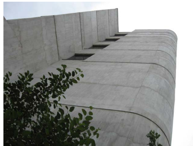
AR-026 – Concrete exterior wall with cementitious coating at A&L exit stairwell (SE).
