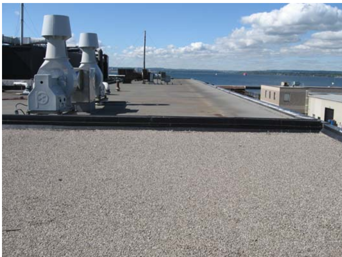
AR-045 – Discoloured SBS membrane from standing water - view looking west.
