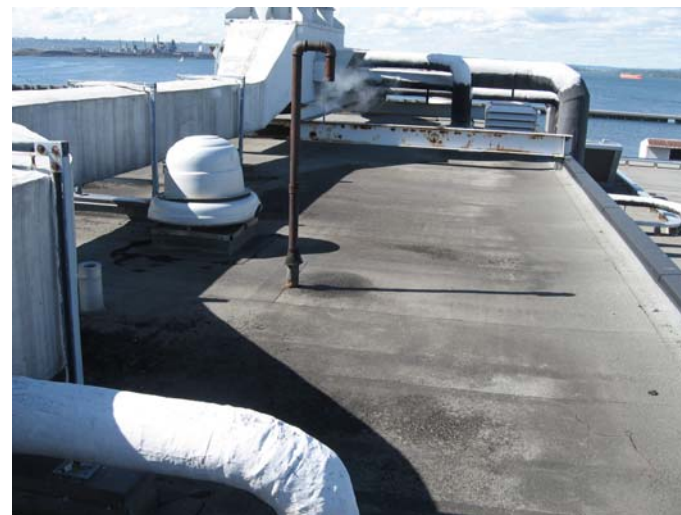
AR-032 – PH roof (north side) looking west - rusting metal equipment supports and stained SBS membrane with sediment/debris build-up.
