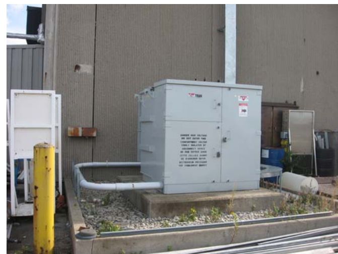
ELE-004 – Primary Transformer – 4160 to 600 volts.
