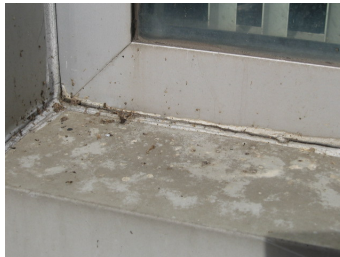
AR-010 – Deteriorated sealant at window.
