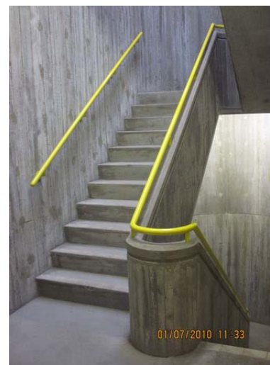
AR-116 – Exit stair handrails without extensions and returns.
