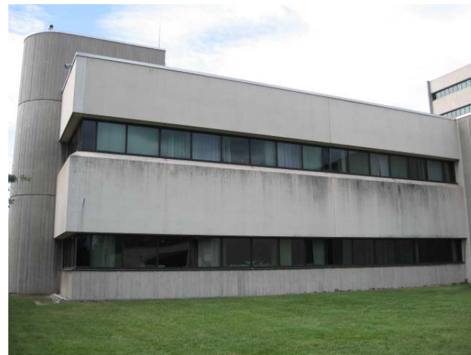
AR-030 – Stained/discoloured surfaces of concrete panels at Hydraulics lab offices.
