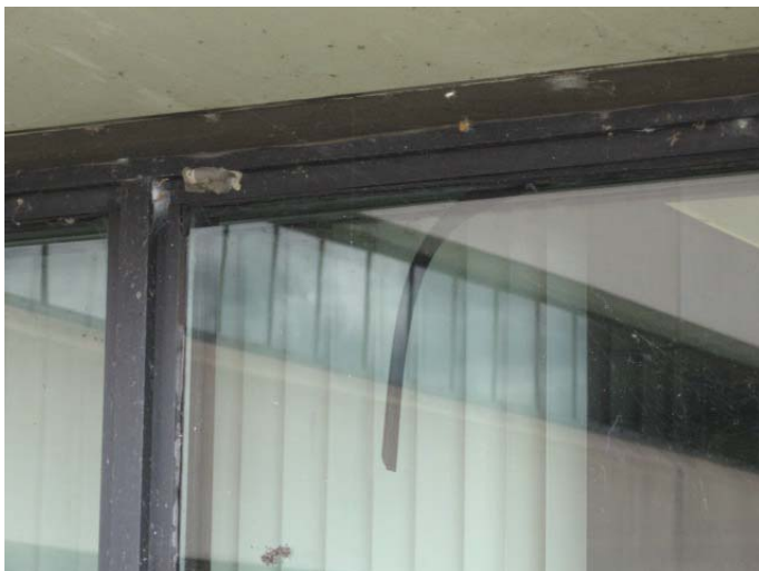
AR-049 – Part of windows interior glazing gasket fallen from place.
