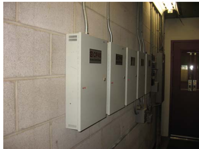
ELE-046 – Typical card access control panels.
