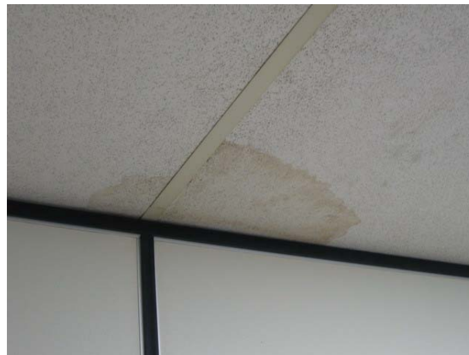
AR-104 – Acoustic ceiling tile with water stain – cause unknown.
