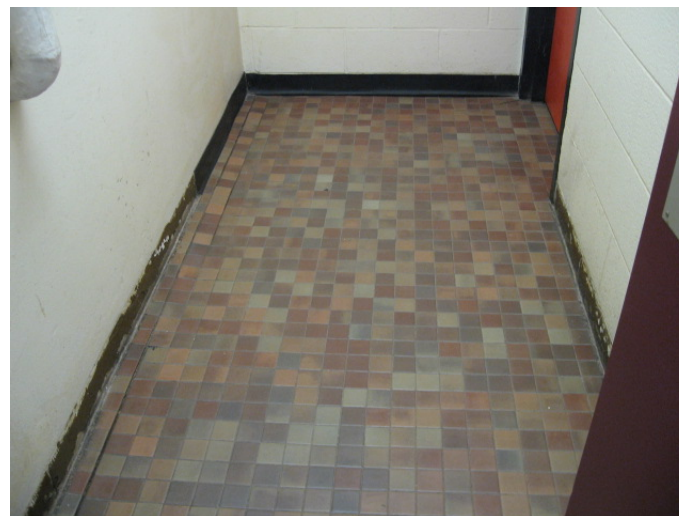
AR-060 – Shifted floor in 1st floor washroom/change room vestibule.
