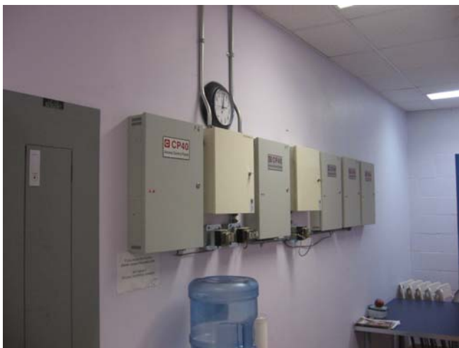
ELE-047 – Typical card access control panels.
