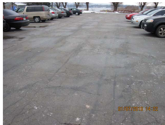
AR-084 – Cracking/alligating of 'residential grade' asphalt pavement throughout driveway.
