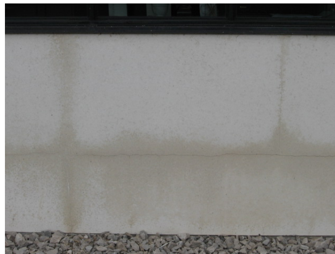
AR-024 – Cracks and discolouration at precast concrete panel.
