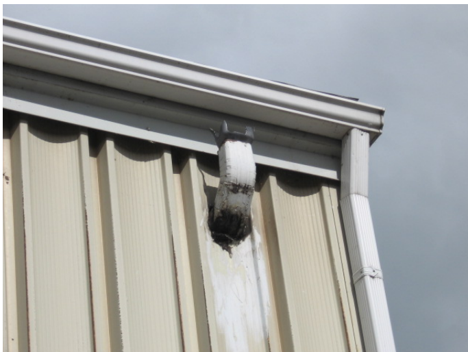
AR-013 – Poorly sealed wall penetration at now abandoned downspout.
