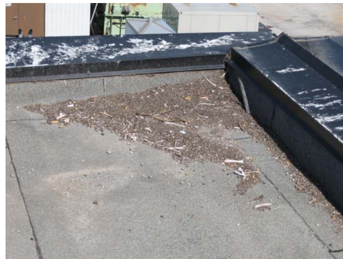
AR-046 – Accumulation of debris in corners of SBS roofing.
