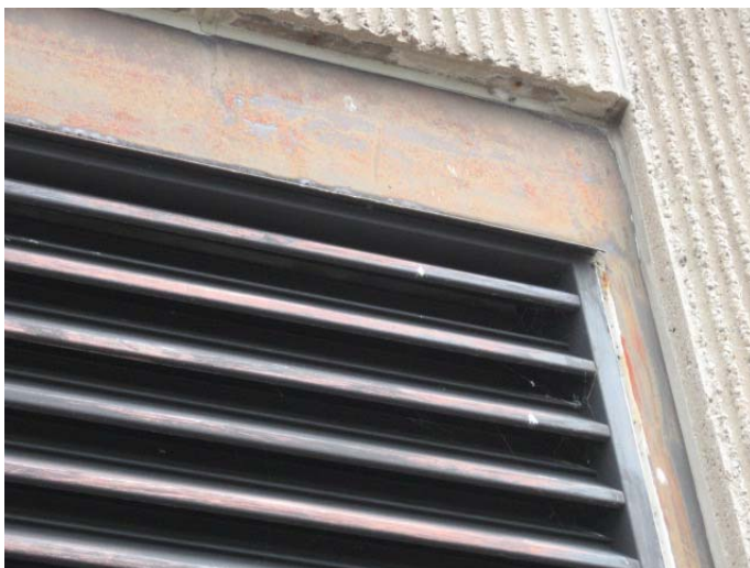
AR-031 – Deteriorated paint finish and rusting metal surfaces at louvre.
