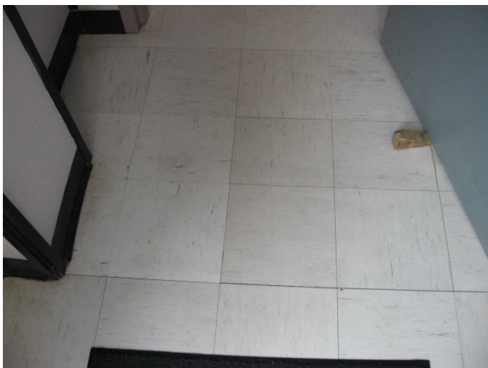
AR-027 – Open tile joints (from shrinkage) at 1st floor entrance lobby.
