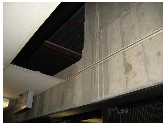
AR-120 – Opening in fire separation between corridor and exit stairwell (HE)
