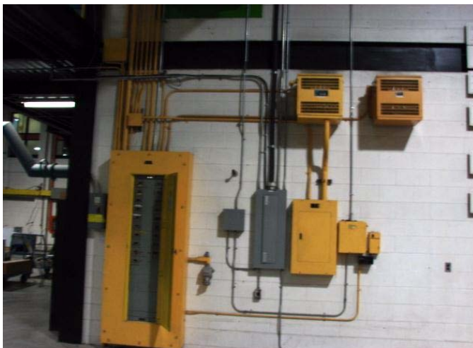
ELE-013 – Wet Lab panels with no guarding.
