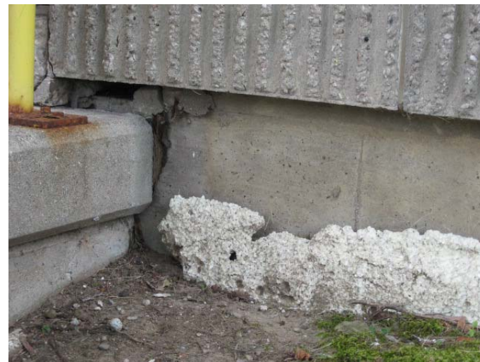
AR-014 – Exposed and deteriorating foundation insulation at Warehouse north elevation.
