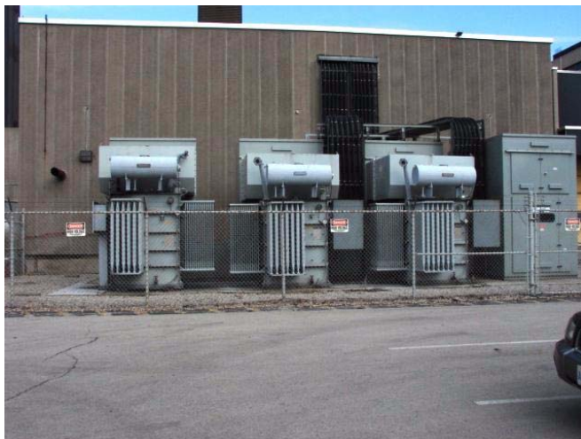
ELE-001 – Main transformers and high voltage switchgear.
