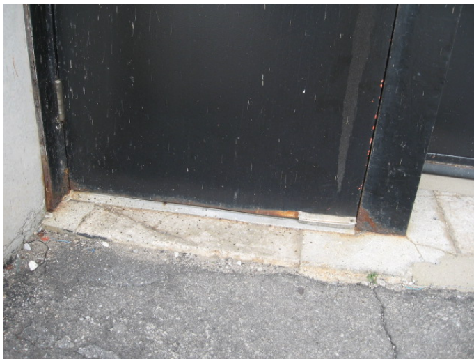
AR-011 – Deteriorated paint finish and rusting metal surfaces at exterior door.
