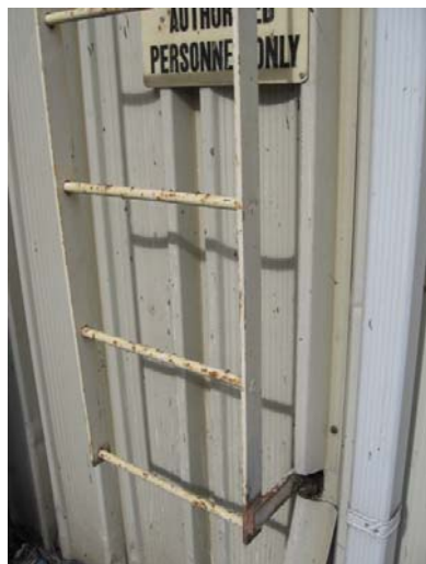
AR-015 – Deteriorating paint finish and rusting metal surfaces at roof access ladder.
