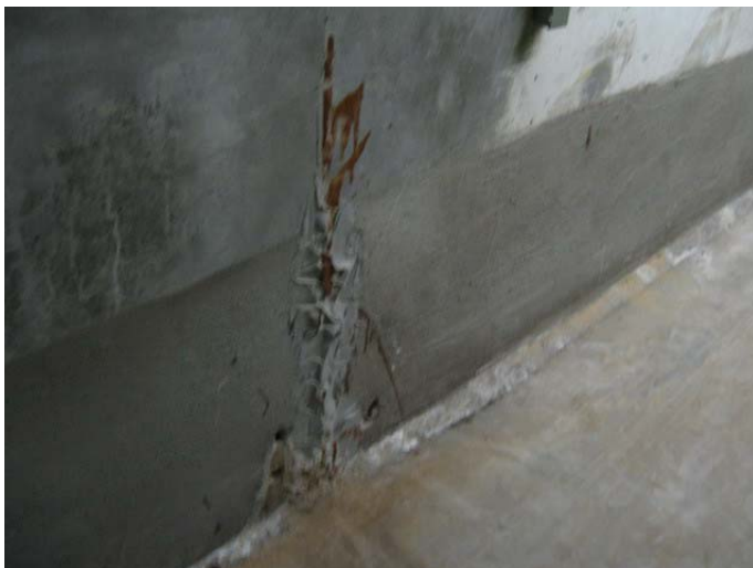
AR-023 – Previous crack repair (poorly executed) in tunnel wall.
