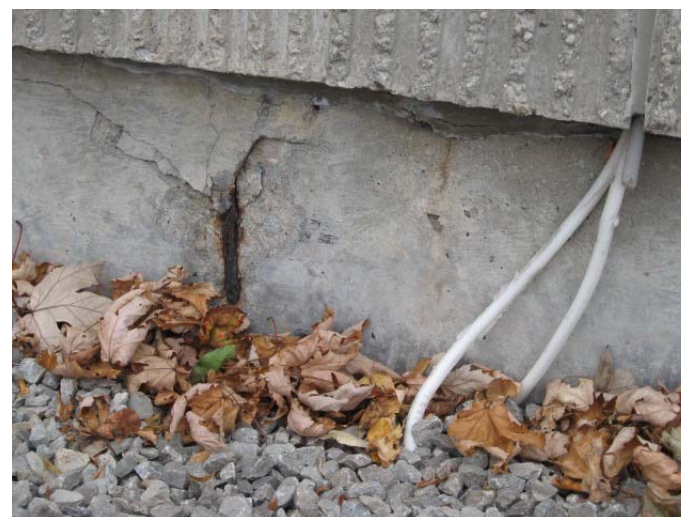
AR-012 – Exposed rebar/deteriorating concrete at foundation, and undersized sealant backer rods falling out from behind wall panel.
