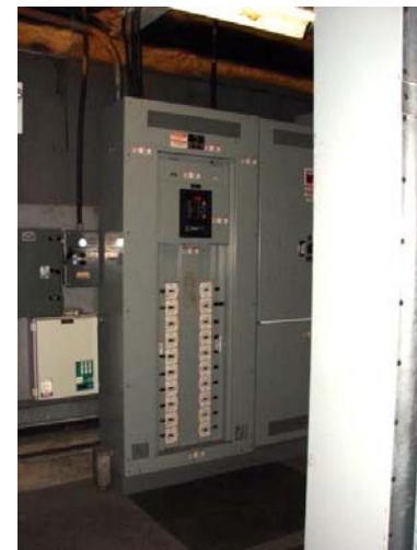
ELE-002 – Main 120/208V distribution for Labs and Offices.
