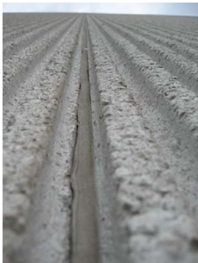
AR-005 – Debonded sealant at precast concrete sandwich panel joints.
