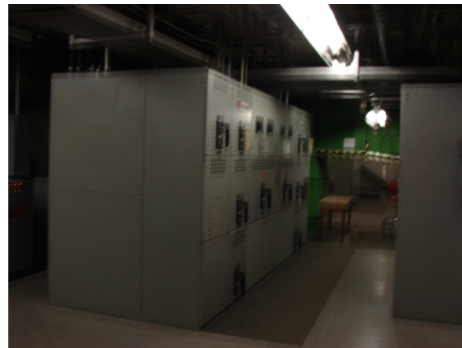
ELE-002 – Typical main 600 V electrical distribution switchboard.
