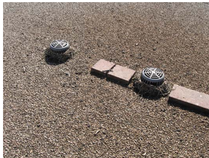
AR-044 – Debris around BUR area drains.
