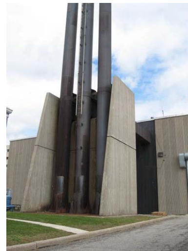
AR-018 – Concrete chimney support structure and rusting metal chimneys/breechings at Boiler Plant west elevation.
