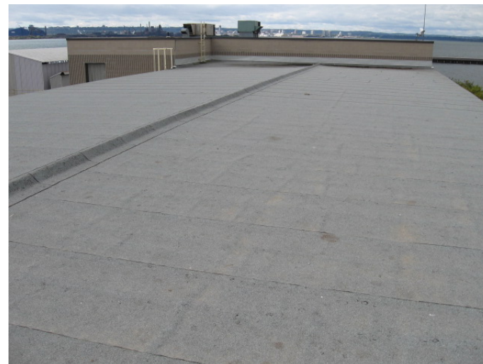
AR-018 – Ridging of membrane throughout warehouse area roof.
