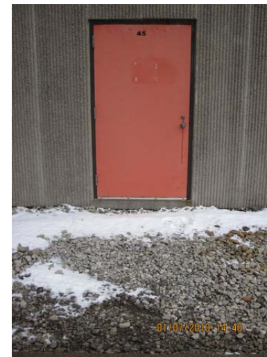
AR-088 – Exit stair (WS) exterior door (Door 44) leading on to uneven surface.
