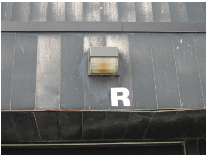
AR-017 – Deteriorated paint finish and damaged soffit at canopy.
