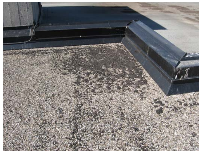
AR-040 – Asphalt bleed-through at field area on BUR.
