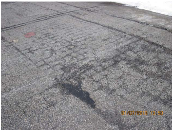
AR-085 – Deteriorated asphalt paving at wharfside outdoor storage/work area.
