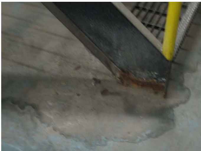
AR-113 – Deteriorated paint finish and rusting metal at Boiler Plant stair.
