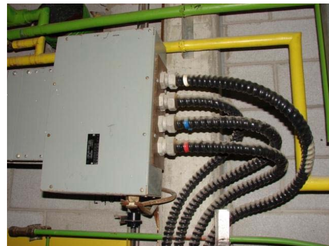
ELE-012 – Bus duct which feeds all upper floor lab panels.
