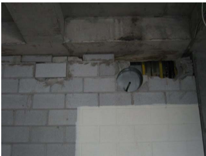
AR-119 – Unprotected openings in fire separation between lab and service core.
