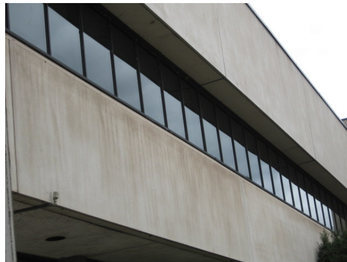
AR-022 – Surface staining at precast concrete panel surfaces.
