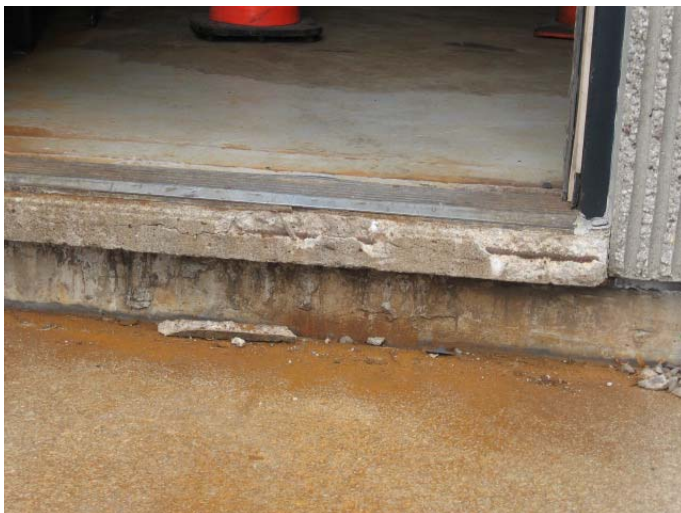
AR-053 – Deteriorating concrete door sill at Boiler Plant (Door 17).
