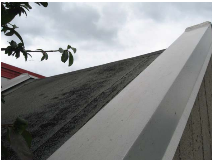
AR-057 – Deteriorated SBS roofing membrane at old guardhouse roof.
