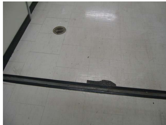
AR-094 – Vinyl tile breaking at building control joint.
