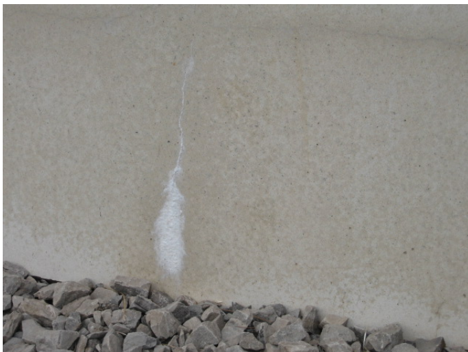
AR-025 – Efflorescence accumulating around cracks in precast concrete panel.
