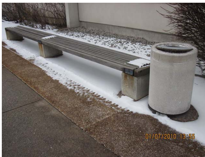
AR-075 – Rusting metal components and stained surfaces at exterior bench.
