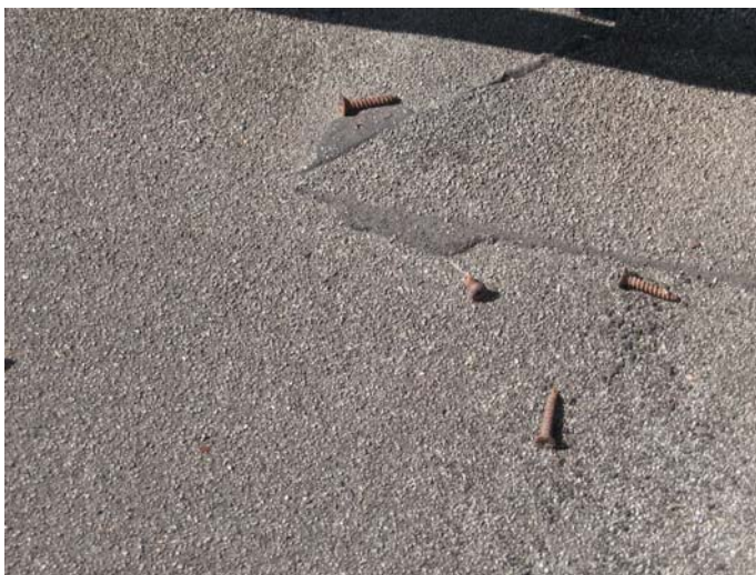
AR-035 – Old fasteners lying on SBS membrane - a puncture waiting to happen.
