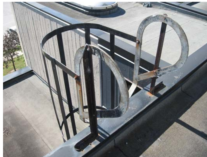
AR-038 – Deteriorating paint finish and rusting metal surfaces at PH roof access ladder.
