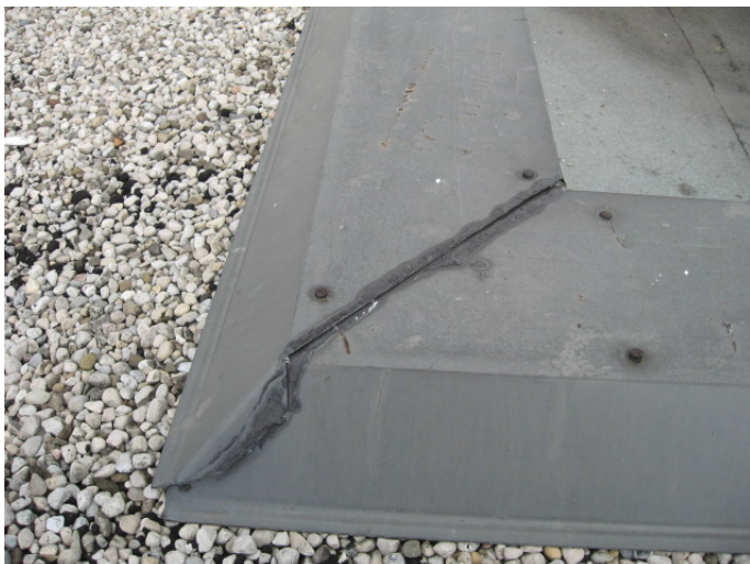
AR-025 – Deteriorated sealant at joints BUR metal counter flashing.
