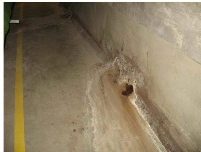
AR-024 – Water staining from ongoing seepage at tunnel wall/floor.
