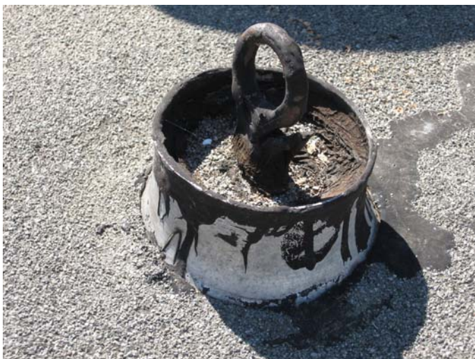
AR-047 – Deteriorated filler in abandoned pitch pocket.
