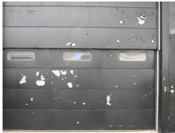
AR-018 – Deteriorated paint finish and rusting metal surfaces at exterior overhead door.
