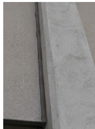
AR-036 – Debonding sealant at concrete panel.
