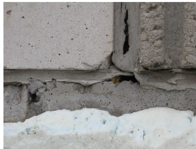
AR-028 – Open wall joints at 'east-end' addition - now an active wasp nest.
