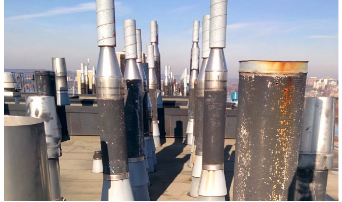
Figure 3.4 – Existing Exhaust Vents on A&L Building Penthouse Roof
