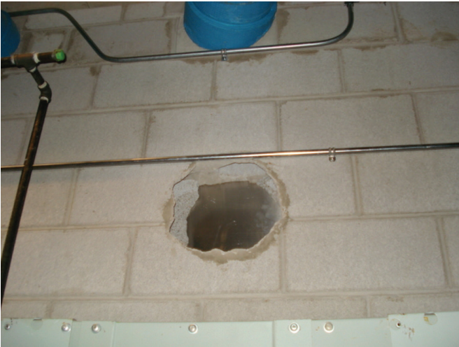
Typical Unprotected Penetration in Laboratory Rear Wall (to Service Space)
