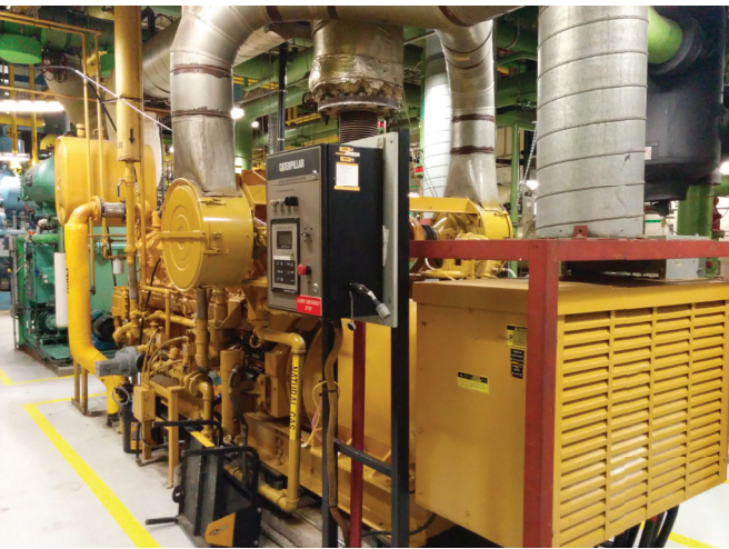
810 kW 600V Co-Generator Unit
