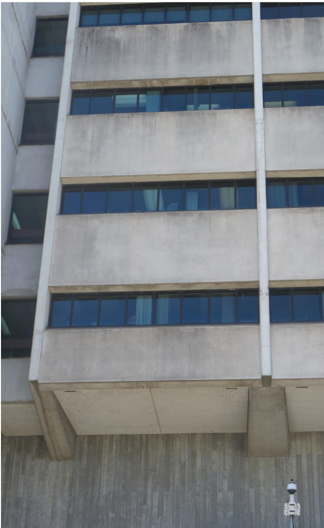
Exterior View of A&L Building Showing Floor 4-7 Cantilever
