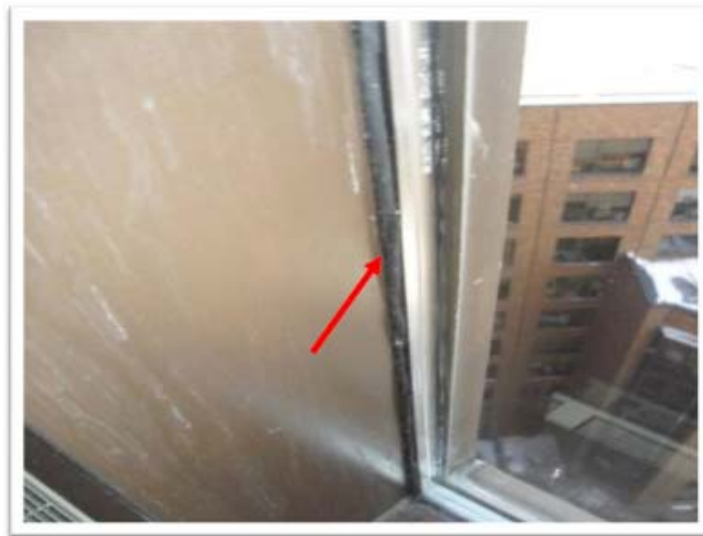
Fig. 11 – The window caulking throughout the complex is known to contain asbestos.
