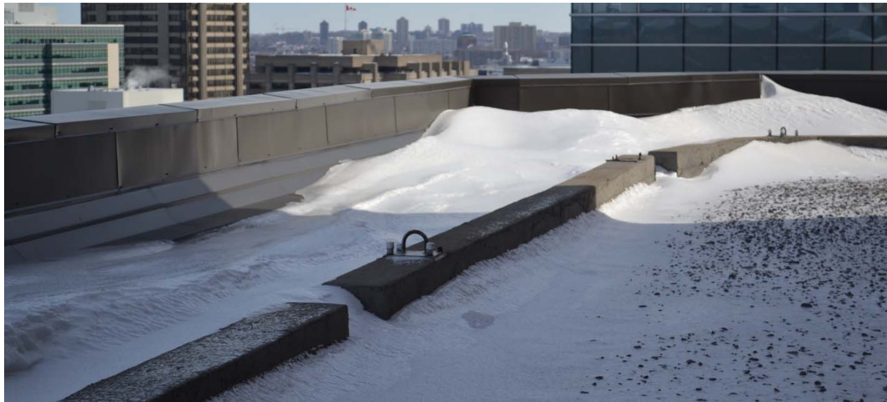
Fig. 41 – The existing parapet of 25 Eddy with perimeter track and positioning anchors. The existing anchors are not suitable for life-line attachment.
