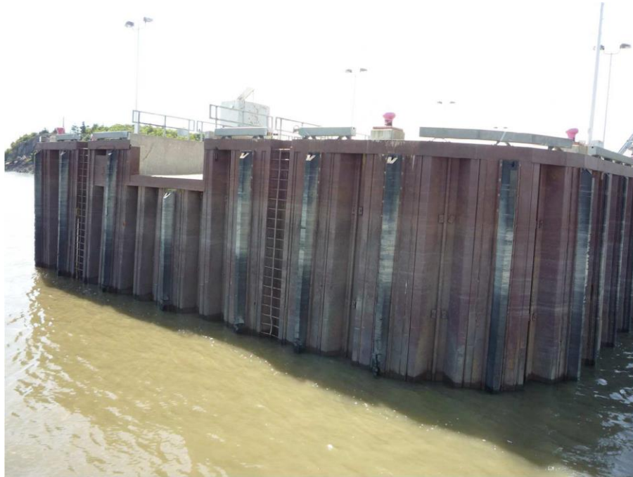
Wharf and access ramp at Grosse-Île (low and high tide)
