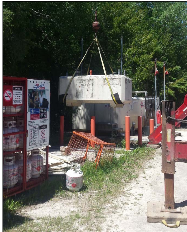
Figure 2: Removal of the 1,200 L convault diesel storage tank.
