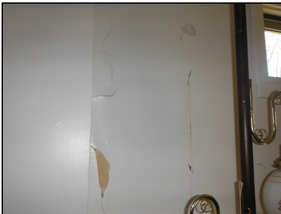
Photograph 11: Lead-Containing White Paint on Drywall – Interior, Lot 20 – Residence
