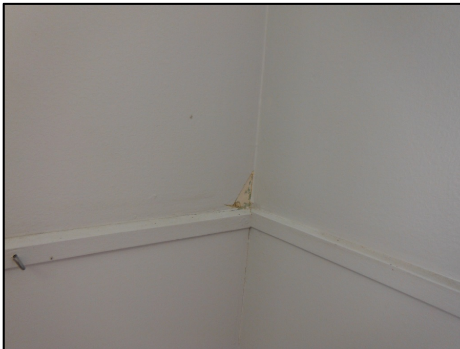
Photograph 2: Asbestos-Containing Drywall Joint Compound, Lot 20
