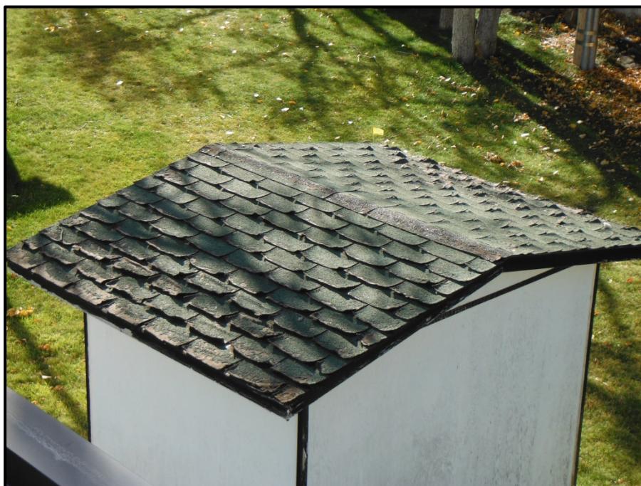
Photograph 5: Asbestos-Containing Asphalt Roofing Shingles, Shed, Lot 20 – Exterior of Residence
