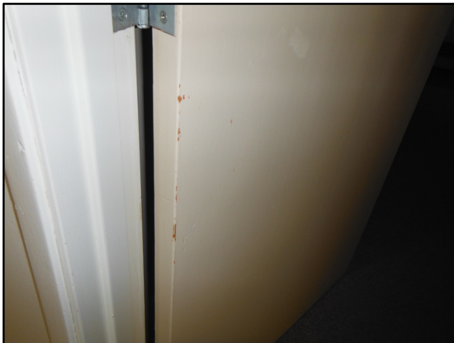
Photograph 6: Lead-Containing Beige Paint on Wood Doors/Cabinets – Interior, Bunkhouse
