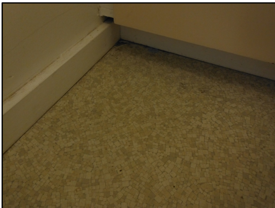
Photograph 3: Asbestos-Containing Beige Mosaic Sheet Floor, Unit 16
