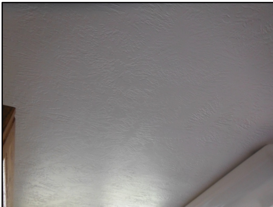
Photograph 6: Asbestos-Containing Ceiling Texture Coat (Mud), Lot 21
