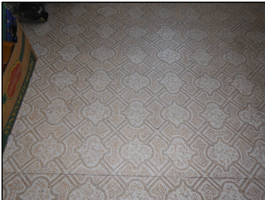
Photograph 3: Asbestos-Containing Beige Patterned Sheet Flooring, Lot 21
