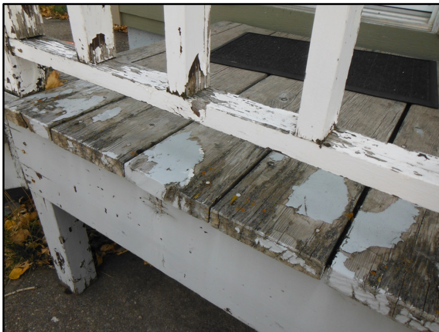
Photograph 8: Lead-Containing White and Grey Paint on Wood Deck – Interior, Lot 21
