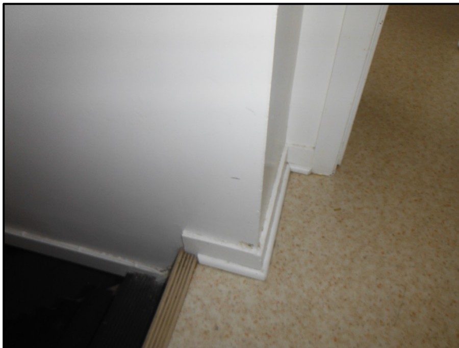
Photograph 7: Lead-Containing Beige Paint on Drywall and Wood Trim – Interior, Lot 21
