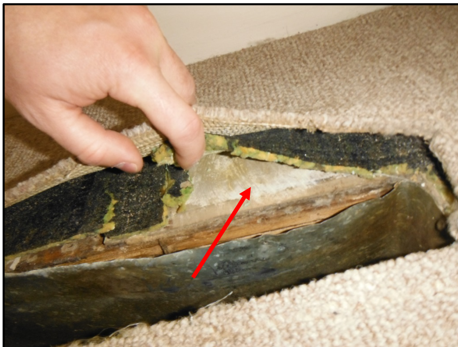
Photograph 2: Asbestos-Containing Brown Vinyl Floor Tile (Sub Floor), Lot 21
