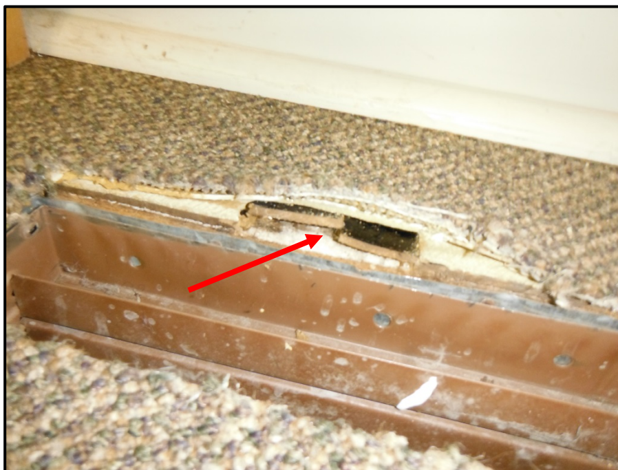
Photograph 3: Asbestos-Containing Vinyl Flooring Tile Beneath Sheet Flooring / Carpet, Lot 20 – Post Office
