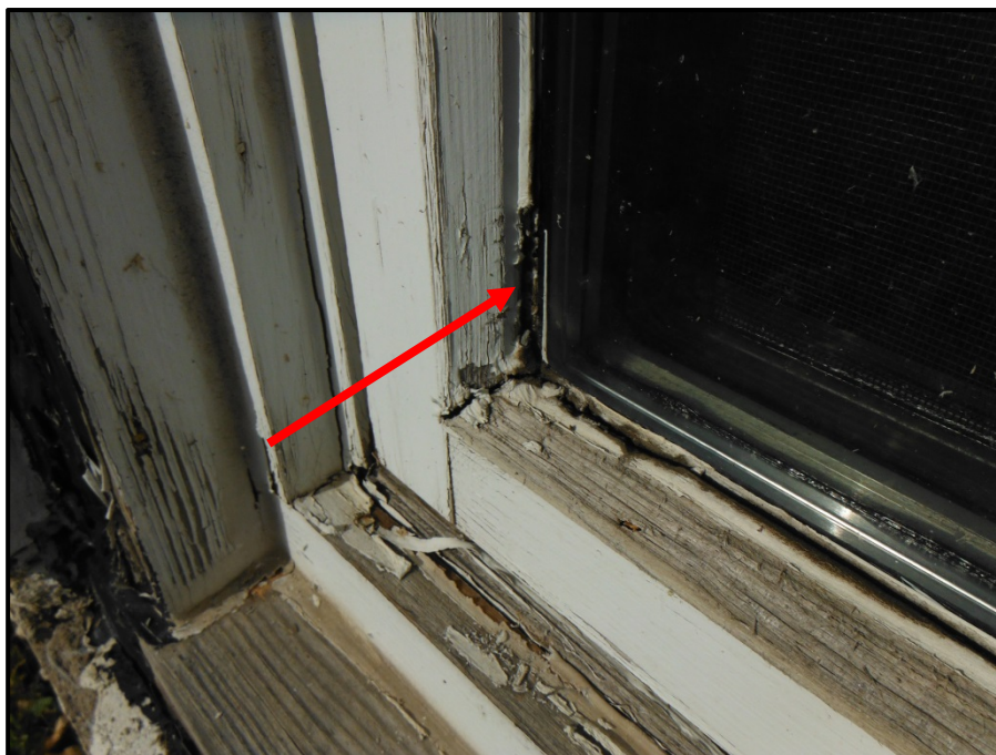
Photograph 4: Asbestos-Containing Grey Window Putty, Exterior, Lot 20 – Exterior of Residence
