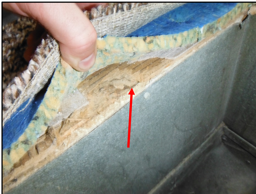
Photograph 6: Asbestos-Containing Vinyl Floor Tile Beneath Carpet, Lot 20 – Residence
