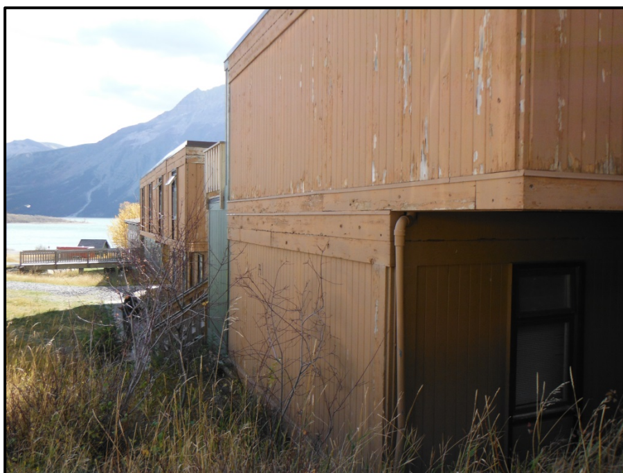
Photograph 4: Lead-Containing Brown Paint on Wood Siding/Trim – Exterior, Bunkhouse Compound
