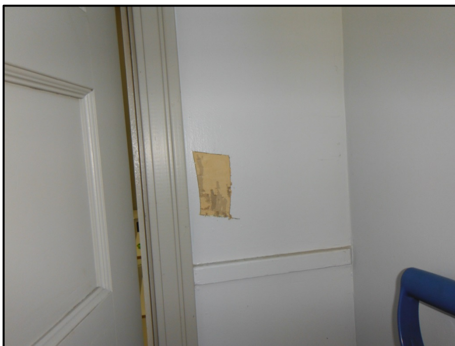
Photograph 10: Lead-Containing Light Grey Paint on Drywall – Interior, Lot 20 – Post Office
