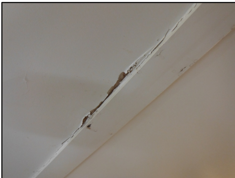
Photograph 5: Lead-Containing Off-White Paint on Drywall/Wood Trim – Interior, Bunkhouse Compound
