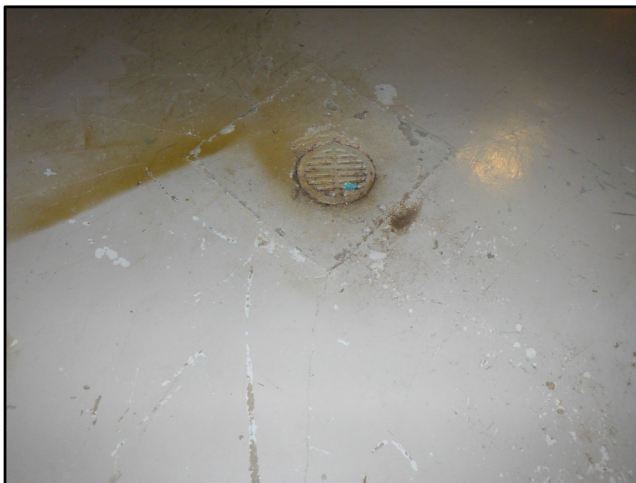
Photograph 9: Lead-Containing Grey Paint on Concrete Floor – Basement, Lot 21
