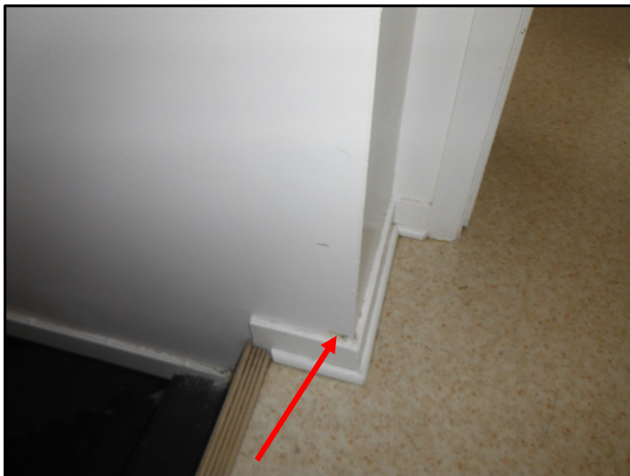
Photograph 4: Asbestos-Containing Drywall Joint Compound, Lot 21
