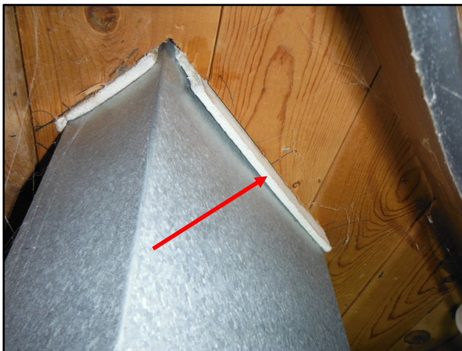
Photograph 9: Asbestos-Containing White Insulation Board around Floor Vents, Lot 20 – Residence
