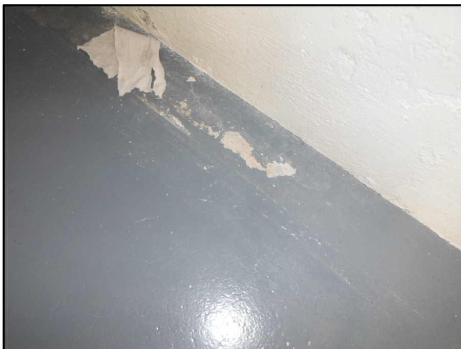
Photograph 12: Lead-Containing Grey Paint on Concrete Floor – Interior, Lot 20 – Residence
