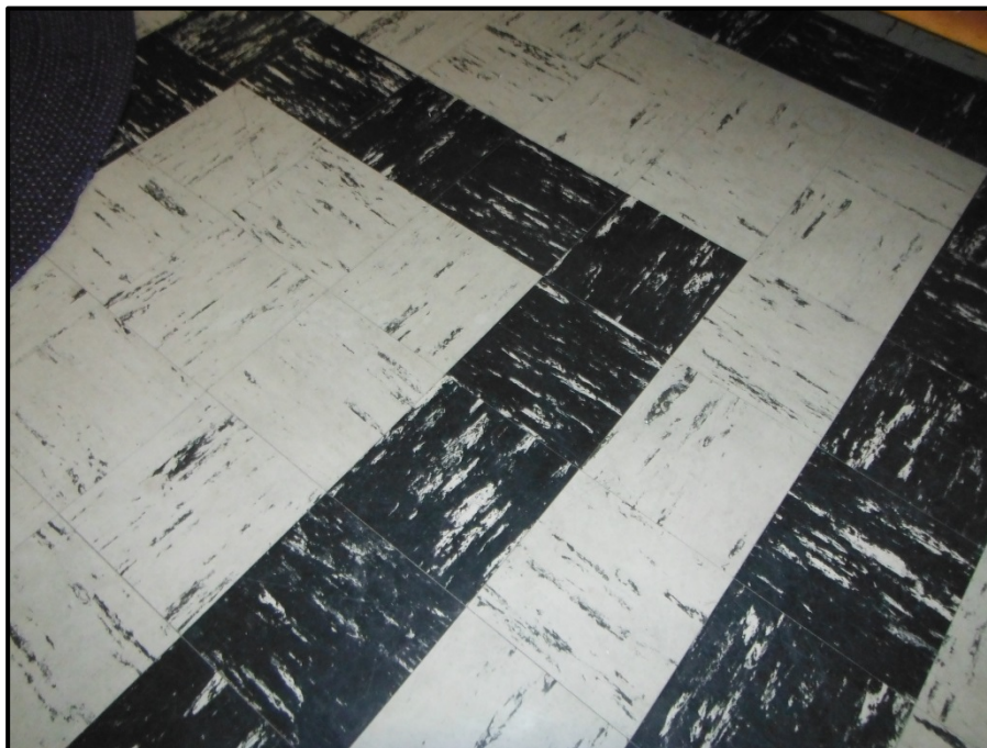
Photograph 8: Asbestos-Containing 9" x 9" Vinyl Floor Tile, Basement, Lot 20 – Residence
