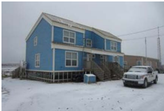
Photo 1: Outdoor above ground fuel tank
