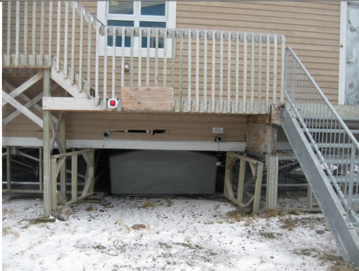
Sewer tank at detachment, between triodetic foundations
