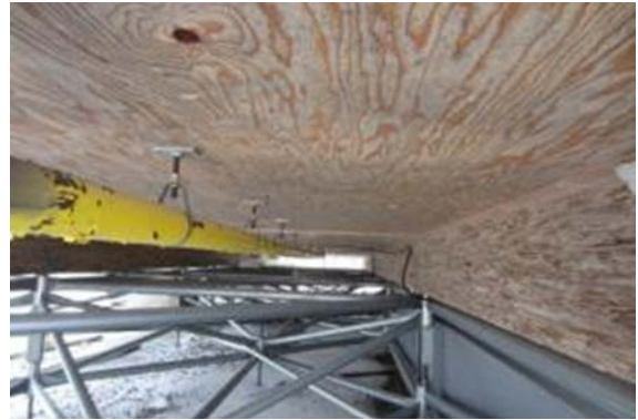
Photo 4: Exterior piping below building
