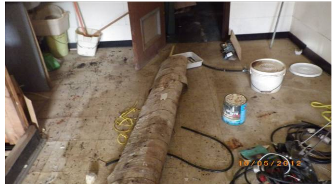
Photo 30. View of debris inside subject building including pipe lagging (Sample TK-ACM-2) and general debris.
