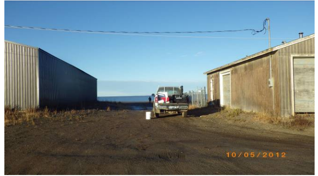
Photo 2. Looking west between on-site building and NRCAN Cold Storage Building. Includes view of Beaufort Sea to the west. Location of samples TK-TH1 to TK-TH4 along south perimeter of building.
