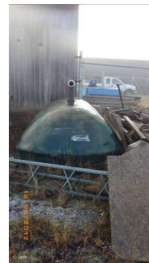
Photo 18. View of green fiberglass holding tank on south side of the subject building (Sample TK-LP-6).
