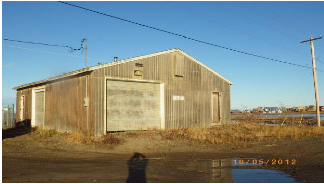
Photo 1. Looking west at on-site building including view of overhead power lines and sample locations TK-TH8 (east of garage door) and TK-TH-LP-1 (garage door).
