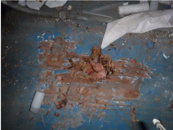
Photo 73: Insulation below blue painted wooden flooring (2016).
