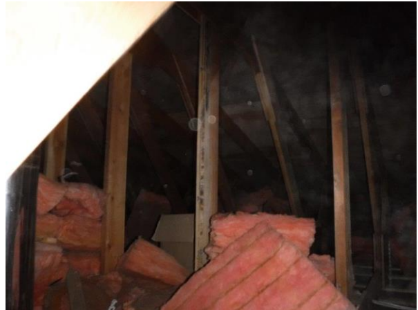
Photo 16: Insulation in attic and roofing (2016).
