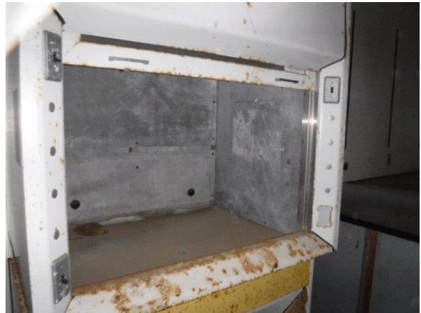
Photo 20: View of fumehood located in NE room/lab (2016). Cementitious panels within fumehood were none detected for asbestos fibres.
