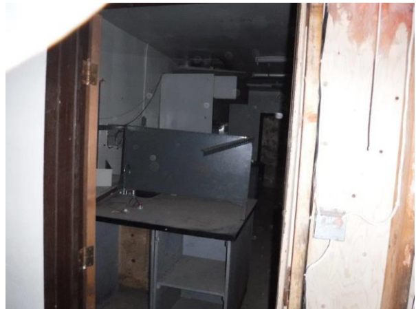
Photo 18: Equipment and desks in NE room/lab area (2016).
