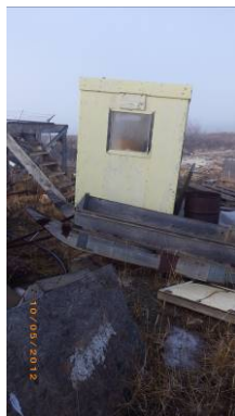
Photo 17. Close up view of skid shed located north of the on-site building. Sample location TK-LP-5.
