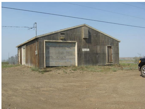
Photo 1: View of exterior Lab and Storage Building (2012).
