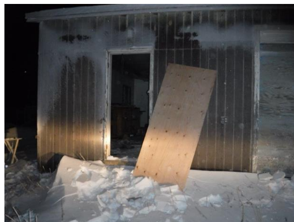
Photo 2: View of exterior entrance to building (2016).
