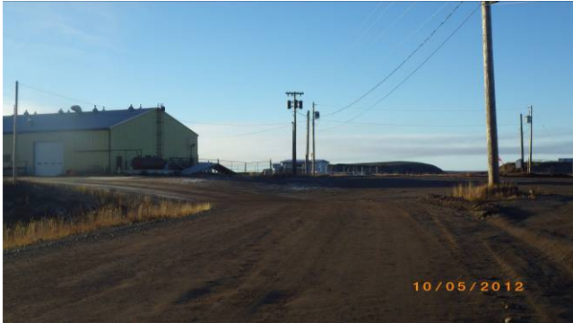
Photo 7. Looking further to the south-southeast towards Hamlet property (garage), including transformers on hydro poles and ASTs.
