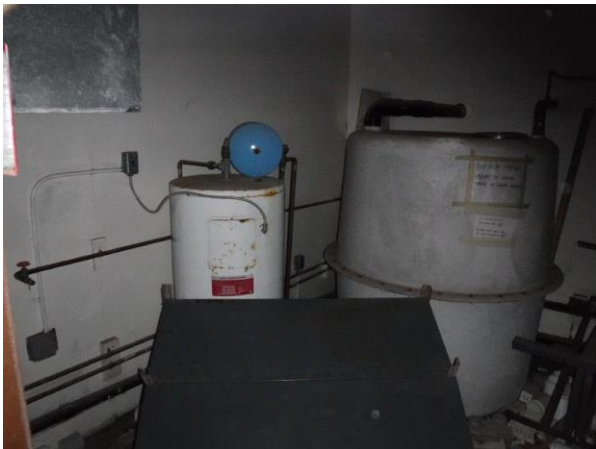
Photo 21: View of NW room/utility room.
