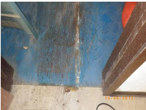
Photo 11: View of transition between vinyl floor tile section in SW room and blue painted wooden flooring in NW room/utility room (2012).
