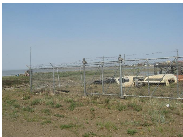
Photo 3: View of miscellaneous debris inside fence (2012).
