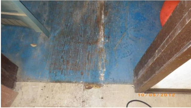
Photo 31. View of two types of flooring inside subject building. Samples TK-ACM-3 (beige vinyl flooring) and TK-LP-4 (dark blue paint on wooden flooring).
