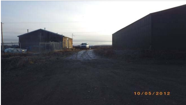
Photo 9. Looking east at the subject property and NRCAN Cold Storage Building.
