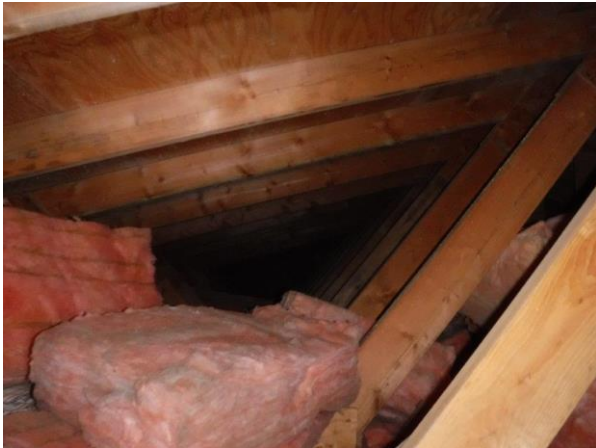
Photo 15: View of attic (2016).
