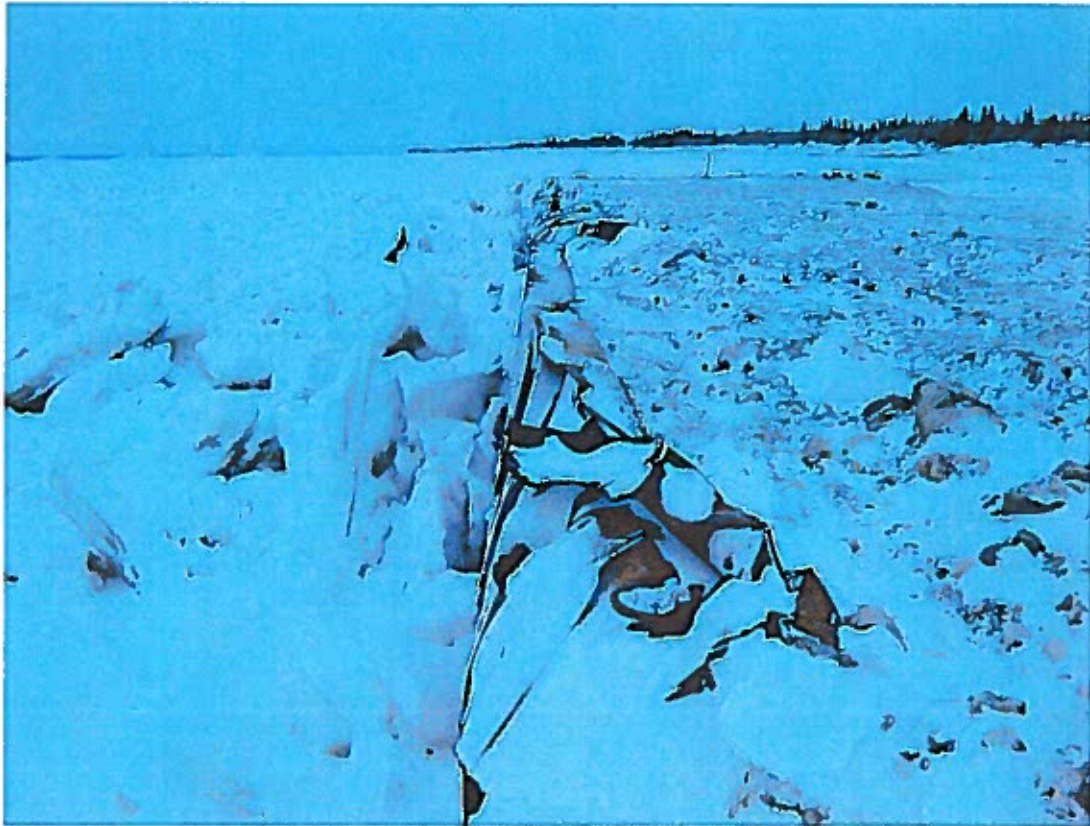
2008-12-03DFO Wharf Norman WellsP011.JPG - Looking west along riverside sheet piling, damaged areas extend down piles ~1.0m throughout.
