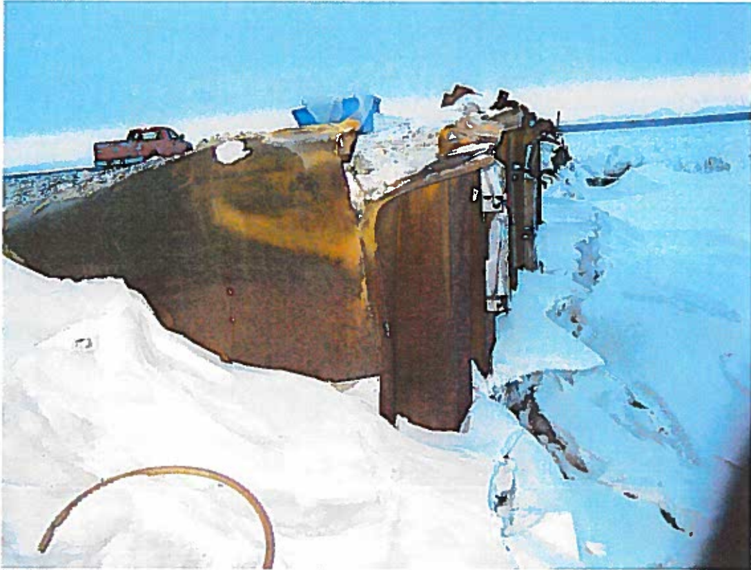
2008-12-03DFO Wharf Norman WellsP023.JPG - Looking south at downstream wharf to north of loading ramp area, buckling and distortions throughout.
