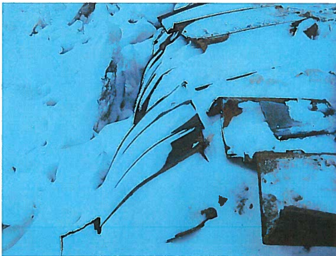
2008-12-03DFO Wharf Norman WellsP014.JPG - Typical ice damage to tops of piles, top ~1.0m distorted ~400mm, local information indicates that ~100mm of infill is added each year.
