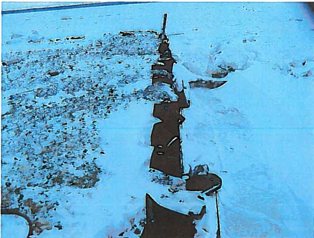
2008-12-03DFO Wharf Norman WellsP020.JPG - Looking north along downstream (west) wall, distorted ~100-200mm throughout at tops.
