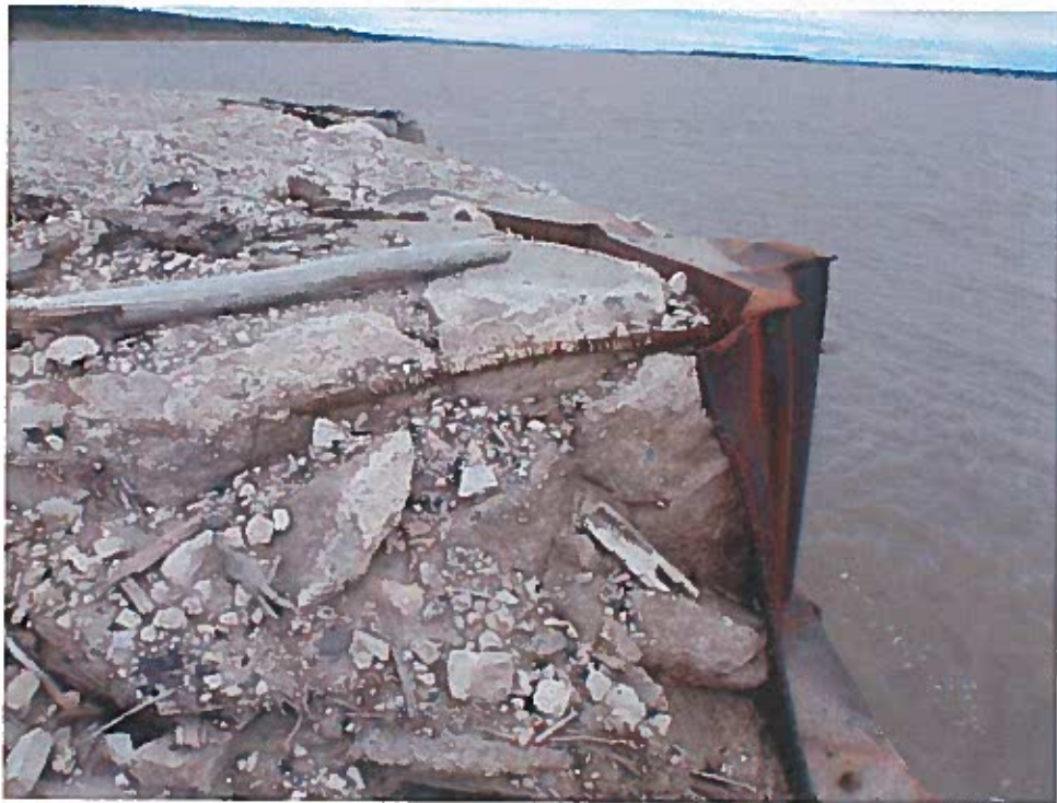
Photo 10: Concrete block/deck on southeast corner of the wharf in poor condition
