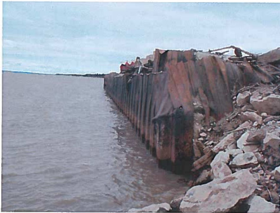
Photo 6: Extensive damage on Southeast corner of the wharf. East wall buried in debris
