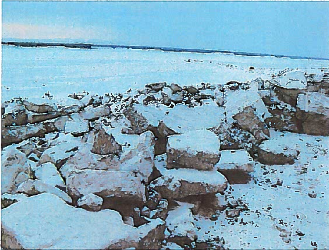
2008-12-03DFO Wharf Norman WellsP027.JPG - Water intake rock protection downstream of wharf, rock up to ~3.0x2.0mx600mm thick.
