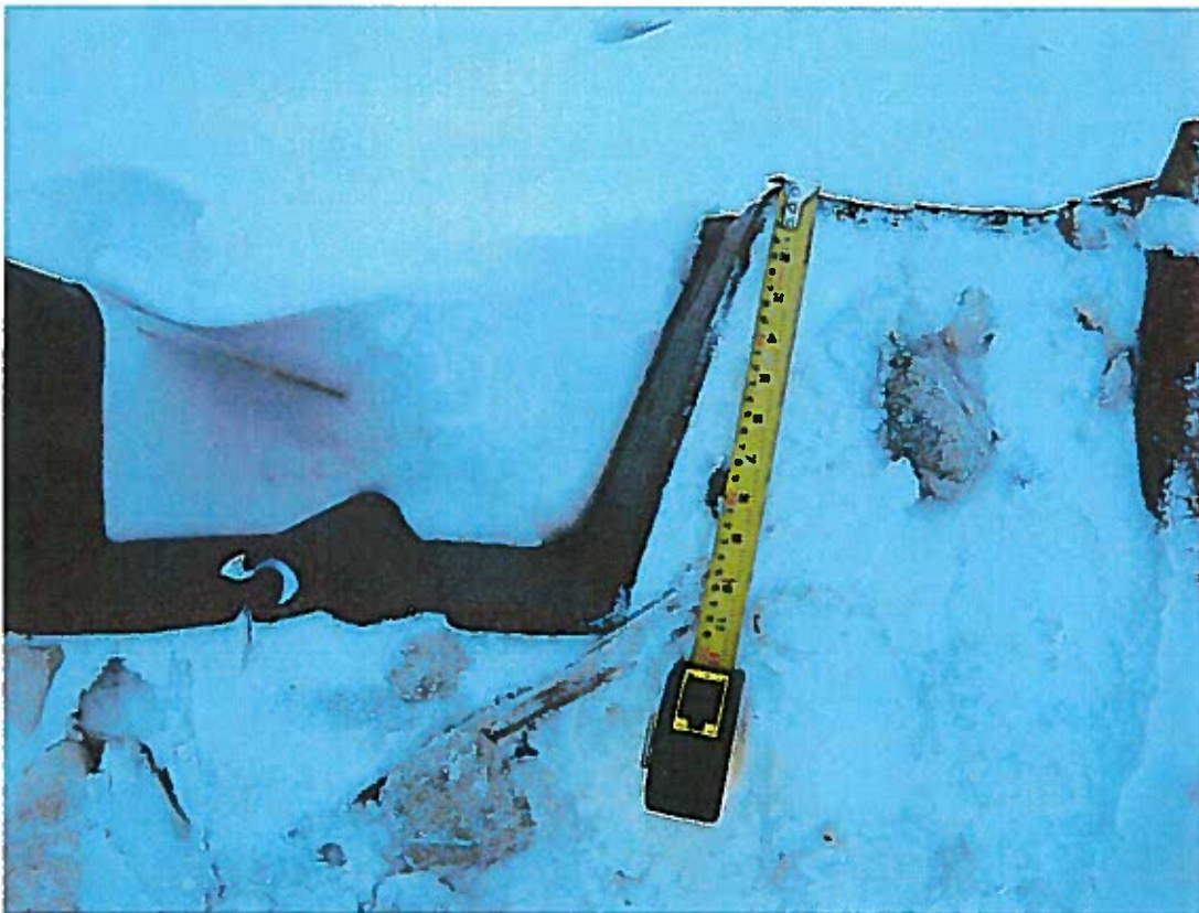
2008-12-03DFO Wharf Norman WellsP010.JPG - Sheet piles appear to be 450x300mm sections.
