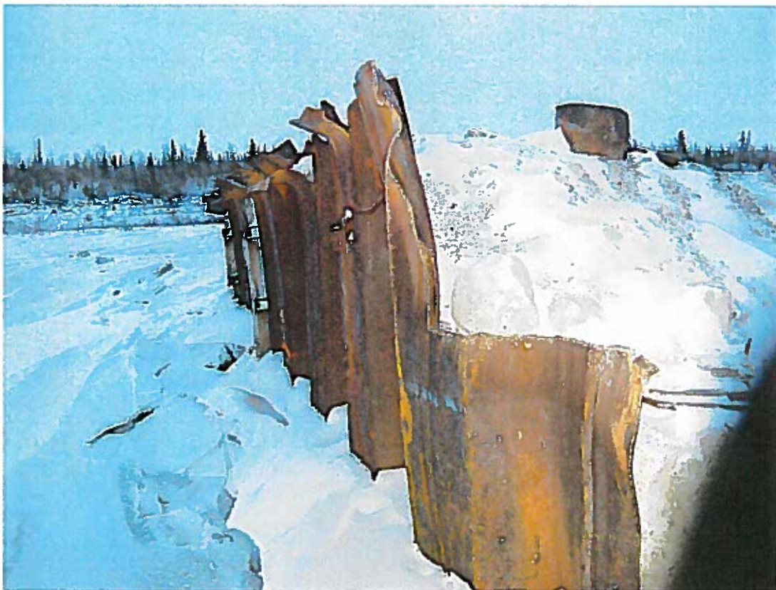
2008-12-03DFO Wharf Norman WellsP022.JPG - Looking north along downstream wharf to north side of loading ramp area, top ~1.0m of piles distorted.
