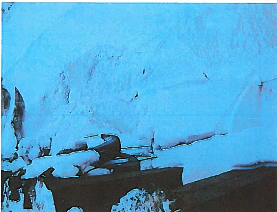
2008-12-03DFO Wharf Norman WellsP016.JPG - ~2.6m freeboard from top of piles to ice at west (downstream) end of wharf.
