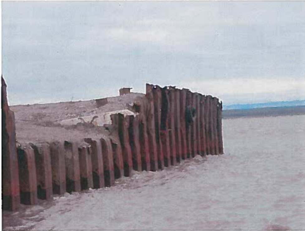
Photo3: Sheet pile cut out for ramp access
