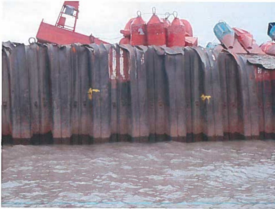
Photo 5: South face of the wharf. Note bent sheet piles at the top
