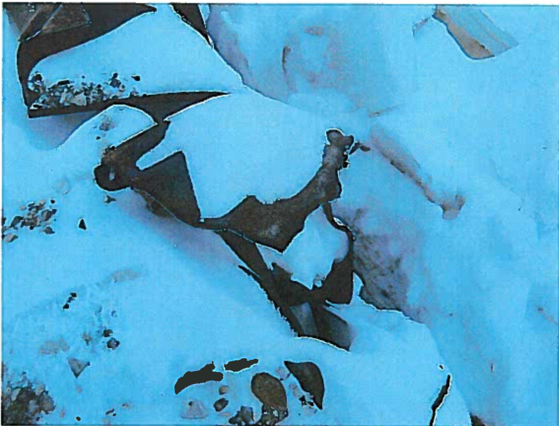
2008-12-03DFO Wharf Norman WellsP018.JPG - One of 3 locations with bad separations or tears in south riverside wall, ~1.0m deep and separated/torn ~300mm.
