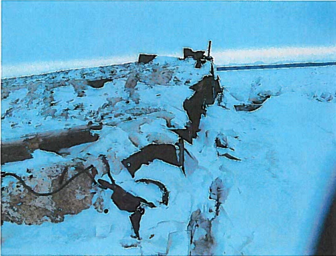
2008-12-03DFO Wharf Norman WellsP021.JPG - Looking south along downstream (west) wall, distortion and buckling for top ~1.0m of piles, also note deterioration of concrete with exposed corroded rebar.
