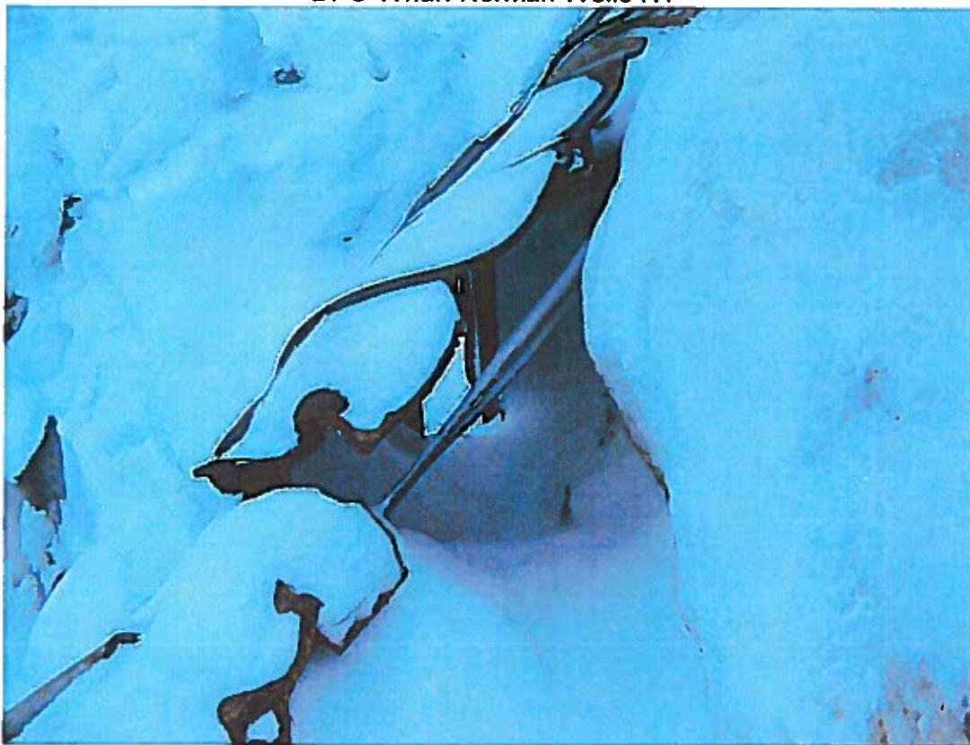
2008-12-03DFO Wharf Norman WellsP015.JPG - Separations between and tears to piles up to ~300mm wide losing fill at 3 locations, also note exposed tie back cables ~100mm below fill at this location.
