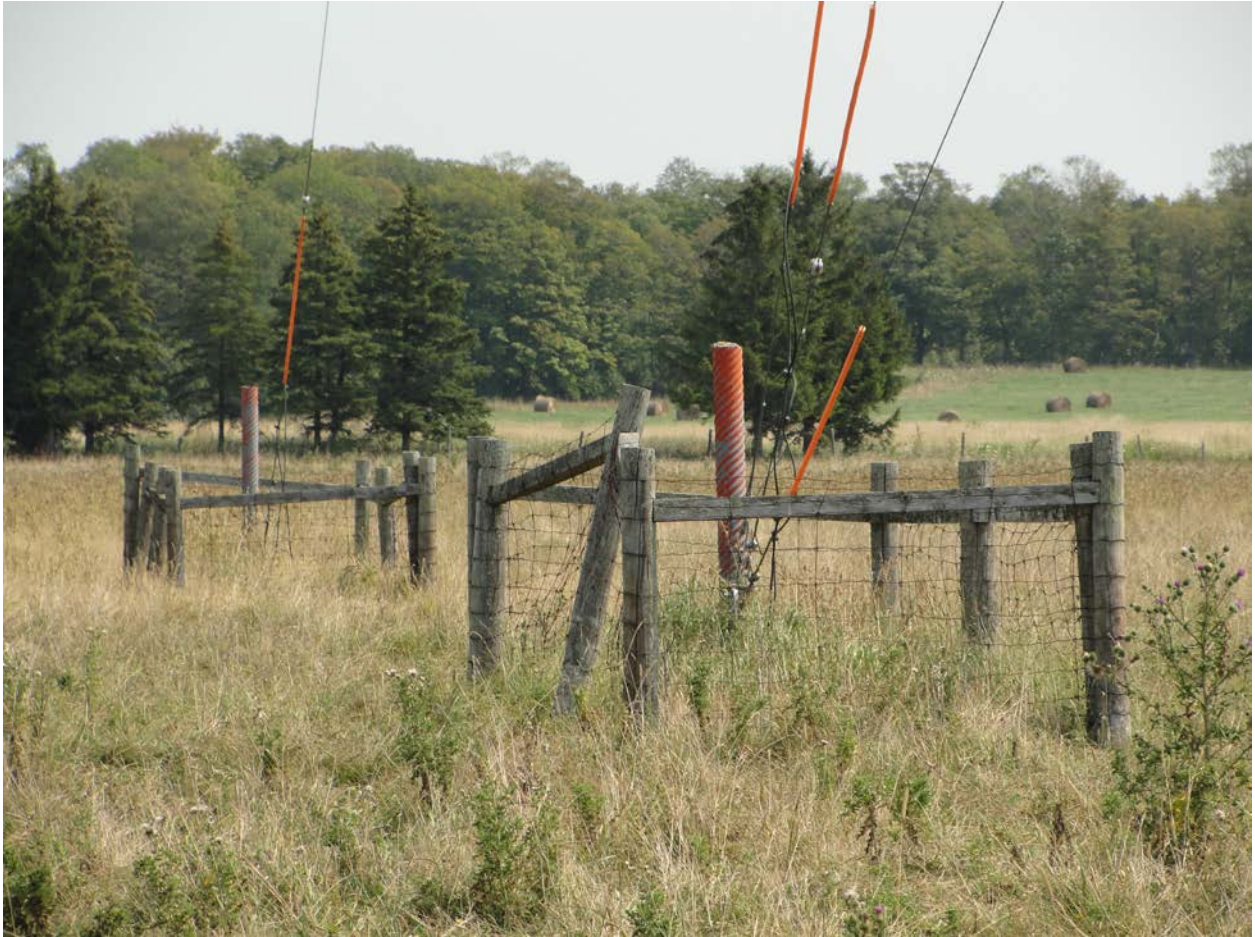
Figure 2: Typical fencing compounds to be replaced
