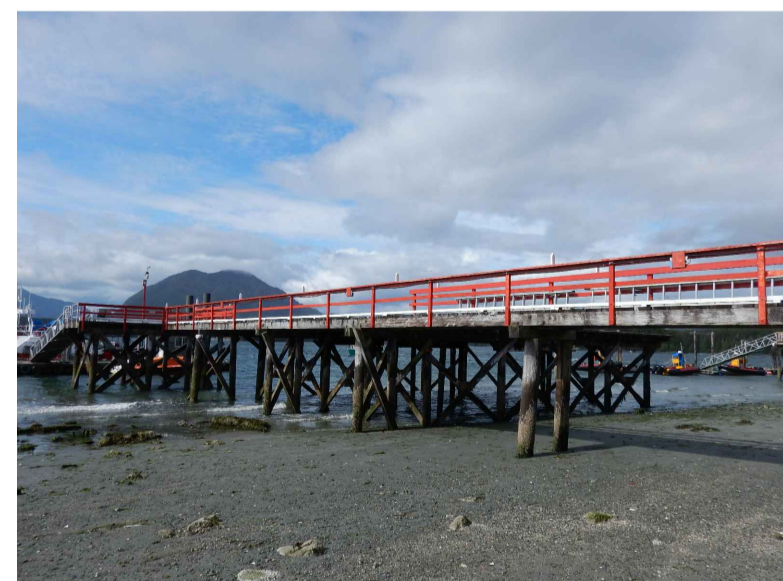
A. West side of the Approach
