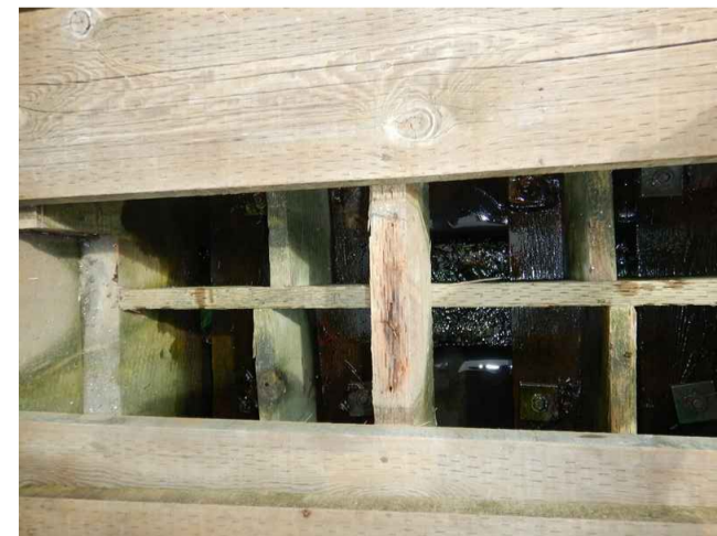
C. Cross section showing upper cross tie and internal blocking timbers
