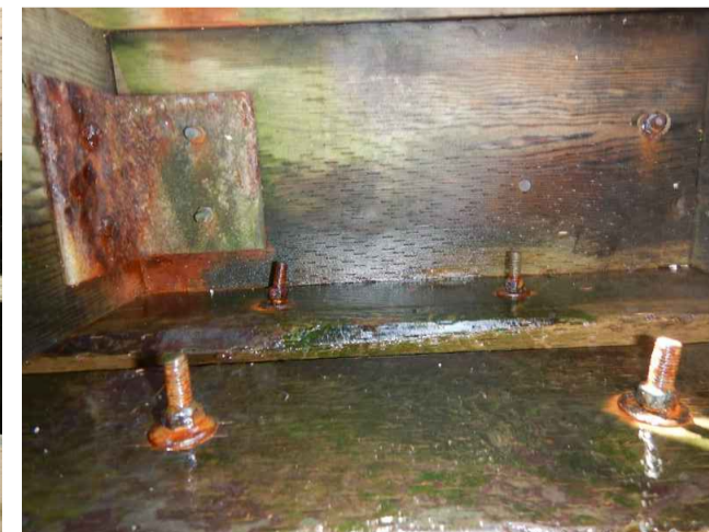
D. Lower cross ties and flotation attachment hardware
